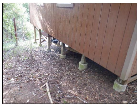
Photo 4. The post and pier foundation of the pre-existing drying and curing buildings.
