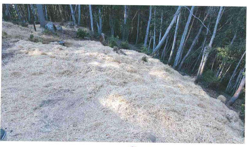
this photograph shows aver (1) after stumps and debri were removed from edge of fill. 22 bales of hay were spread. Clover seed was also spread.
