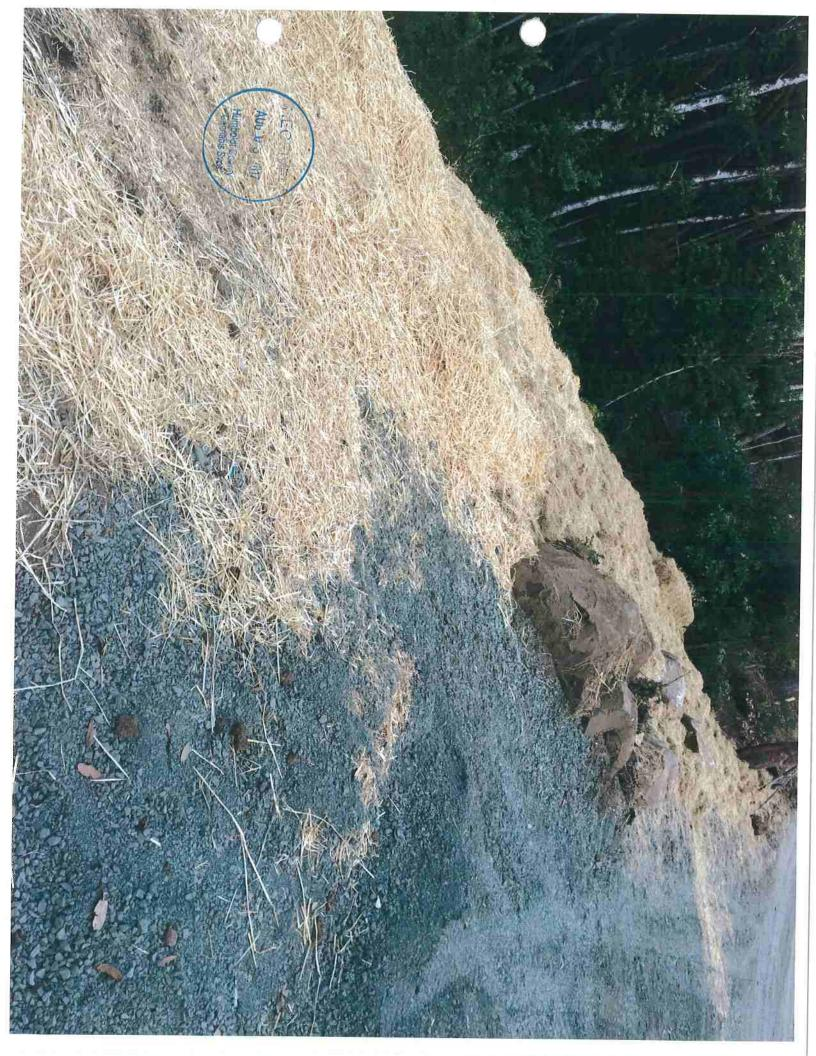
this photo of AP NO 221.211.025 was taken August 3.2017 this photograph shows Mitigation efforts. Stumps and debut are coverage gone and entire disturbed area is hayed by deep over 95% coverage granded area is revocked. Grass and clover seed is sprend this is Mitigation priority # (1) on Resource Protection Plan.
