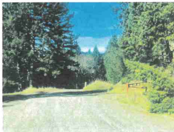
Figure RP 3. Photograph showing the access of Road 3 from the viewpoint of Road 2. This section is approximately 22 ft. wide, is paved, has a slope of around 2% and has a good pullout and visibility to the turn that leads to access to Road 3. Roadway 2 provides access to approximately 15 parcels and has an ADT of less than 400.
