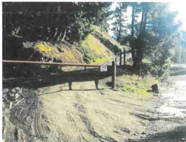
Figure RP 4. Photograph showing the start of Access Road 3 (Private Access) where it intersects with Road 2 (Old Highway 299). The access to Road 3 has good visibility, is dirt and is approximately 12-14 ft. wide with slopes of 5-10%.
