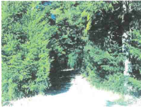
Figure RP 10. Photograph showing brush encroaching into the road that needs to be removed to provide clearance for larger vehicles reduce fire hazard and provide better visibility.
