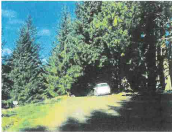
Figure RP 8. Photograph showing Road 3 at the residence for Project 1. The road north of the existing residence needs to be brushed to provide clearance for larger vehicles reduce fire hazard.
