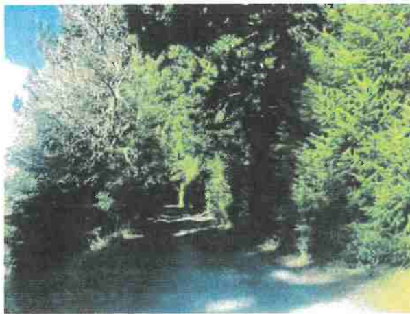
Figure RP 11. Photograph showing brush encroaching into the road that needs to be removed to provide clearance for larger vehicles, to reduce fire hazard and provide better visibility.
