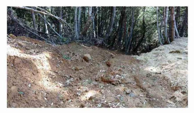
Figure 11. Site number 11, road drainage needed; rolling dip location the bank on the left side of the photo will need a dich excavated through it.
