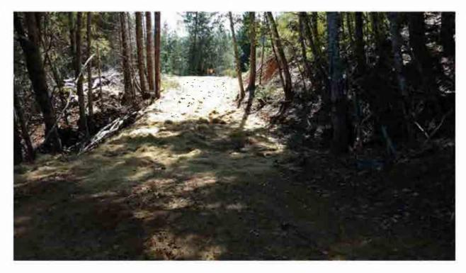
Figure 18. Site number 17, road drainage needed, rolling dip location
