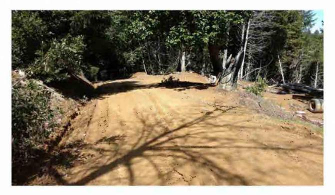
Figure 29. Site number 29, road drainage needed, rolling dip location
