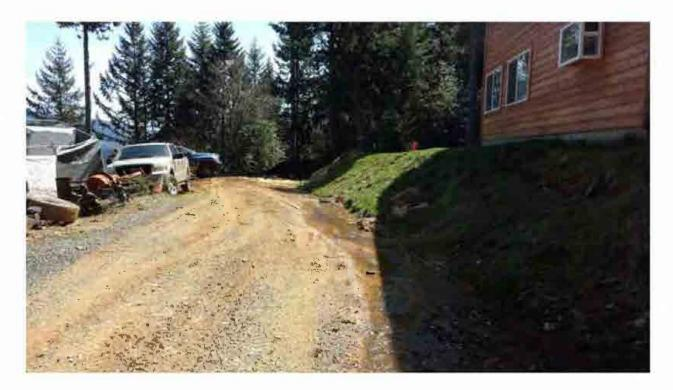
Figure 25. Site numbers 23 & 24, a French drain will be installed in the inside ditch to accommodate drainage from the Class III watercourse. Photo was taken looking downstream toward Site number 22; The Soil pile at Site number 24 is visible in the far middle of the photo.
