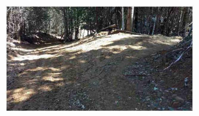
Figure 17. Site number 16, road drainage needed, rolling dip location
