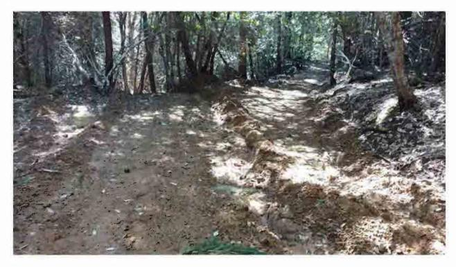
Figure 10. Site number 9, road drainage needed, rolling dip location
