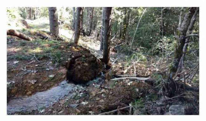
Figure 23. Site number 22, fill material eroding into the Class III watercourse at the point it leaves the inboard dich
