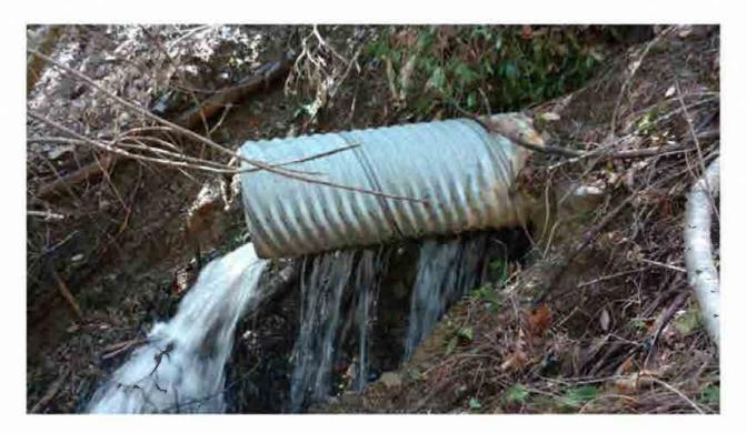
Figure 32. Site number 31, culvert outlet is above steam grade and rusted through in multiple places
