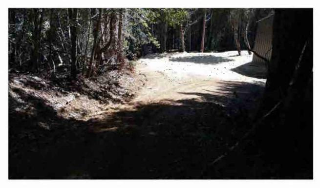
Figure 16. Site number 15, road drainage needed, Install 18" ditch relief culvert.
