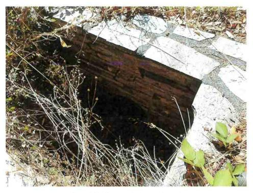
Figure 7: RP4. Outlet of 12' ditch relief culvert.
