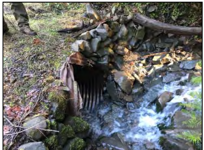
Photo #12 Fish Canyon Rd Damage 36" Culvert In
