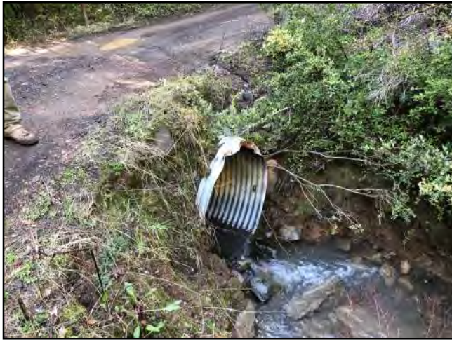
Photo #13 Fish Canyon Rd Damage 36" Culvert Out
