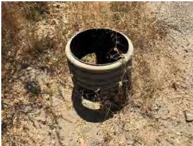
Photo #207 Red Rock Rd Looking @ 18" Culvert Inlet
