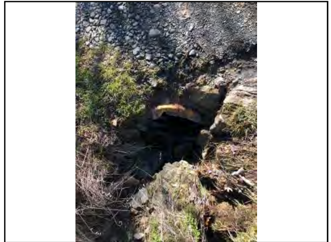
Photo #70 Road H @ Driveway Partially Clogged and Rusty 12" Culvert In
