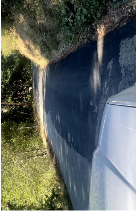
Image 7: Patching and widening undertaken about 100 feet past the location of Image 6, even with the power pole visible in Image 6 & 8 (October 19, 2022)
