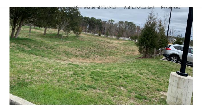
Figure 4: Stockton University's detention basin, located by the Arts and Science Building. Helps to prevent flooding from Lake Fred and runoff water from nearby parking lots. (Vincent Morano, 2020)
