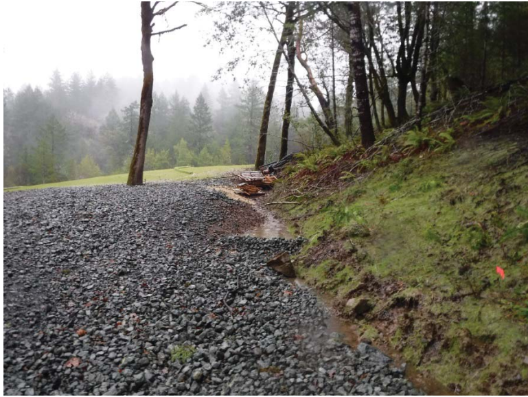
Figure 3: Rerouted reach of MP-3. A small ditch was hand-dug to keep the flow in this channel off the restored pond area (left). The right photo shows the outlet from the forest onto the rock ford, looking east. Photos taken on 11/23/18.
