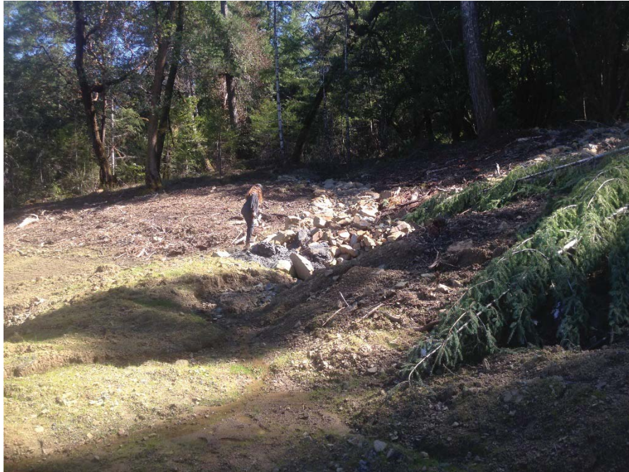
Figure 18: Cutslope above pond showing slope failure and fallen trees. Photo taken looking southeast on 4/4/18.
