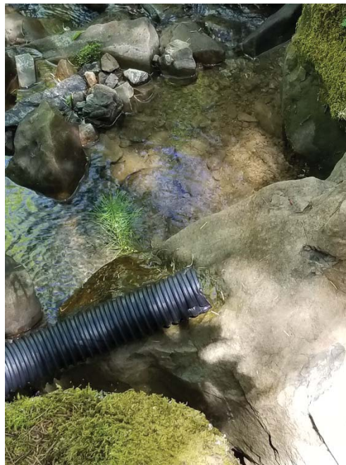
Figure 6: Outlet of cofferdam diversion (DP-3) into unnamed Class II watercourse. Photo taken looking northeast on 5/3/18.
