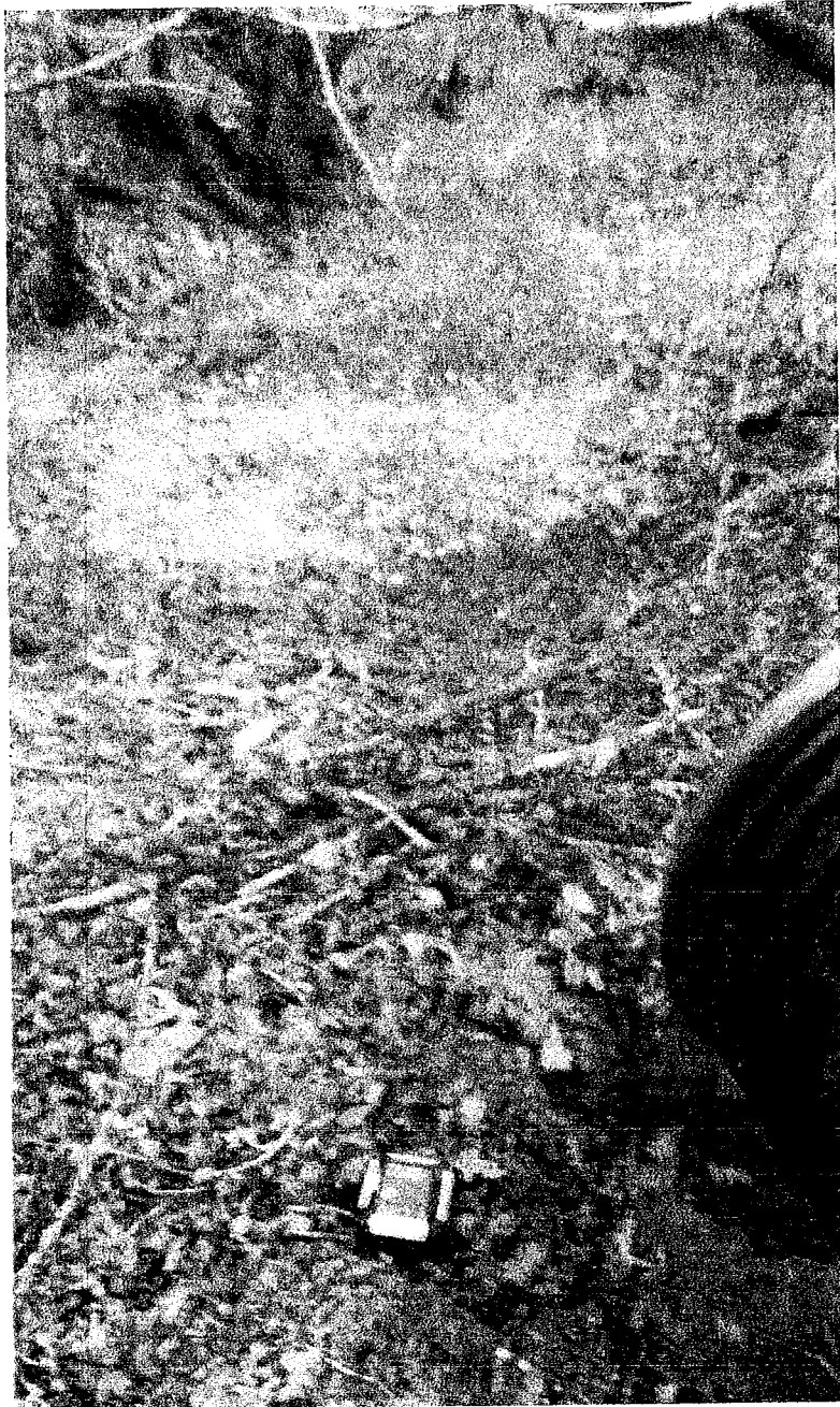
Picture 7: This is a picture of the outlet area below the culvert at Map Point 3. Rocks shall be placed below the outlet for energy dissipation and the Discharger shall monitor this area to make sure that erosion does not increase to the point of delivering to the Class III watercourse. The small topographical sediment trap located above the Class III watercourse can be seen in the distance. Photo date 12/2/2016
