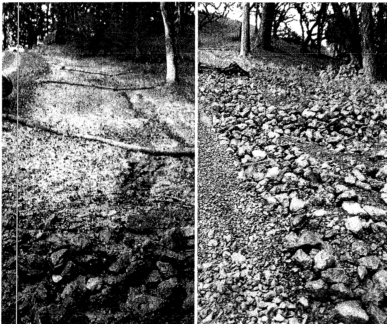
Pictures 8 and 9: These are pictures of the drainage ditch associated with Map Point 3. The picture on the left shows the wattled, seeded and mulched ditch segment above the culvert inlet. The slight rill erosion that had taken place is anticipated to lessen over time as it becomes revegetated with grass. The picture on the right is the heavily rocked segment of this ditch located below the inlet at Map Point 3. Photo date 12/2/2016
