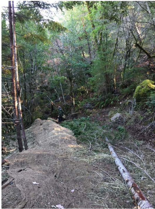
Figure 12: View of the decommissioned road south of MP-6. This is the point is the end of vehicle access from the flat with a cabin. An exaggerated water bar has been installed to make the roadway impassable for vehicles. Woody debris, jute netting and straw bale barrier have been installed to filter surface runoff and prevent erosion. Photo taken looking north on 12/6/18.
