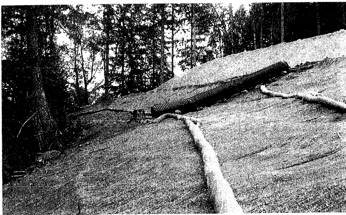
Picture 10: This a picture of the likely temporary culvert being used as an outlet to the shallow rolling dip in the road at Map Point 4. The outlet is located directly above a small conifer stump and placed rocks for dispersal. Drainage was not visible below the stump. Photo date 12/2/2016
