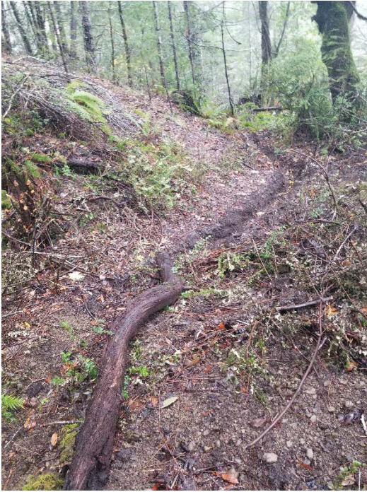
Figure 3: Rerouted reach of MP-3. A small ditch was hand-dug to keep the flow in this channel off the restored pond area (left). The right photo shows the outlet from the forest onto the rock ford, looking east. Photos taken on 11/23/18.
