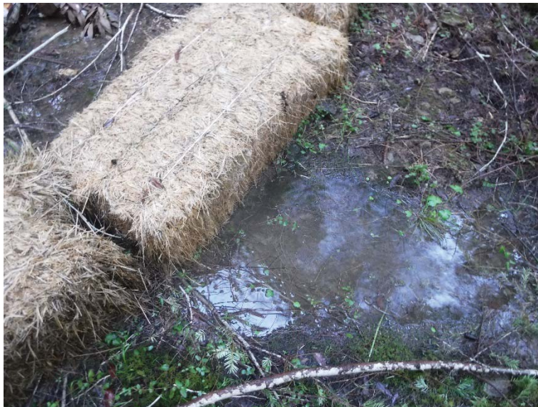
Figure 10: Outlet of rerouted reach of MP-5. Straw bales placed as a temporary checkdam/sediment trap will be replaced with an armored outfall into the unnamed Class II during summer of 2019. Photo taken 2/5/19.
