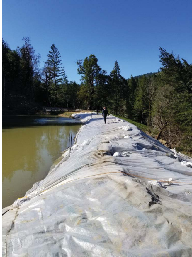
Figure 15: Pond before draining, with scarps on embankment shown in foreground. The owner tried to stabilize the embankment by covering with plastic sheeting to protect from rain. Photo taken looking northwest on 04/02/18.
