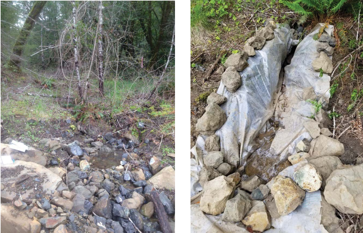
Figure 5: Before (4/25/18) and after (5/9/18) installation of the cofferdam diversion on MP-5. This temporary measure will be removed before October 2019. Photo taken looking southeast.
