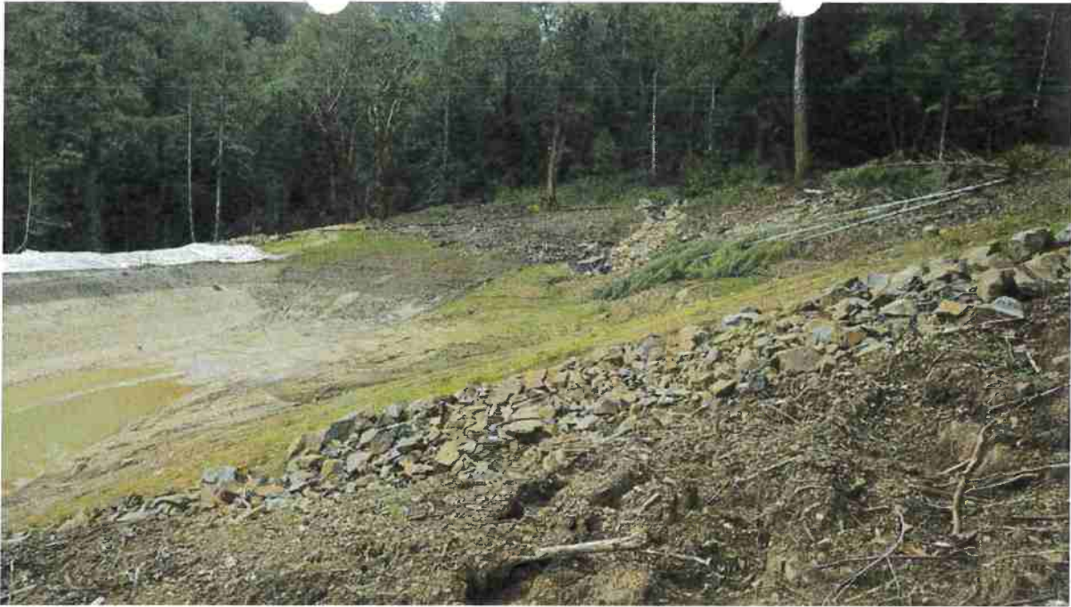
IMG0830 Large portion of cutbank failing into an illegally constructed pond in an unstable area
