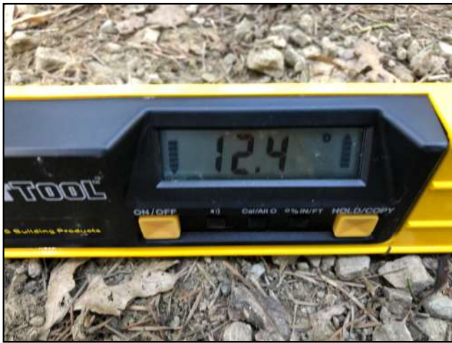
Photo #37 APN 210-074-008 Private Access Rd Slope 12.4%
