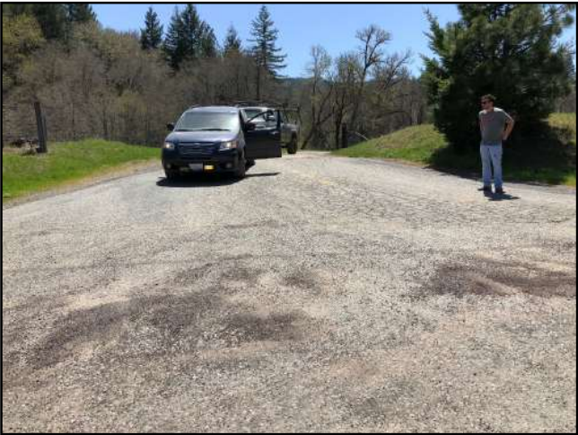
Photo #166 Hidden Valley Rd @ Hwy 36 Looking South
