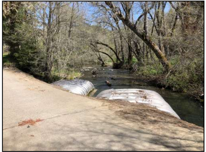
Photo #128 Hidden Valley Rd Double 120" Elliptical Culvert In
