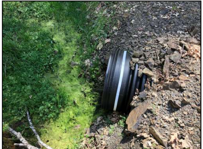
Photo #34 APN 210-074-008 Private Access Rd 18" Culvert In
