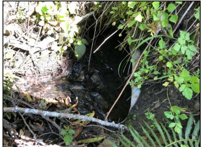
Photo #106 Hidden Valley Rd d 18" Culvert In
