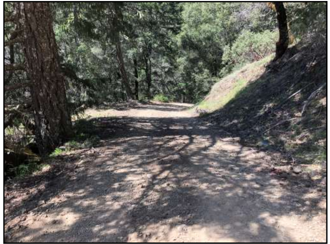
Photo #44 APN 210-074-008 Private Access Rd @ Turnout Looking SW @ Curve
