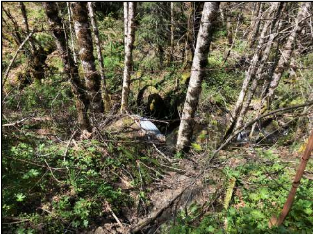
Photo #99 Hidden Valley Rd 120" Elliptical Culvert In
