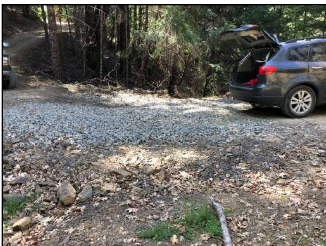
Photo #35 APN 210-074-008 Private Access Rd Looking@ Placed Rock for Drainage
