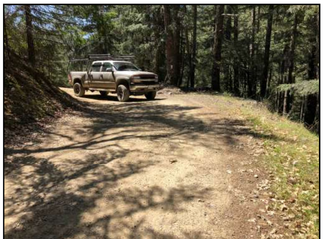
Photo #48 APN 210-074-008 Private Access Rd @ Curve w/ Turnout Looking SE
