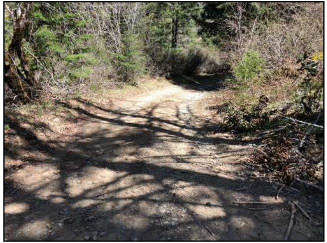
Photo #62 APN 210-074-008 Private Access Rd @ Curve w/ Turnout Looking NE
