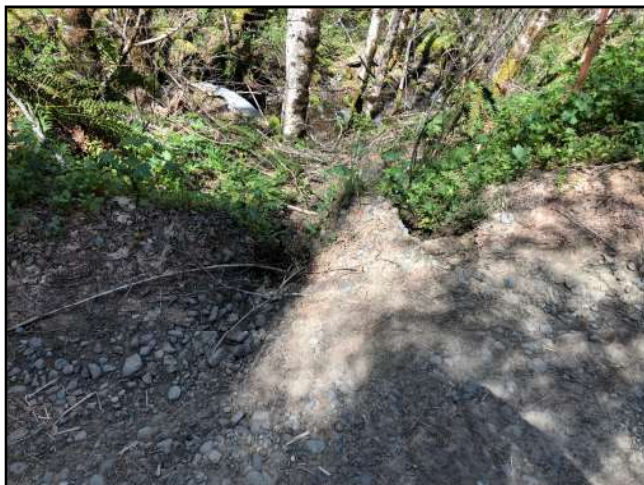
Photo #101 Hidden Valley Rd 120" Elliptical Culvert Out
