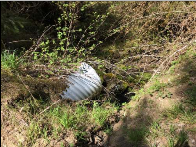
Photo #69 APN 210-074-008 Private Access Rd 18" Culvert In
