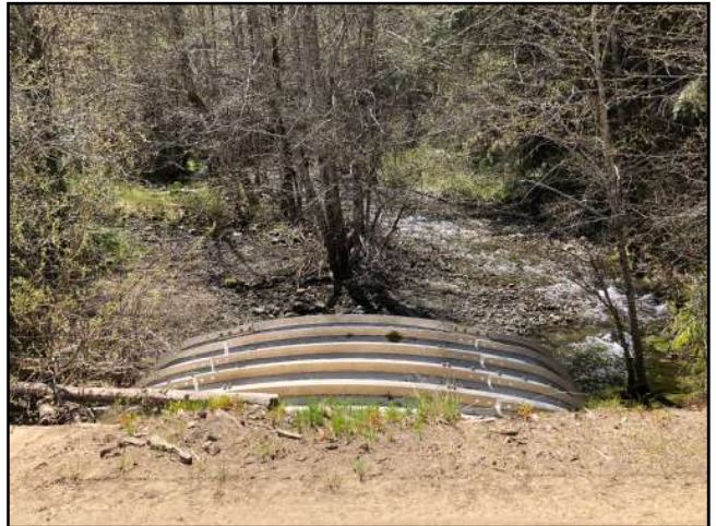
Photo #82 Hidden Valley Rd 120" Elliptical Cul- vert Out
