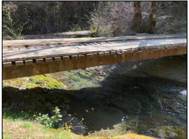
Photo #76 APN 210-074-008 Private Access Rd @ Railroad Car Bridge Looking Underneath
