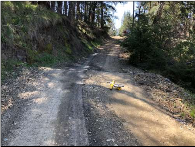
Photo #31 APN 210-074-008 Private Access Rd @ Turnout Looking SW @ Curve
