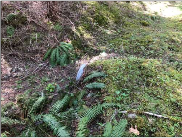
Photo #109 Hidden Valley Rd 12" Culvert In
