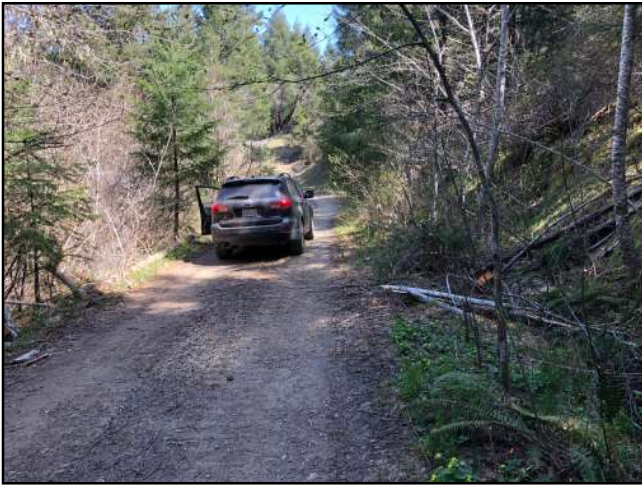
Photo #67 APN 210-074-008 Private Access Rd @ Turnout Looking NE
