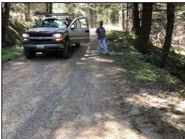
Photo #119 Hidden Valley Rd @ Turnout Looking SW
