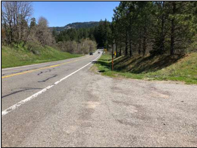
Photo #165 Hidden Valley Rd @ Hwy 36 Looking NE
