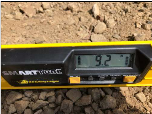
Photo #45 APN 210-074-008 Private Access Rd Slope 9.2%
