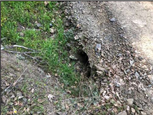
Photo #33 APN 210-074-008 Private Access Rd 18" Culvert In
