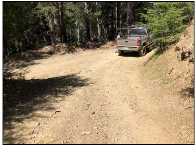
Photo #50 APN 210-074-008 Private Access Rd @ Curve w/ Turnout Looking SW @ Driveway
