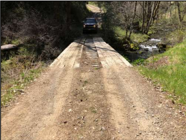
Photo #75 APN 210-074-008 Private Access Rd @ Railroad Car Bridge Looking SW
