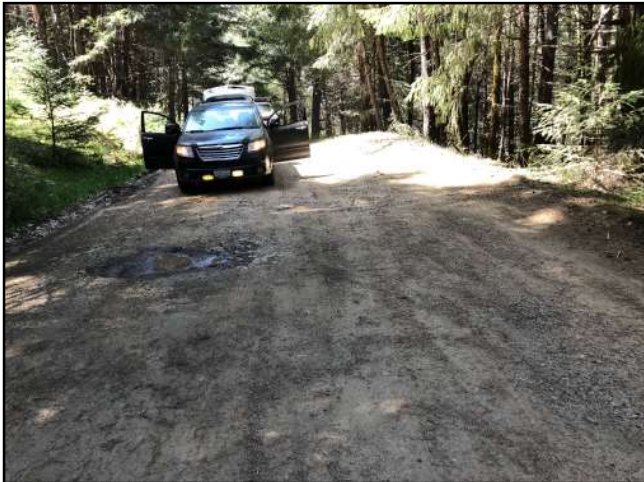
Photo #93 Hidden Valley Rd @ Turnout Looking SW
