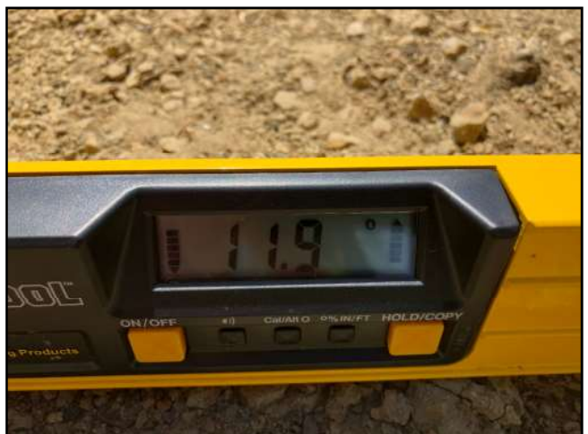
Photo #24 APN 210-074-008 Private Drive Slope 11.9%
