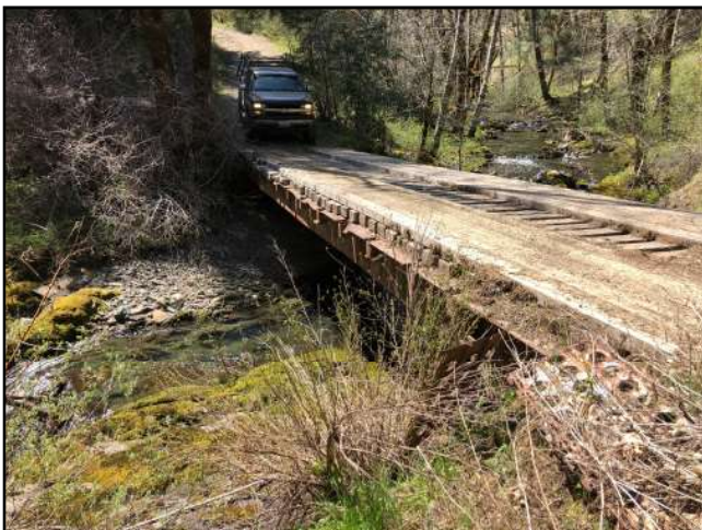
Photo #77 APN 210-074-008 Private Access Rd @ Railroad Car Bridge Looking SW
