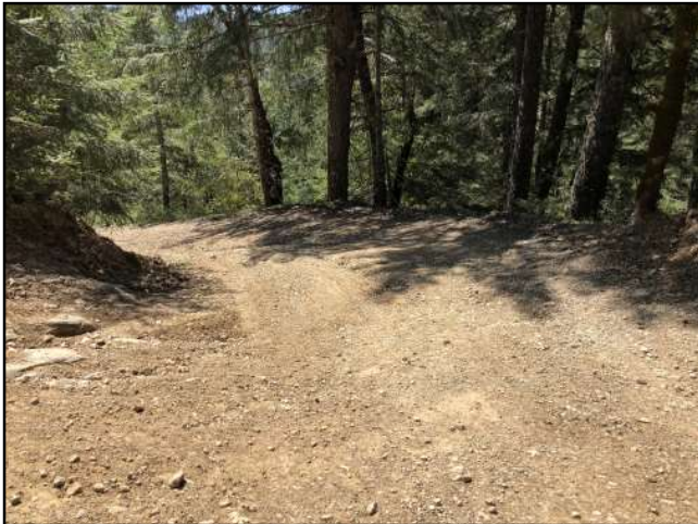
Photo #51 APN 210-074-008 Private Access Rd @ Turnout Looking SE @ Driveway
