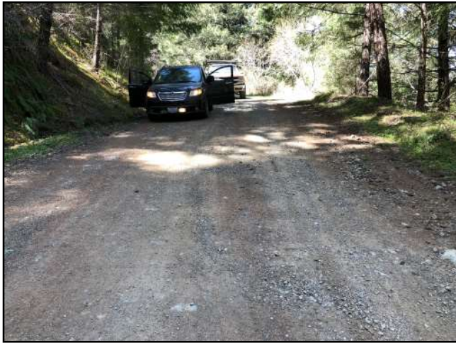
Photo #121 Hidden Valley Rd @ Curve w/ Turn-out Looking NW
