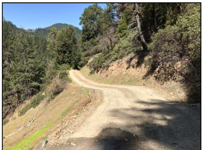
Photo #30 APN 210-074-008 Private Access Rd @ Intersection of Private Access Rd Looking NW
