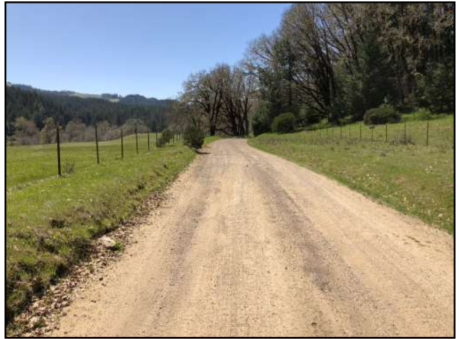
Photo #146 Hidden Valley Rd @ Turnout Looking SW
