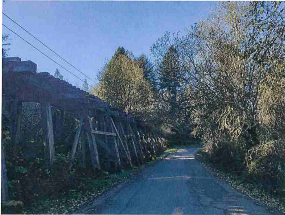
Figure 7: Paved Section around Mile 0.42
