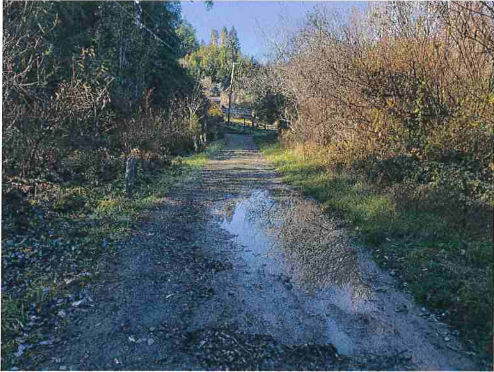
Figure 29: low section on dirt road at Mile 1.76
