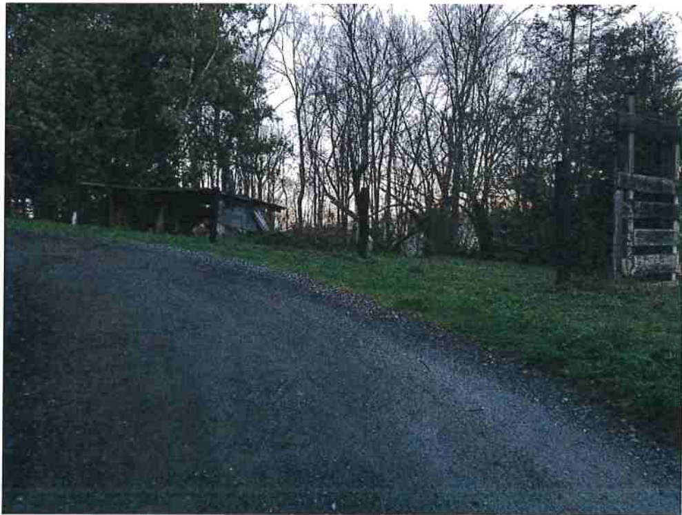
Figure 18: Turnout # 6 at Mile 1.3
