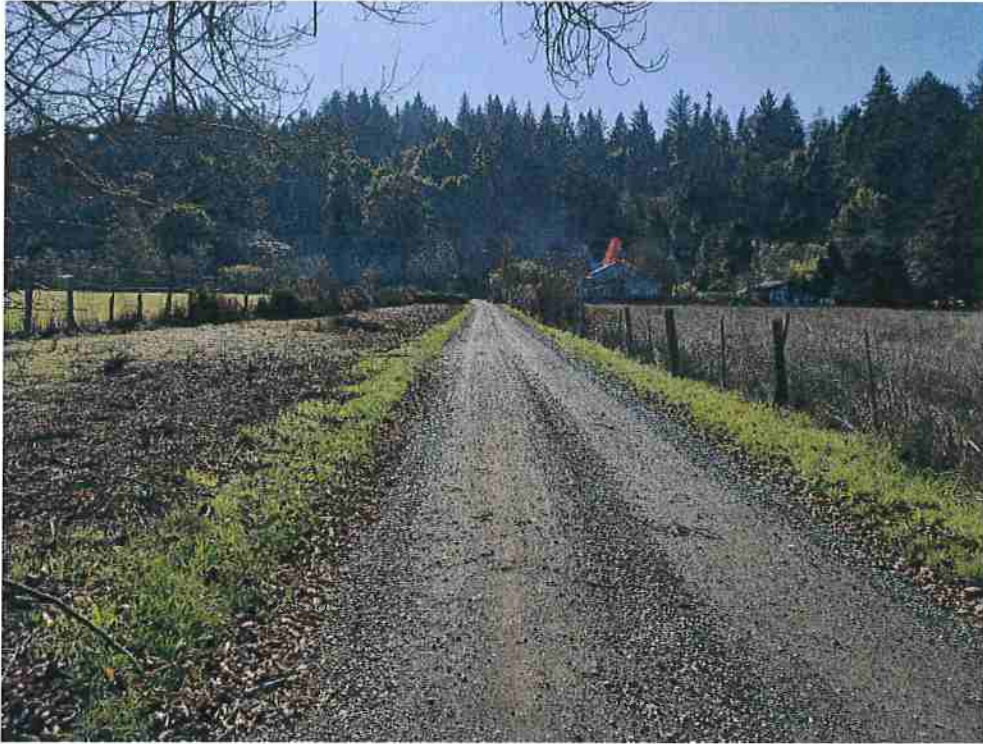
Figure 25: Gravel road at Mile 1.6
