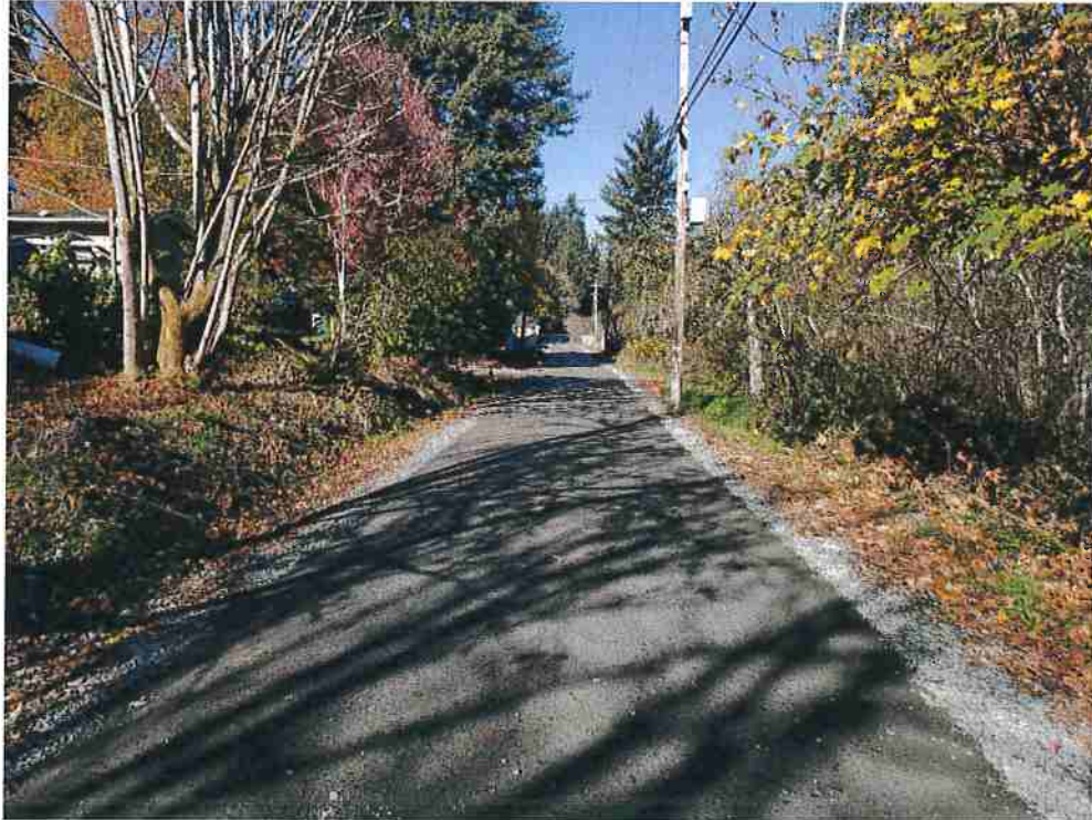
Figure 12: Gravel road surface at Mile 1.03
