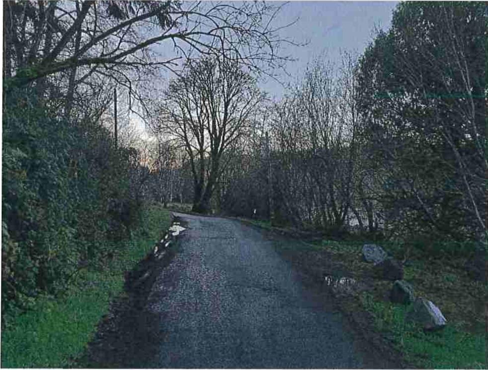
Figure 9: Turnout # 9, recommended to be levelled and rocked at PM 0.54
