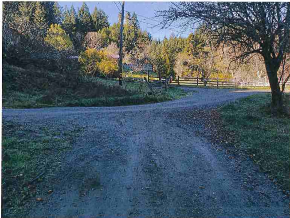
Figure 28: Road junction at Mile 1.73
