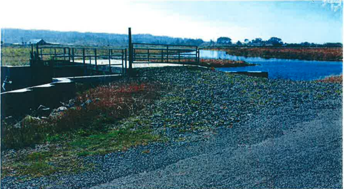
Photo: Recently constructed concrete flood gate structure with gravel entrance.
