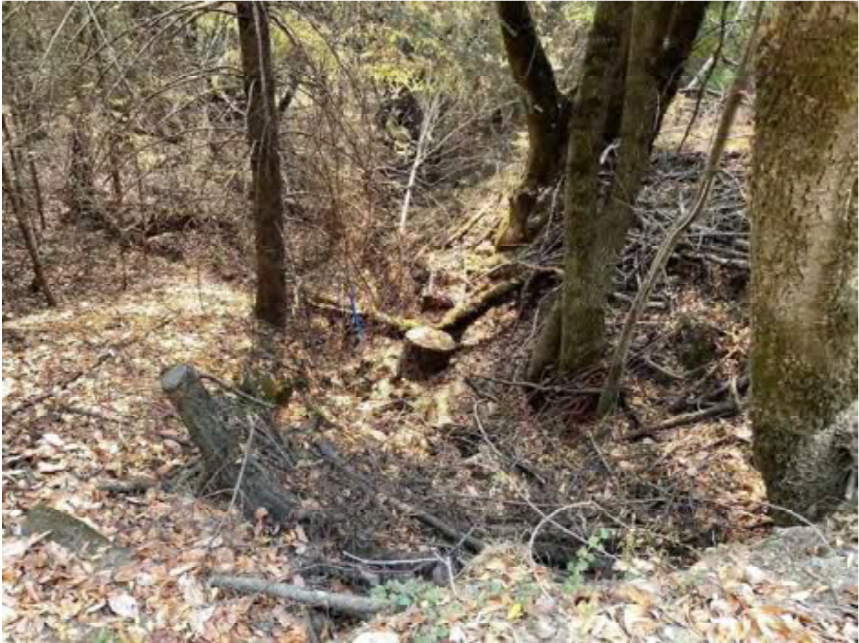
Photo 29: Stream Crossing 07. Looking downstream from the outlet of the 12-inch diameter culvert at stream crossing 07. Photo date 9-1-2021.
