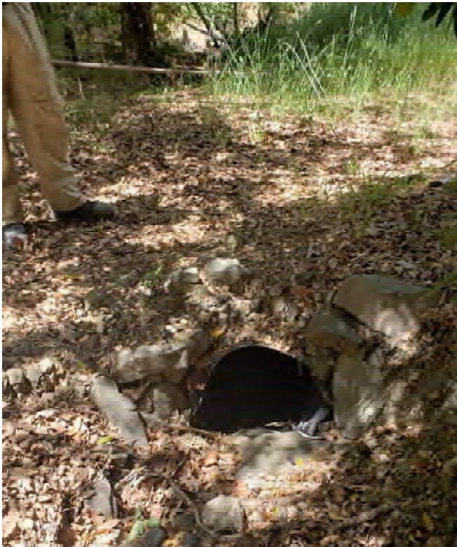
Inlet of Site 19
