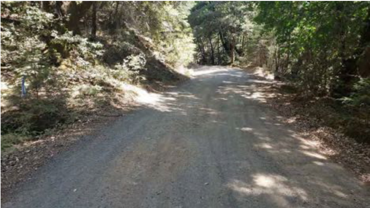
Site 24. Looking down grade.
