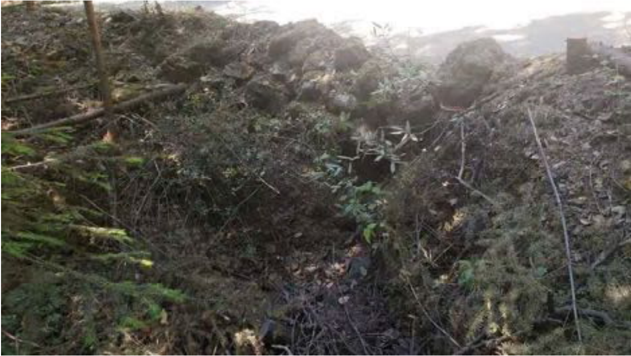
Site 26. Outlet of the watercourse crossing.
