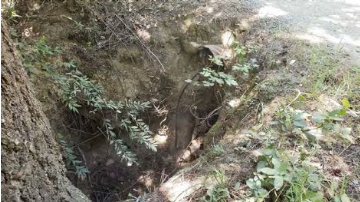
Site 14. Looking at the outlet of the ditch relief culvert.
