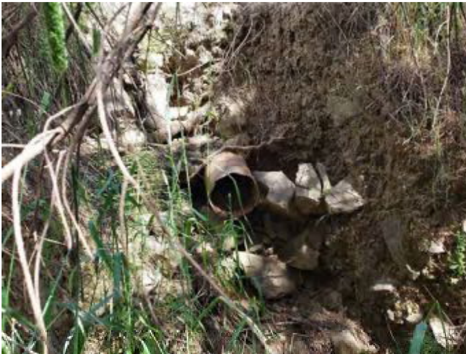
Site 07. Looking at the outlet.
