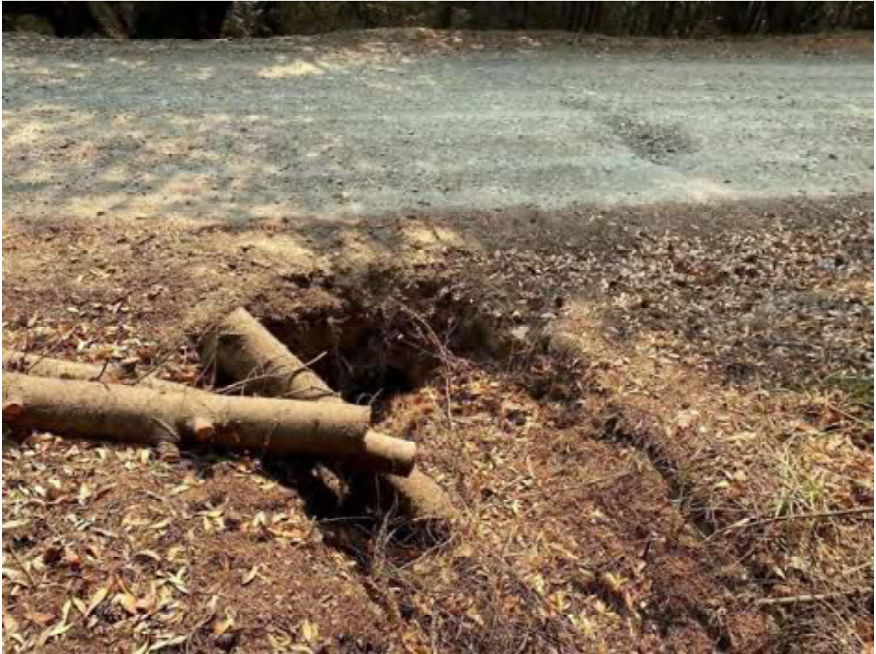
Photo 21: Stream Crossing 06. Looking downstream towards the inlet of the 12-inch diameter culvert at stream crossing 06. Photo date 9-1-2021.
