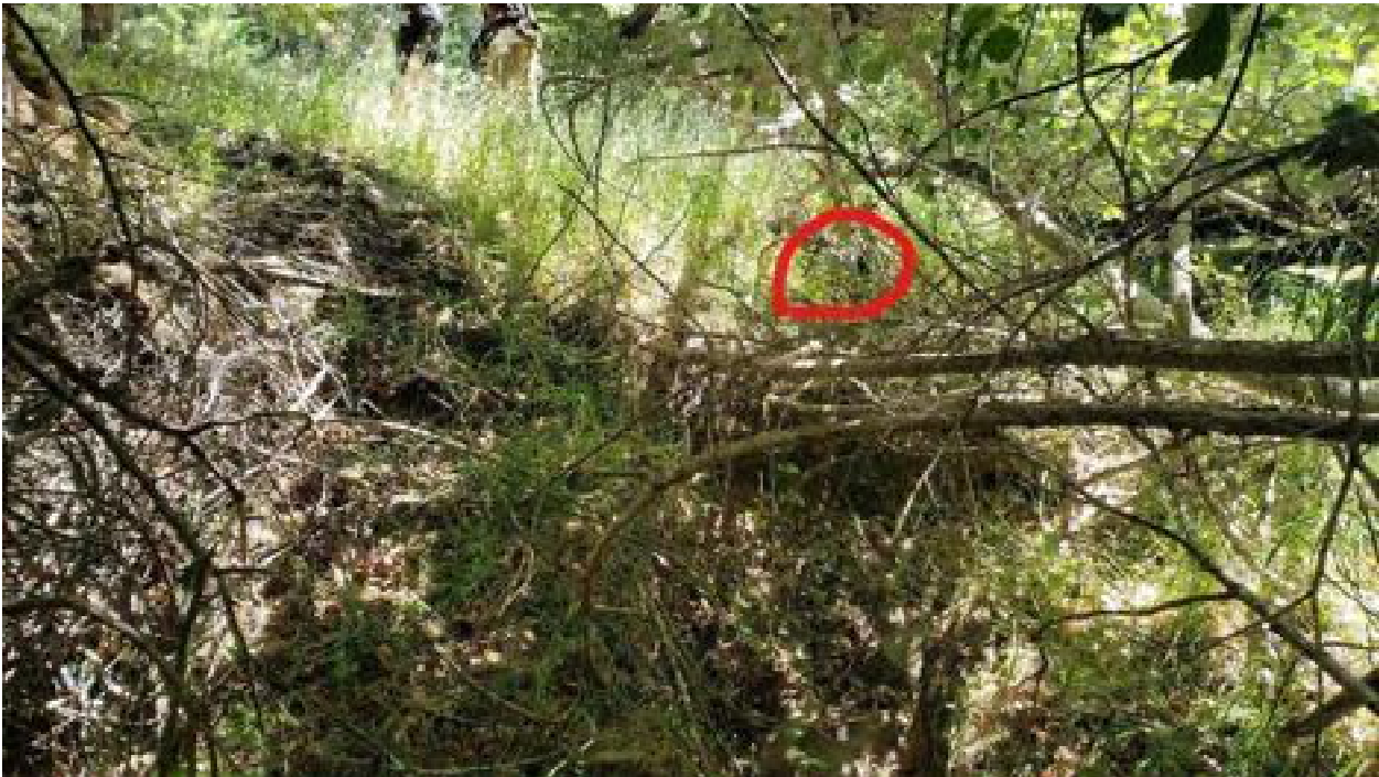
Site 35. Looking at the outlet(circled). The culvert upgrade will re-align the watercourse to its original channel, which will require the outlet to be placed in the lower left of the photo.
