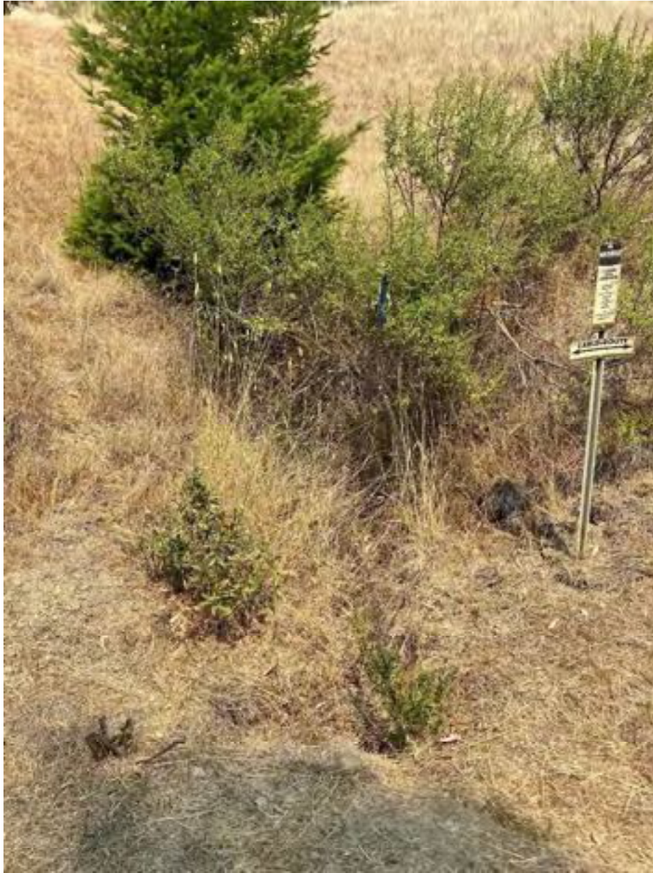
Photo 31: Stream Crossing 08. Looking upstream from the inlet of the 8-inch diameter culvert at stream crossing 08. Photo date 9-1-2021.
