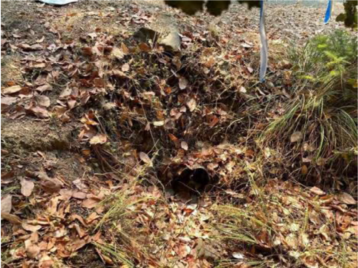
Photo 25: Stream Crossing 07. Looking downstream towards the inlet of the 12-inch diameter culvert at stream crossing 07. Photo date 9-1-2021.
