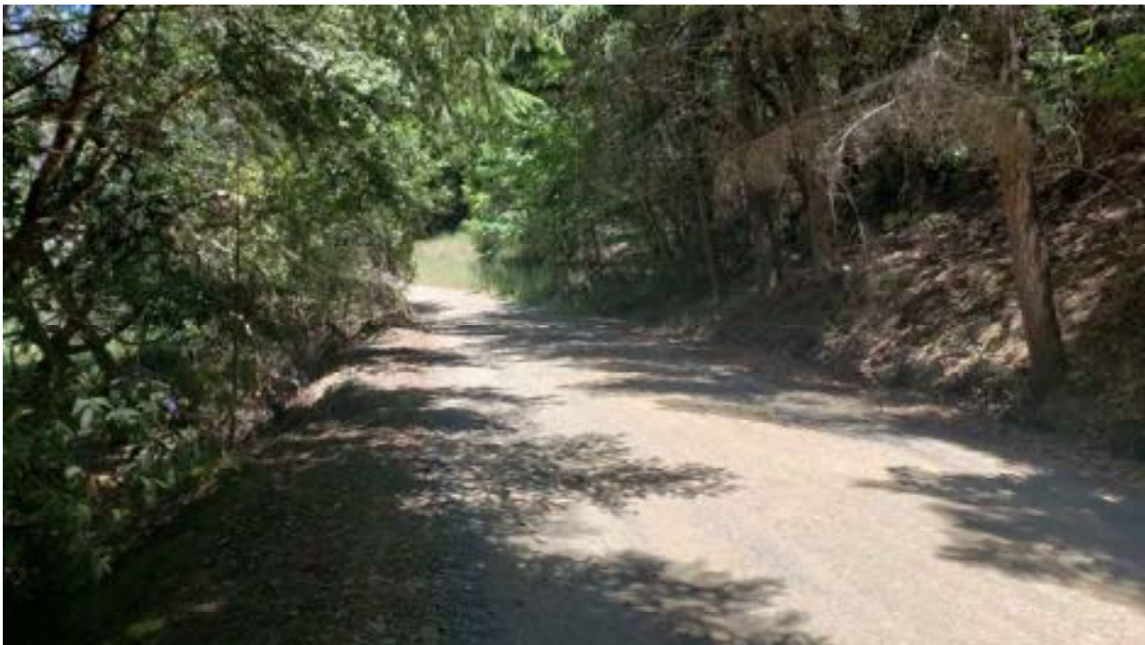
Site 14. Looking up grade towards Site 13.
