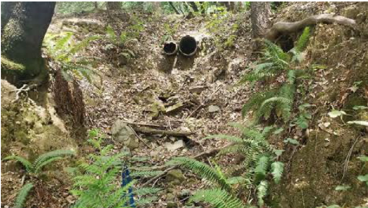
Outlet of watercourse crossing at Site 23. Blue flag represents proposed outlet of culvert upgrade.
