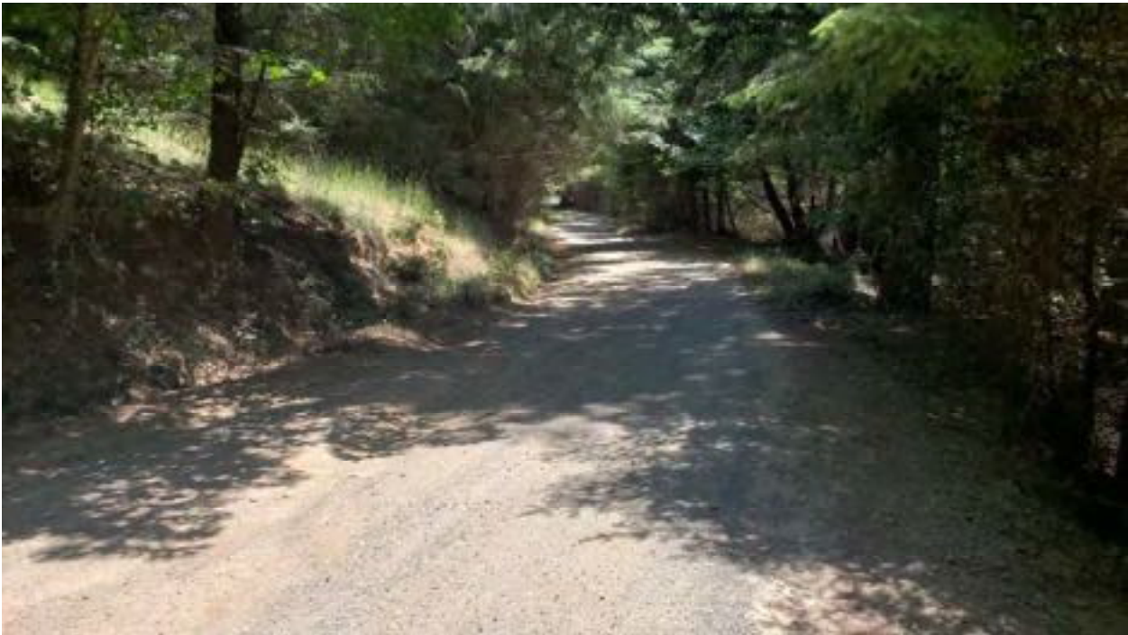
Site 14. Looking down grade at Site 14 with Site 15 further down grade a short distance.
