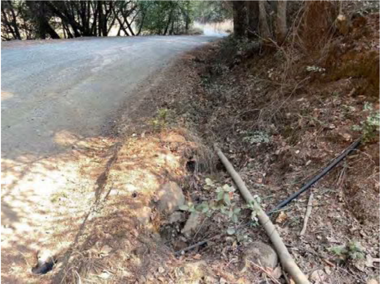
Photo 44: Stream Crossing 13. Looking upslope from the inlet of the DRC along the inside ditch that is currently diverting the flow away from the native stream channel at stream crossing 13. Photo date 9-1-2021.
