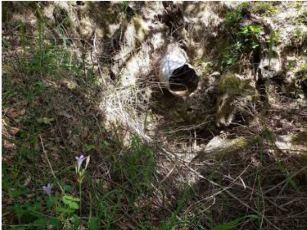
Site 05. Looking at the outlet.
