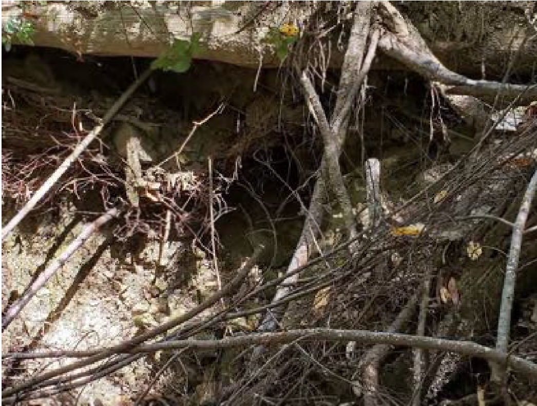
Site 06. Looking at the outlet.
