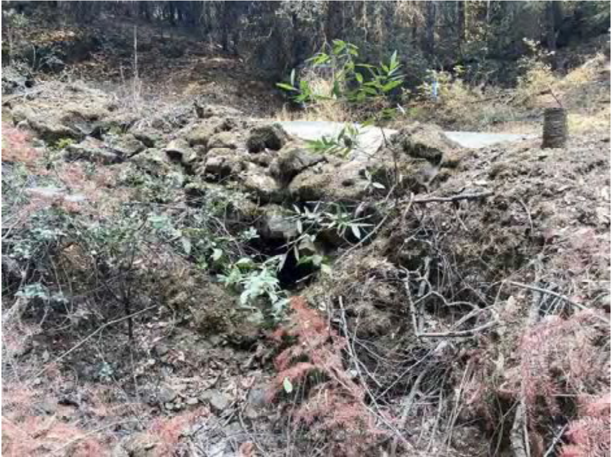
Photo 71: Stream Crossing 26. Looking upstream towards the outlet of the 18-inch diameter culvert at stream crossing 26. Photo date 9-1-2021.
