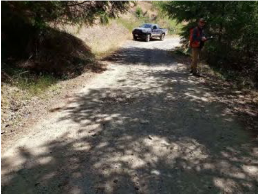
Site 05. Looking up grade to the east towards Site 04..
