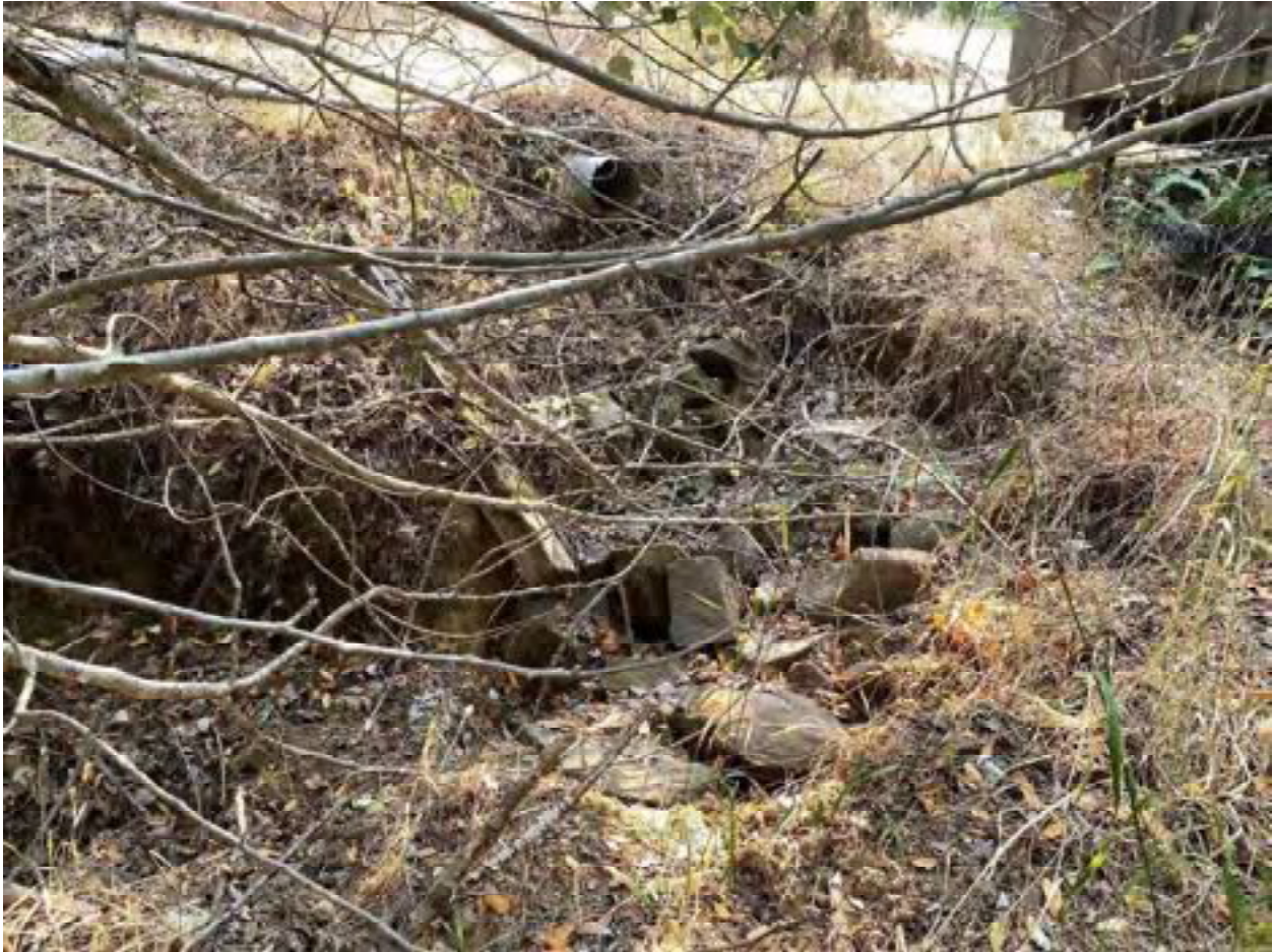
Photo 76: Stream Crossing 35. Looking upstream towards the outlet of the 8-inch diameter culvert at stream crossing 35. Photo date 9-1-2021.
