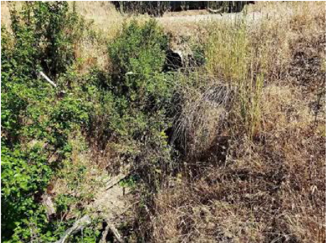
Site 03. Looking at the outlet.
