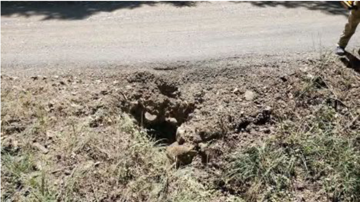
Site 26. Inlet of the watercourse crossing.
