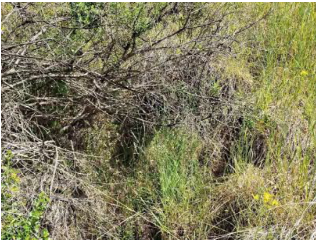
Site 08. Looking at the outlet of the culvert.
