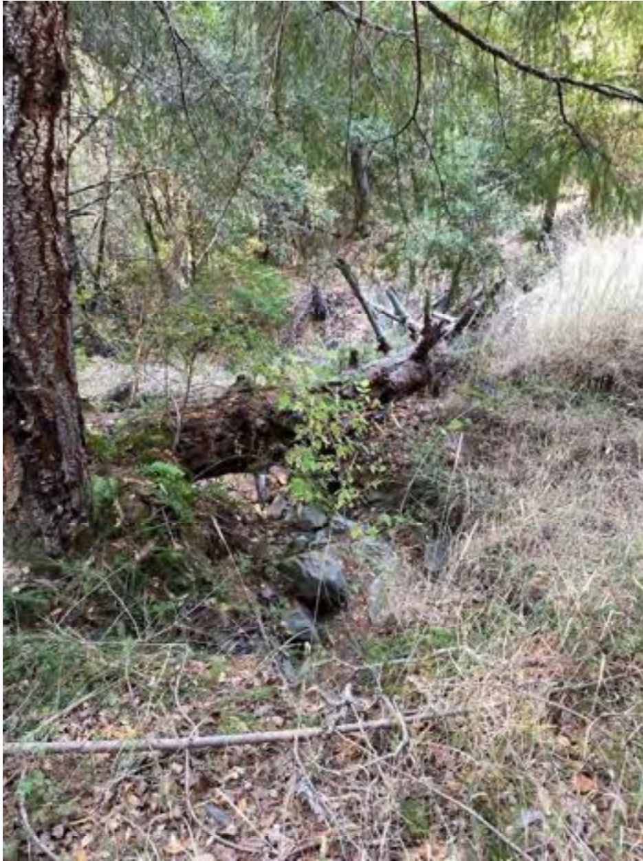
Photo 56: Stream Crossing 19. Looking downstream from the outlet of the 18-inch diameter culvert at stream crossing 19. Photo date 9-1-2021.
