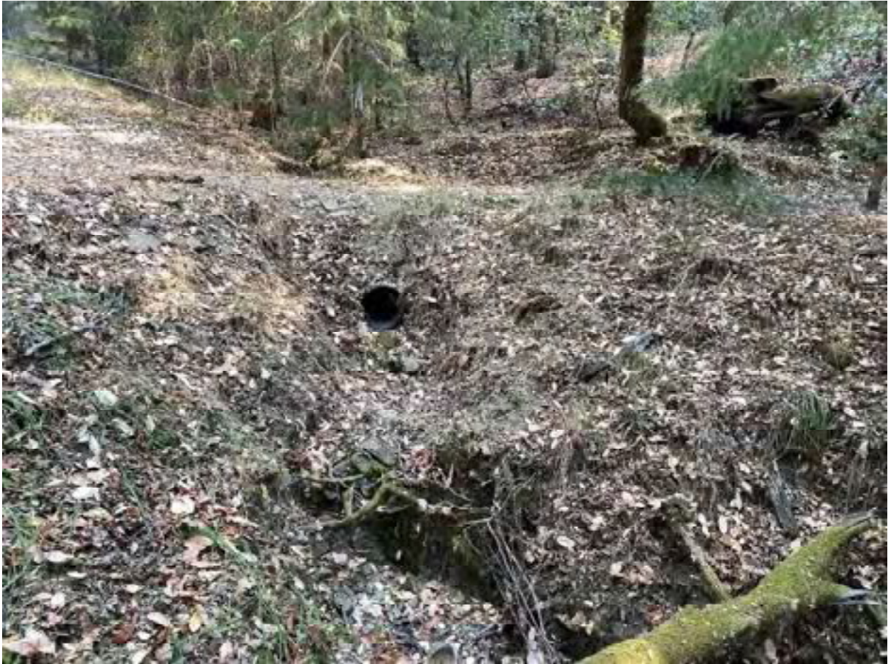
Photo 50: Stream Crossing 17. Looking upstream towards the outlet of the 18-inch diameter culvert at stream crossing 17 that is proposed for removal. Photo date 9-1-2021.
