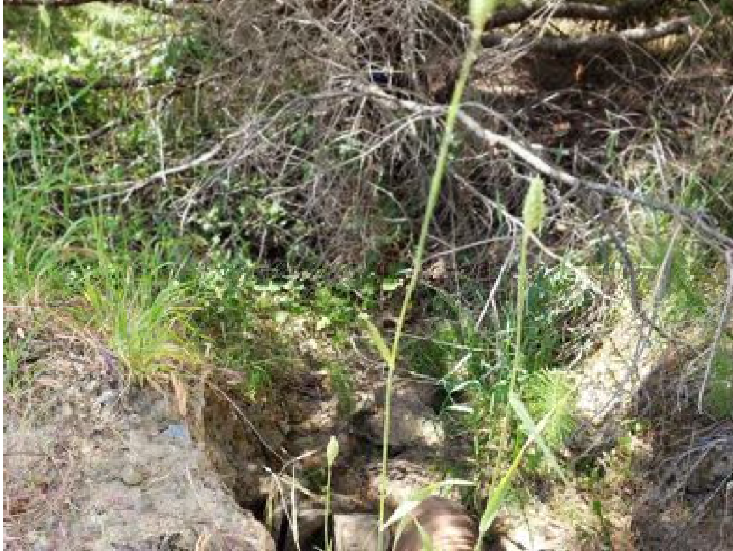
Site 07. Looking down channel from the outlet. The upgraded culvert will outlet approximately in the brush to the upper center of the photo.
