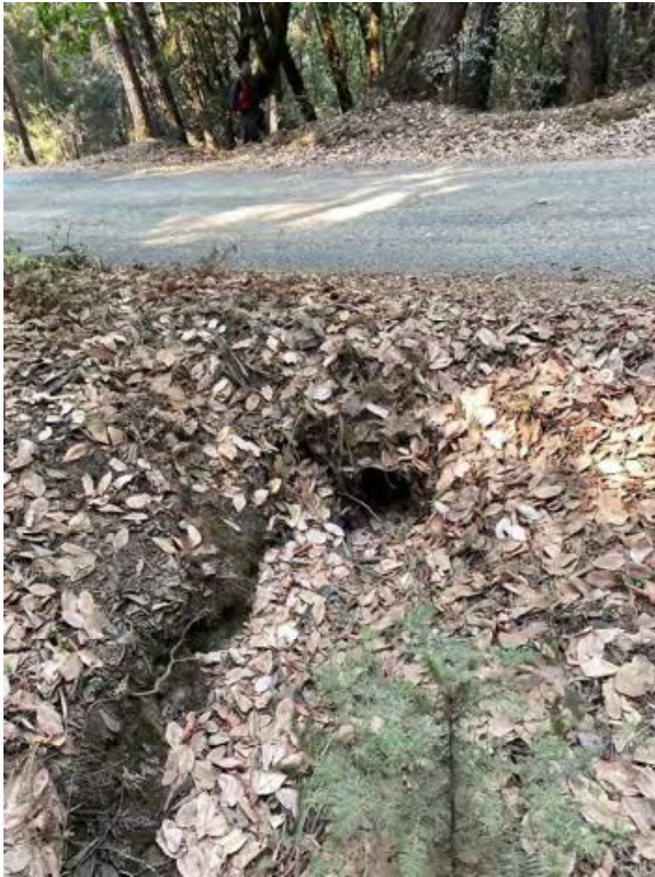
Photo 63: Stream Crossing 24. Looking downstream towards the inlet of the 18-inch diameter culvert at stream crossing 24. Photo date 9-1-2021.
