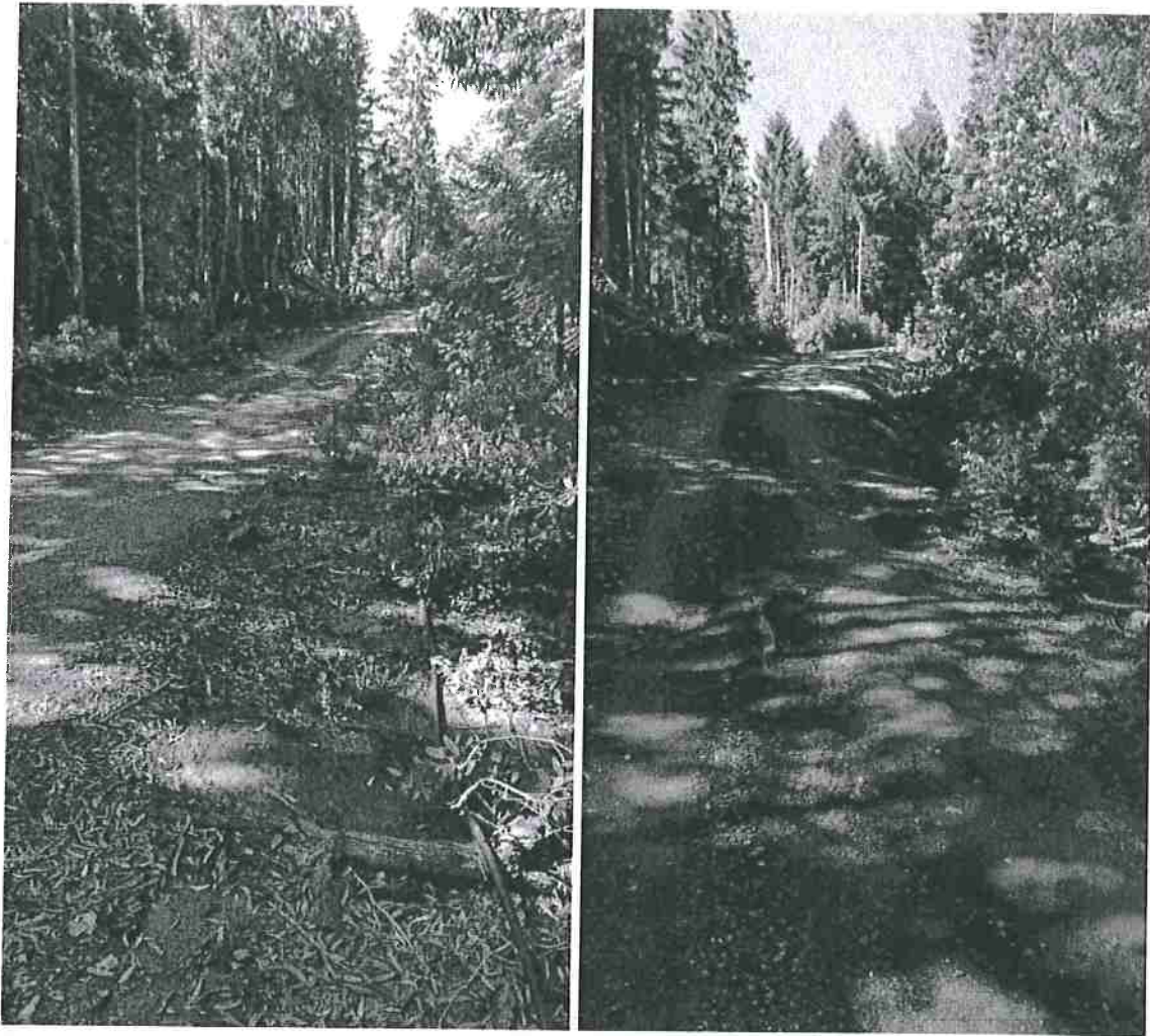
Road Point 5: Surface erosion is occurring down a road slope and the side of the road, following it until it eventually dissipates. Owner will place a water bar above the rilling to reduce erosion down the road slope and place a rolling dip at the bottom so that water is adequately diverted. 7/12/2016
