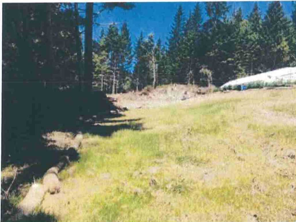
Picture 4: Cultivation conversion site. Area has been cleared and graded, however the grading did not involve significant cuts and/or fill. Photo date 6-23-2018.
