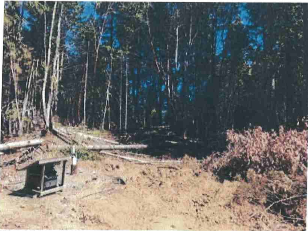
Picture 6: Area of clearing associated with pond construction.
