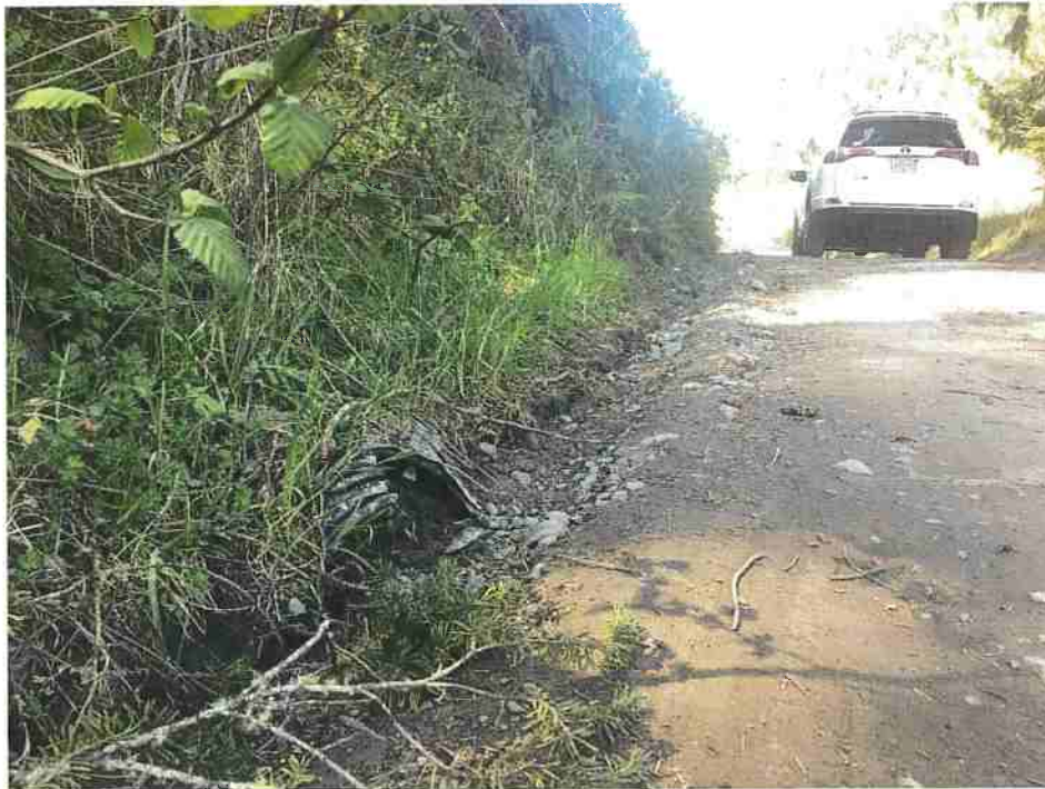
Figure 6: RP3. 14' Paved road width; lead-out ditch. Image shown facing west.
