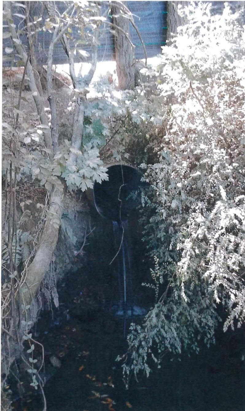
Picture 1: This is a photograph of the outlet of the culvert at Map Point 1. This culvert diameter is 36 inches and calculations for the 100 year peak flow should be at least a 60 inch diameter culvert. Physical examination did not show signs of an undersized culvert. As an alternative to culvert replacement at this time, a rocked outfall should be installed at this location. Rock armoring should extend from the bottom of the steambed up to the edge of the road surface. Photo date 8-4-2016.
