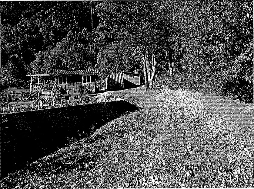
Photo 2 – Dug in cultivation area with concrete footings and retaining wall; watercourse is amongst trees on right side of image
