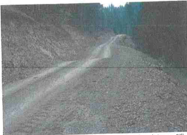
Figure 8. Rolling dips installed to drain an out-sloped road. Source: Bill Weaver, Pacific Watershed Associates.
