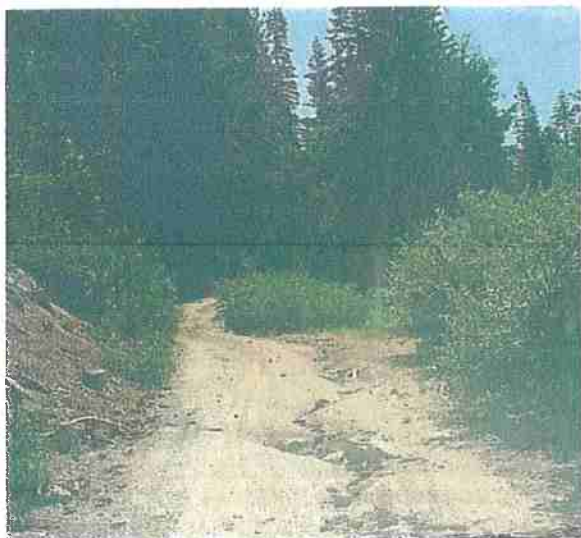
Figure 37. Pinchard Creek road with rilling along the road surface before the project, 2002. Photo: Joe Hoffman, Plumas National Forest.
