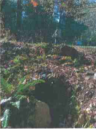
Picture #40 Cobb Rd looking @ 12" culvert inlet
