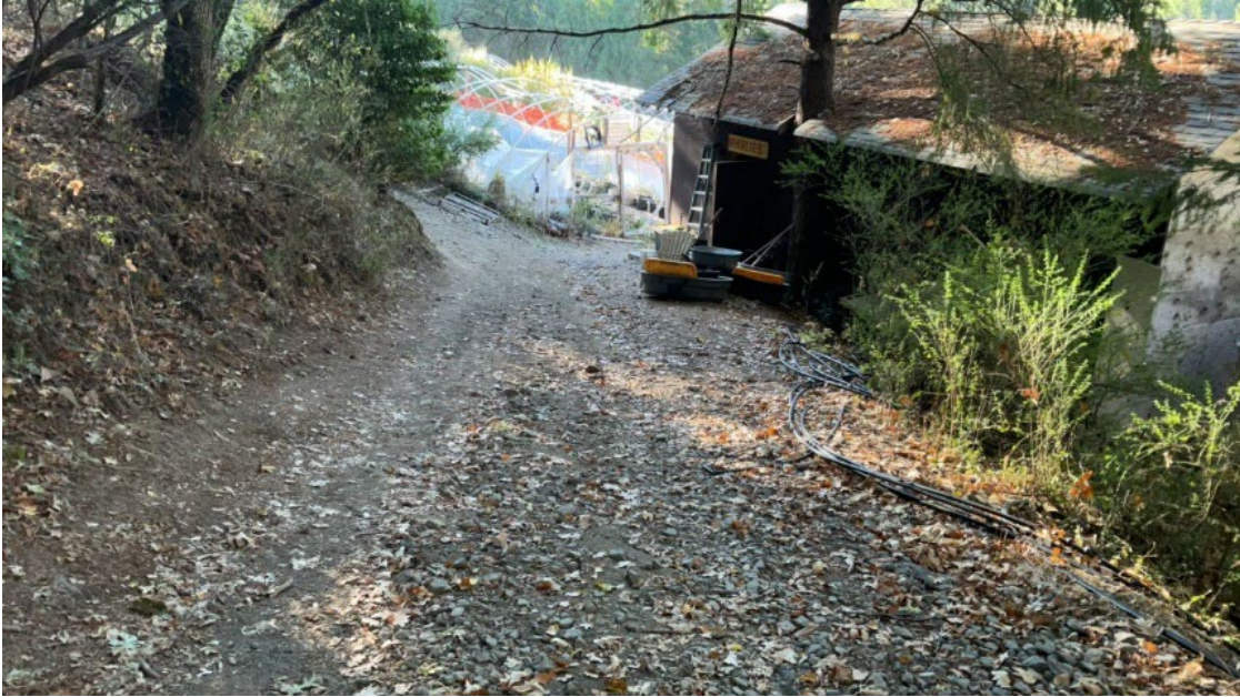
Figure 13. Point 4. Driveway to CA2 is steep and lacks drainage; stormwater runoff is concentrated into the cultivation and storage area.
