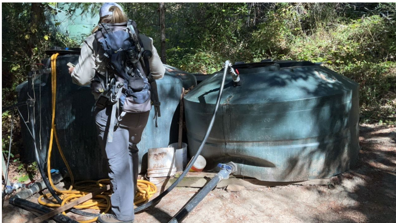
Figure 38. Point 16. The surface water diversion line from Point 2 connects to water storage tanks above CA1 at Point 16 and appears to be used to irrigate.
