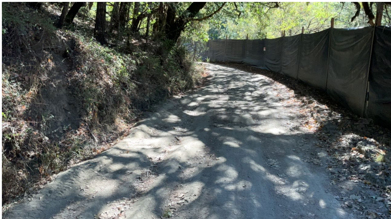
Figure 33. The access road ditch and rilled road surface poses threat of sediment delivery to the stream crossing at Point 12.
