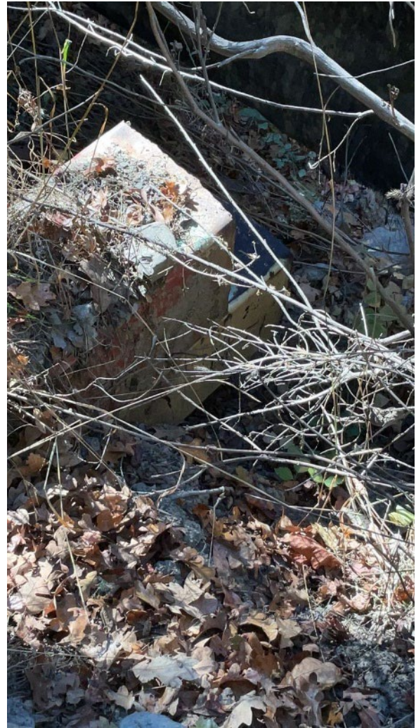
Figure 32. Point 12. The stream crossing is undersized and comprised of two stacked box pipes.
