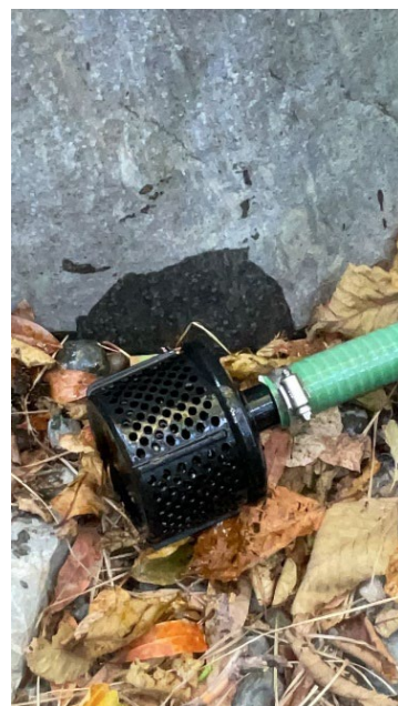
Figure 10. Point 2. Surface water diversion intake screen.
