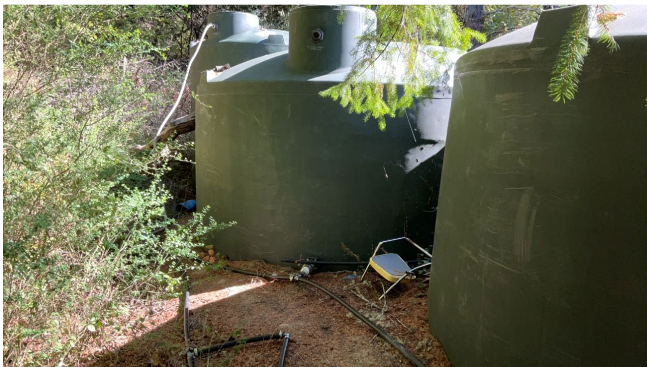
Figure 39. Point 16. The surface water diversion line from Point 2 connects to water storage tanks above CA1 at Point 16 and appears to be used to irrigate.
