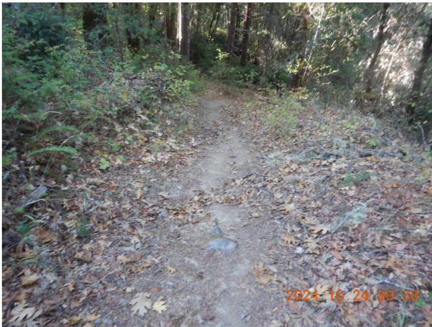
Figure 12. Point 3. Water bar needs to be reinforced.
