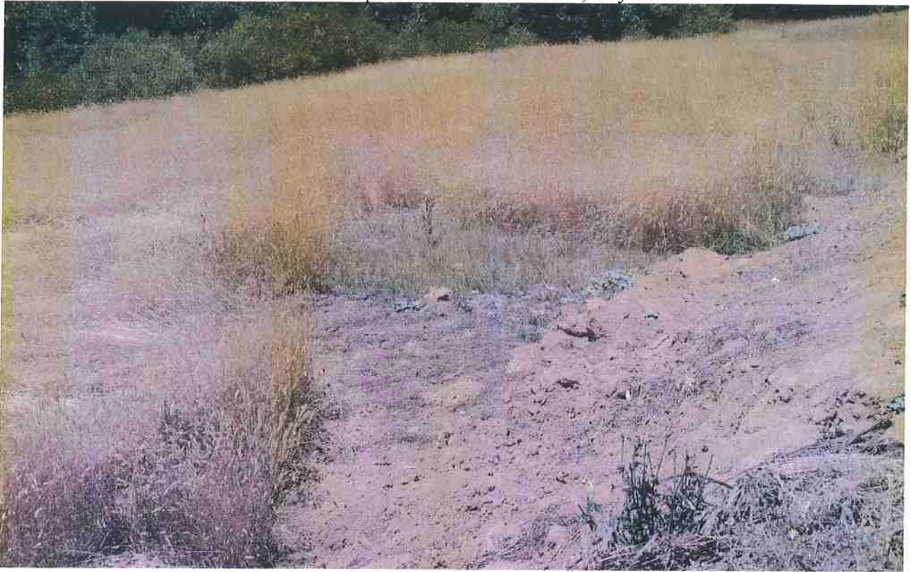
Upper flat with fillslope failure into wetland area July 13, 2016
