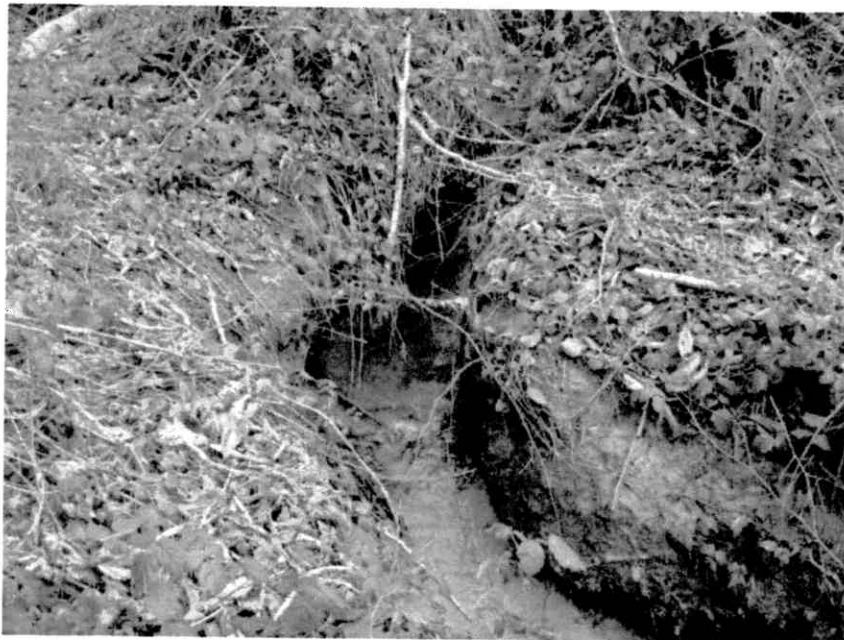
Photo 6. Photo 6 was taken adjacent to sample point 8, which is located on the floodplain. This photo shows the drainage feature located in the low-lying portion of the site. Photo taken by SHN on 2-13-07; orientation is to the south
