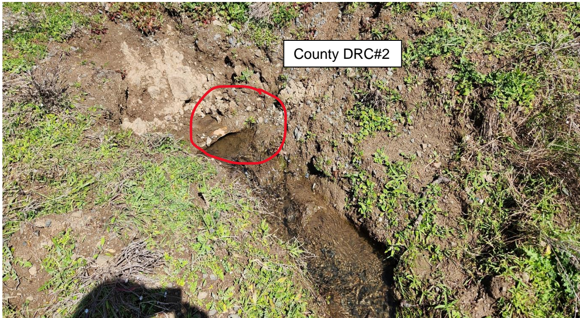
County DRC#2 partially plugged outlet (Photo by Omsberg & Preston Staff, March 16, 2023)
