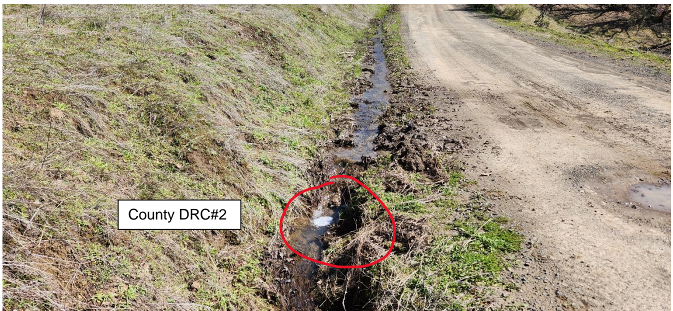
County DRC#2, partially plugged inlet (Photo by Omsberg & Preston Staff, March 16, 2023)
