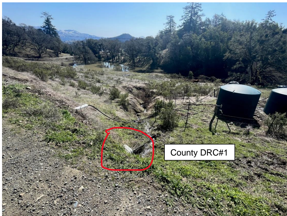
County 16" (15.5") CMP DRC#1 on Lauffer Road, Looking South (Photo by Omsberg & Preston Staff, March 16, 2023)
