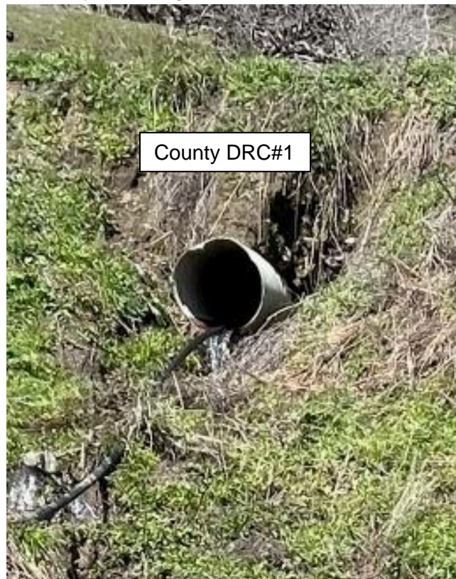
Gully created by shot-gunned County DRC#1 (Photos by Omsberg & Preston Staff, March 16, 2023)
