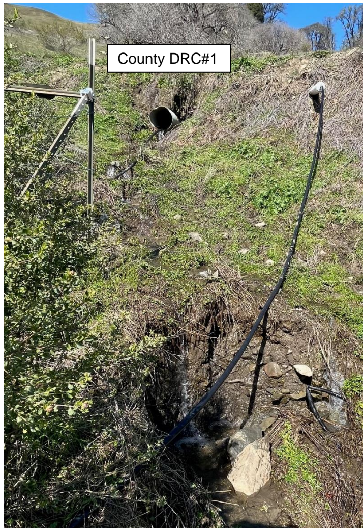
Gully created by shot-gunned County DRC#1 (Photos by Omsberg & Preston Staff, March 16, 2023)
