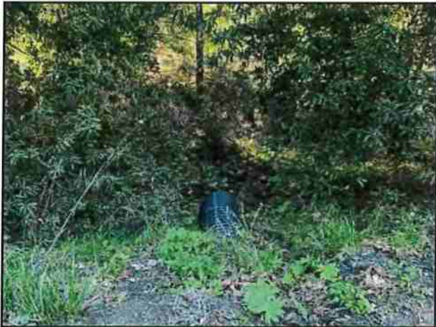
Photo #195 Blue Rock Rd Looking@ 18" Culvert Out
