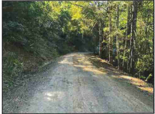
Photo #34 APN #223-034-005 Private Access Rd @ Pullout Looking SE @ Curve
