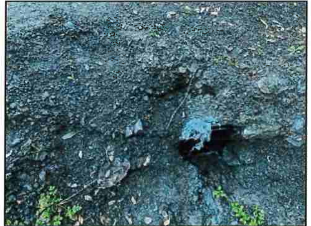
Photo #4 APN #223-034-005 Private Access Rd Looking @ 8" Culvert In
