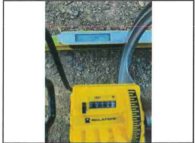
Photo #56 APN #223-034-005 Private Access Rd Width 12'4" Slope 17.2%
