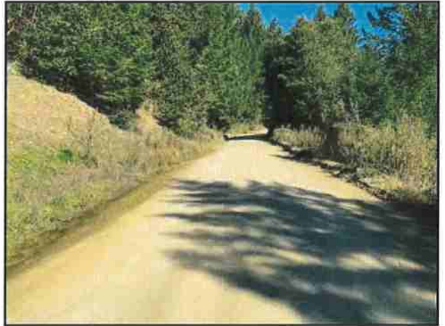
Photo #106 Blue Rock Rd @ Looking North
