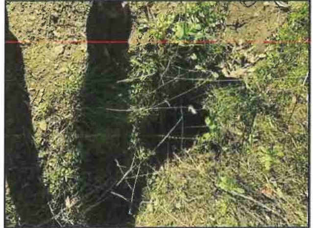
Photo #104 Blue Rock Rd Looking@ Shorth 18" Culvert In
