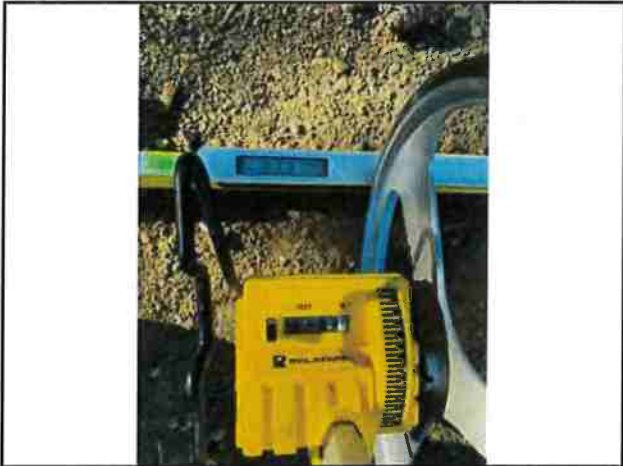
Photo #39 APN #223-034-005 Private Access Rd Width 16'8" Slope 21.3%
