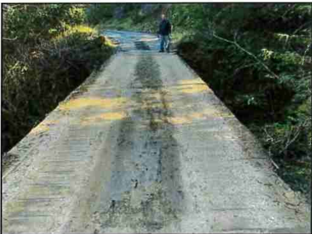
Photo #89 Blue Rock Rd Bridge Looking NE
