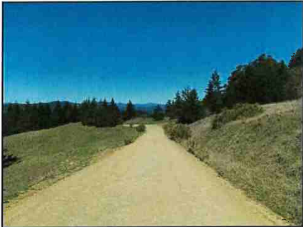
Photo #231 Blue Rock Rd @ Looking NW
