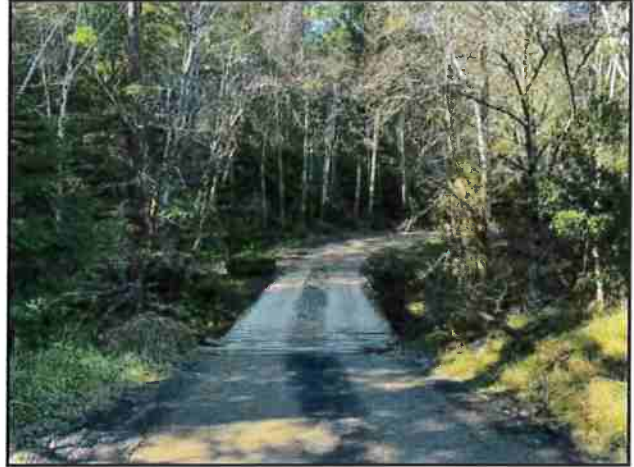
Photo #86 Blue Rock Rd Bridge Looking SW
