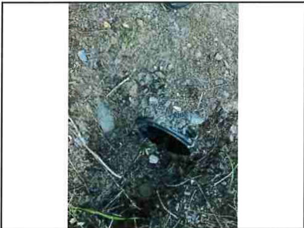
Photo #5 APN #223-034-005 Private Access Rd Looking @ 8" Culvert Out
