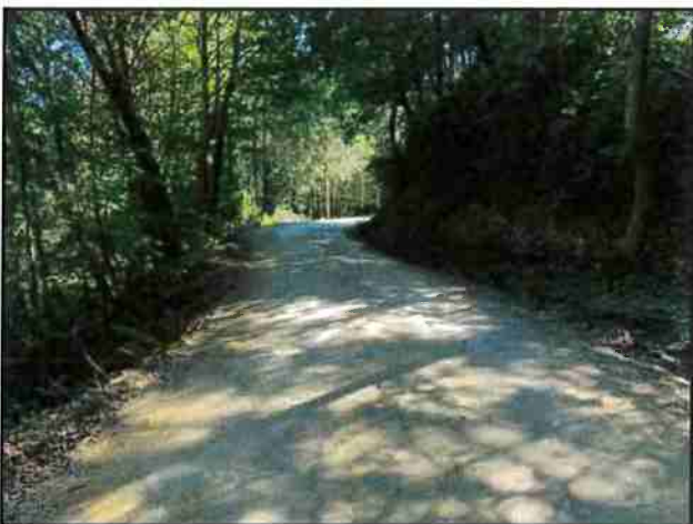
Photo #149 Blue Rock Rd@ Pullout Looking SE Towards Curve
