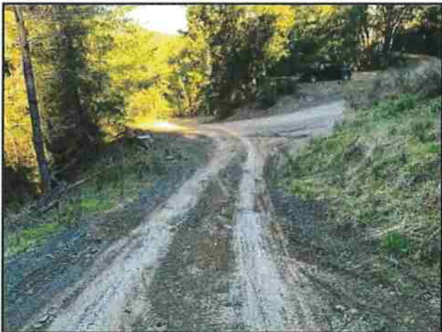
Photo #21 APN #223-034-005 Private Access Rd @ Curve w/ Pullout Looking NW
