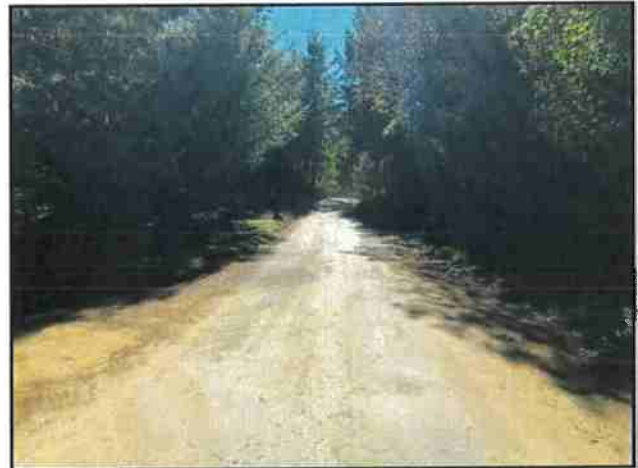
Photo #166 Blue Rock Rd@ Road Intersection Looking SE
