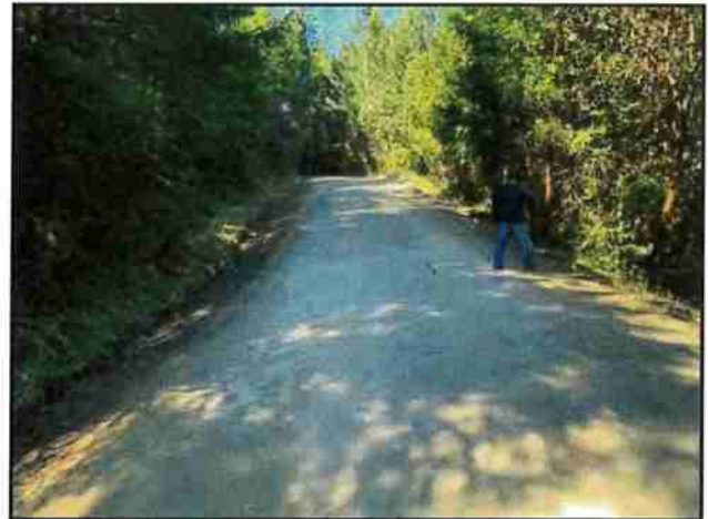
Photo #136 Blue Rock Rd @ Pullout Looking NW
