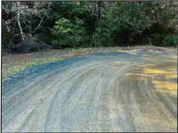
Photo #63 APN #223-034-005 Private Access Rd @ Curve w/ Pullout Looking SW
