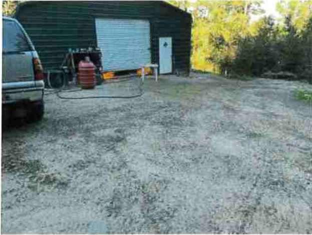
Photo #1 APN #223-034-005 Private Access Rd Looking @ Turnaround
