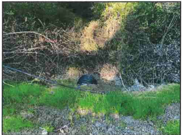
Photo #84 Blue Rock Rd Looking @ 18" Culvert Out
