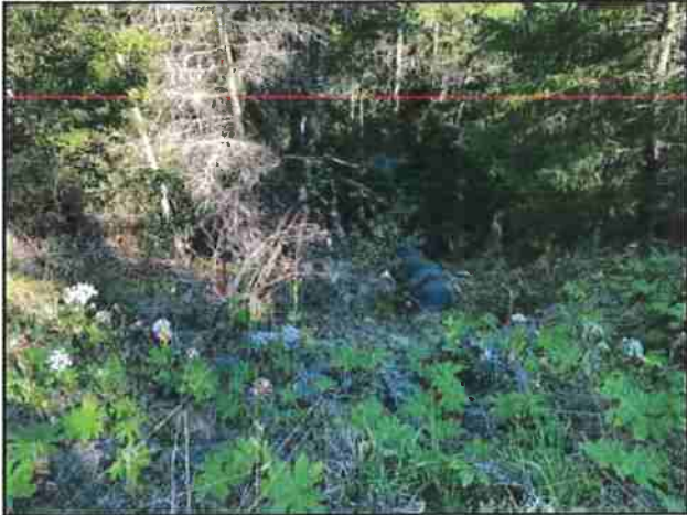
Photo #139 Blue Rock Rd Looking@ 18" Culvert Out
