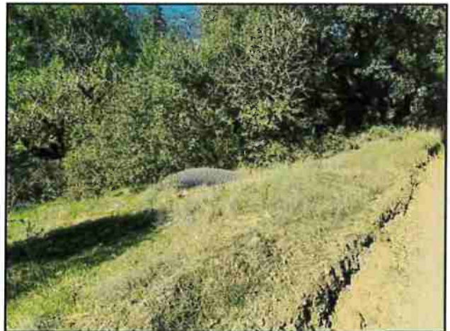
Photo #256 Blue Rock Rd Looking@ 18" Culvert Out
