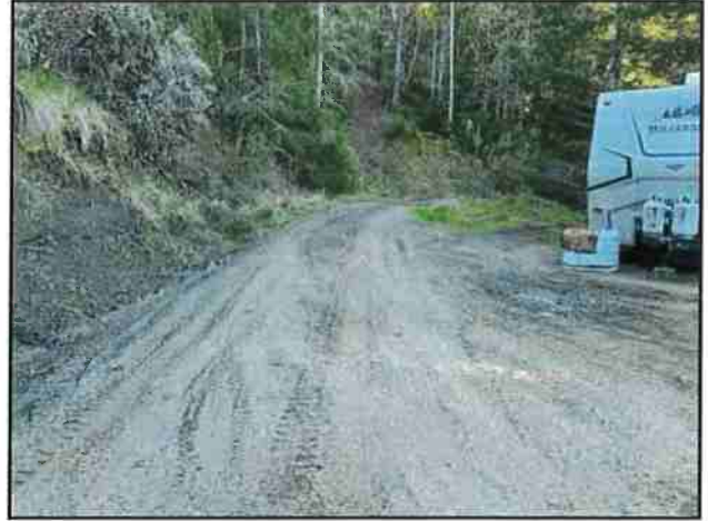
Photo #2 APN #223-034-005 Private Access Rd @ Pullout Looking North @ Curve
