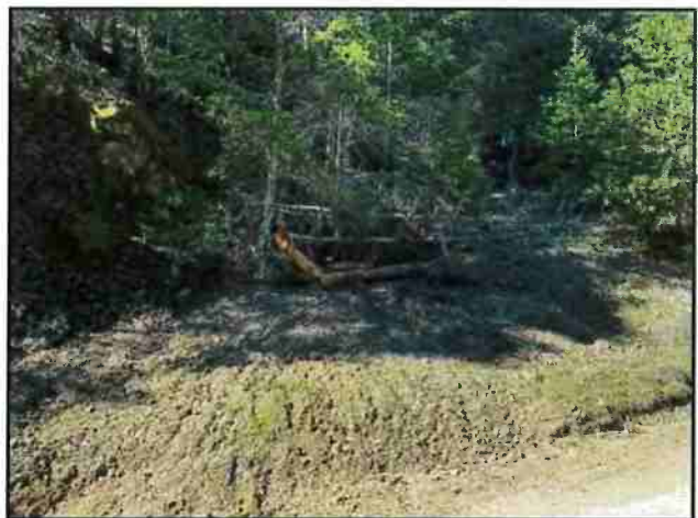
Photo #174 Blue Rock Rd Looking @ Old Culvert To Be Removed
