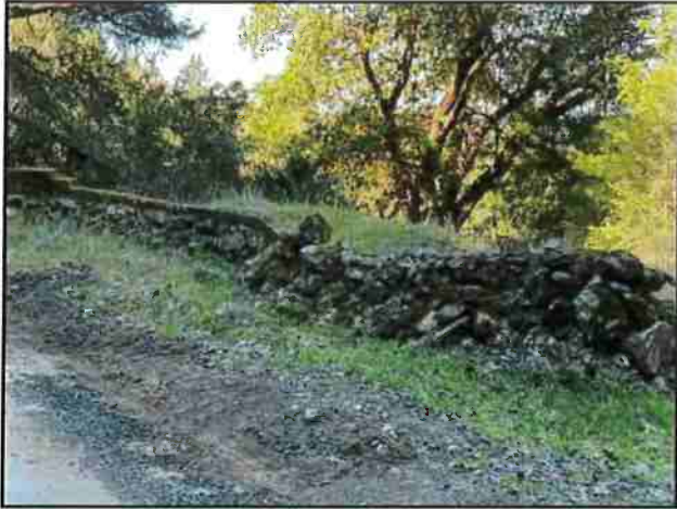
Photo #181 Blue Rock Rd Looking@Wall Along Road
