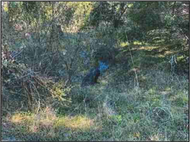
Photo #105 Blue Rock Rd Looking@ 18" Culvert Out
