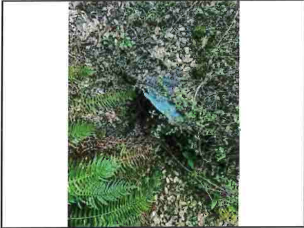
Photo #13 APN #223-034-005 Private Access Rd Looking@ 12" Culvert In
