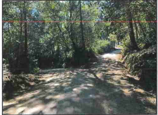
Photo #152 Blue Rock Rd@ Curve w/ Pullout Looking SE Towards Driveway
