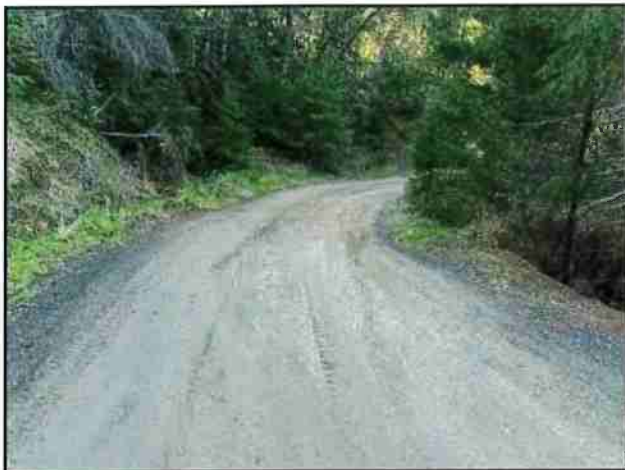
Photo #17 APN #223-034-005 Private Access Rd @ Curve w/ Pullout Looking NW
