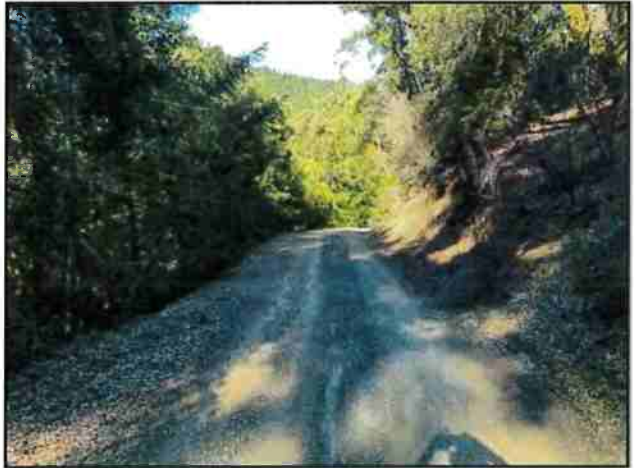
Photo #52 APN #223-034-005 Private Access Rd @ Pullout Looking NW
