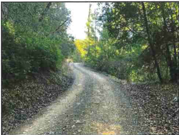
Photo #71 APN #223-034-005 Private Access Rd @ Curve w/ Pullout Looking SW
