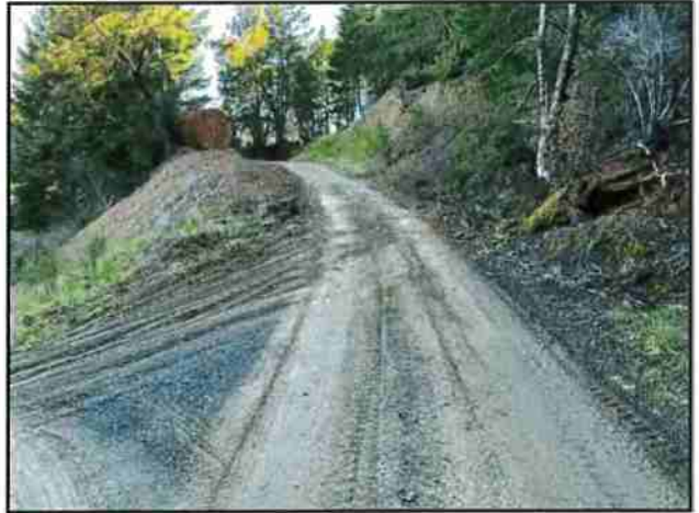
Photo #16 APN #223-034-005 Private Access Rd @ Pullout Looking NE @ Curve & Fuel Tank
