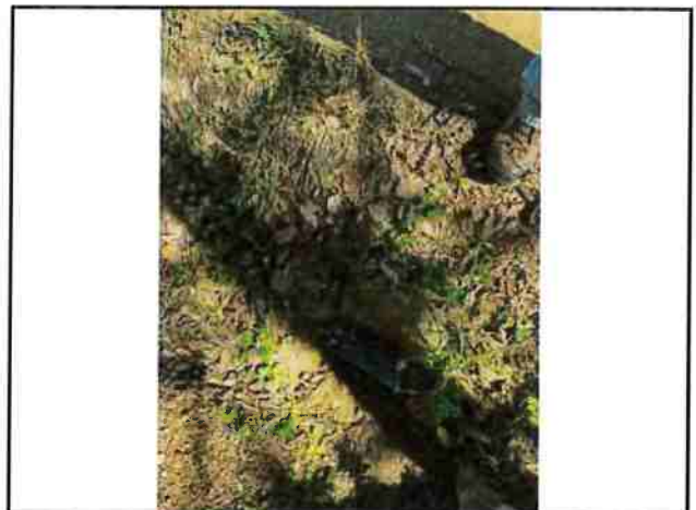
Photo #160 Blue Rock Rd 18" Culvert In
