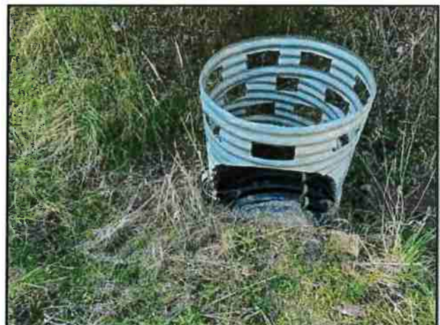
Photo #138 Blue Rock Rd Looking @ 18" Culvert In
