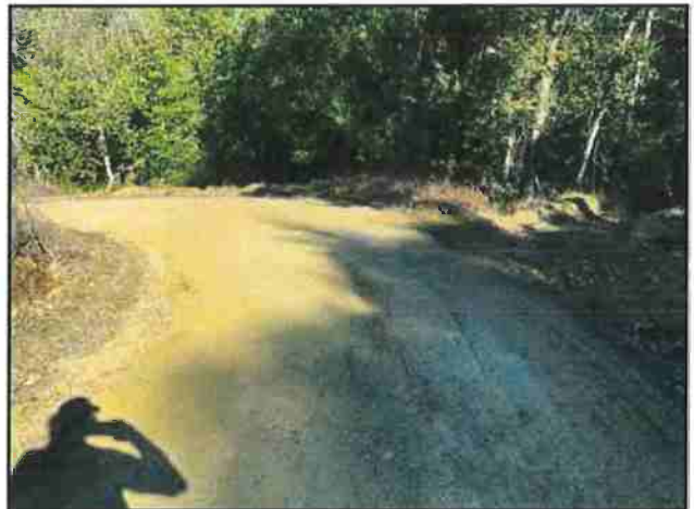
Photo #58 APN #223-034-005 Private Access Rd @ Curve w/ Pullout Looking NW
