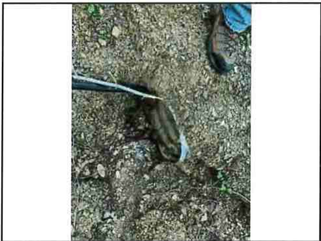
Photo #41 APN #223-034-005 Private Access Rd Looking@ 12" Culvert In
