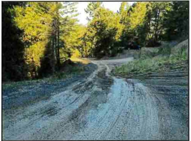
Photo #18 APN #223-034-005 Private Access Rd @ Curve w/ Pullout Looking SW
