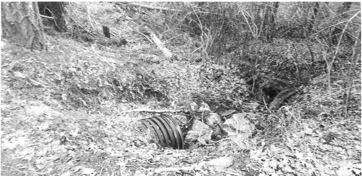
Photo looking at the outlet of the watercourse crossing at Site 08.
