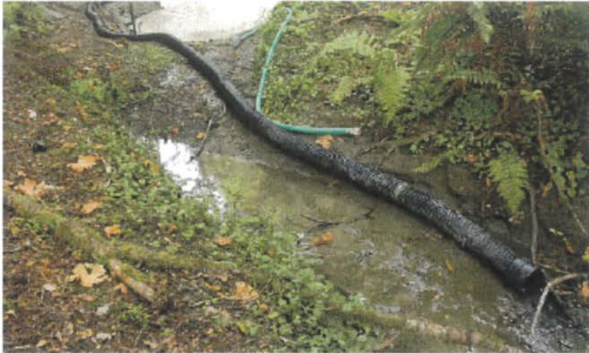
FIGURE 197. Flex pipe stream diversion around a road construction site. The inlet to this 6 inch diameter flex pipe inlet collects clear streamflow from a retention dam above the project site and gravity feeds it around the project area and back into the natural channel downstream from construction work (see photo).
