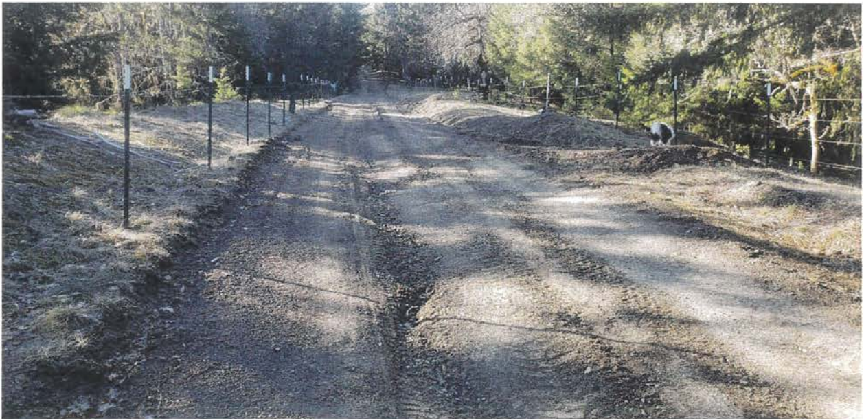
Photo looking up grade at Site 01.
