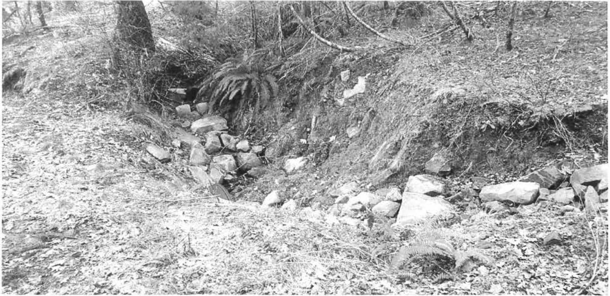
Photo looking at the inlet of the watercourse crossing at Site 08.
