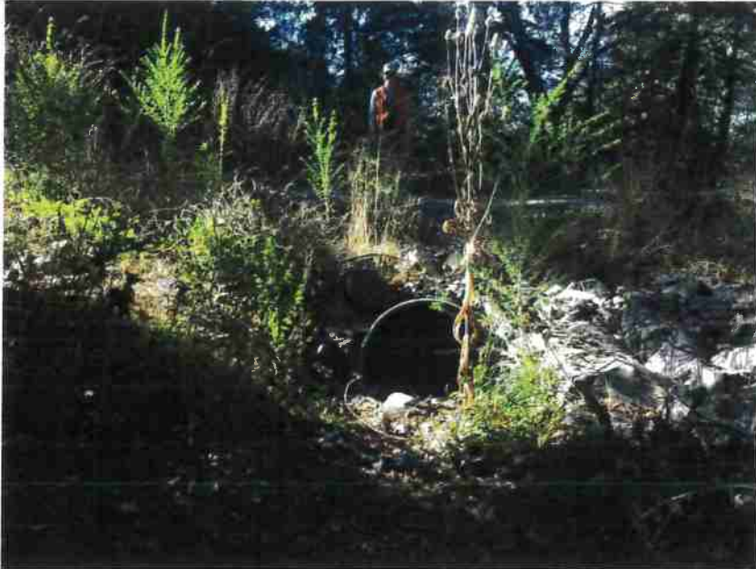
Photo 7, MP#5 – SC#3 , view of 42-inch diameter culvert inlet (Photo November 2018).
