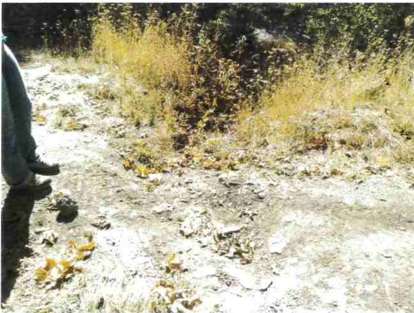
Photo 14, MP#9 – SC#7 , no formal drainage structure on a near origin Class III stream, view looking downstream from road bed (Photo September 2016).
