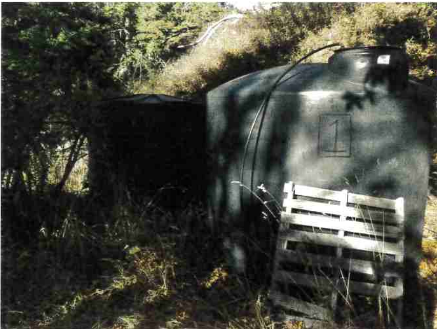
Photo 26, MP#20 – View of two water storage tanks (3,000 gal and 2,825 gal) located less than 50 feet from a Class III stream (Photo September 2016).
