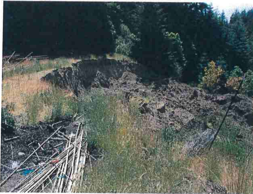
Photo 1-5A: Outboard landing fillslope failure looking southeast from the right edge of head scarp. (Photo taken June 13, 2016).
