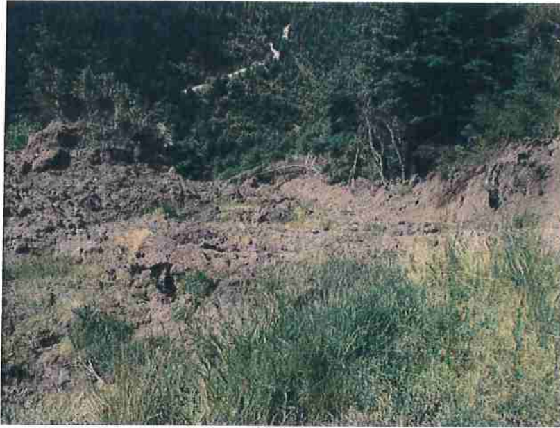
Photo 1-5C: Outboard landing fillslope failure looking downslope from near the center of feature. (Photo taken June 13, 2016).
