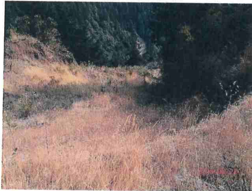
Photo 2-5C: Outboard landing fillslope failure looking downslope from near the right center of feature. Note natural revegetation of bare soil areas as compared to 2016 photos. (Photo taken August 22, 2018).
