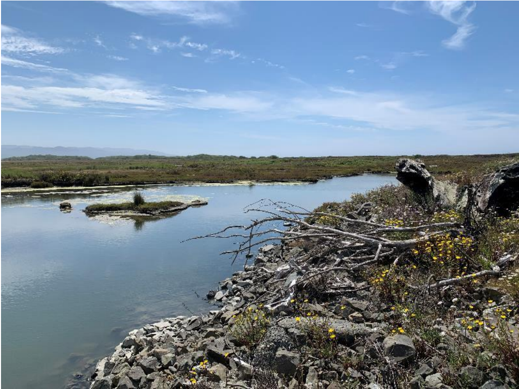
Photo 14—Rocked levees around the tide gate, facing southwest.
