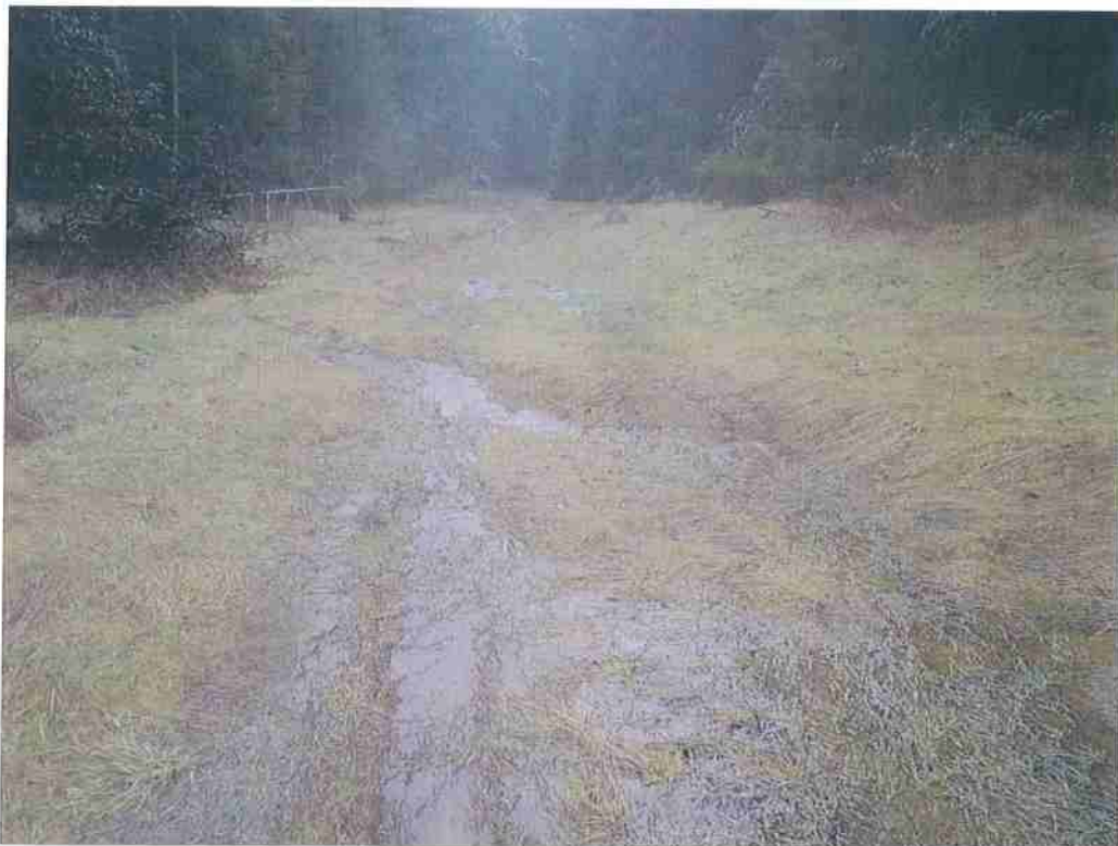
Photo 10. Project 3; Looking down road (towards Left Bank of crossing) at failed ranch road waterbar.
