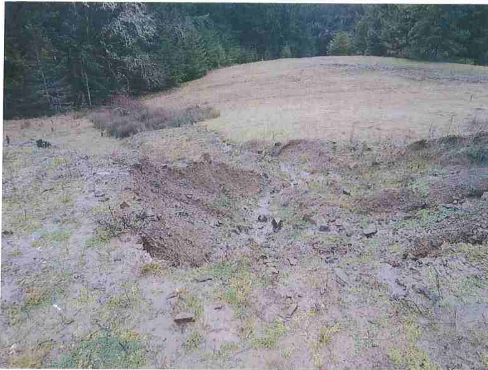
Photo 4. Project 1; Looking Downslope at Fill Failure caused by flow from NE corner of terrace.
