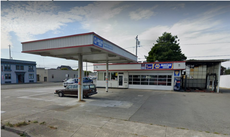
Figure 3: Existing Structures at 803 4th Street
