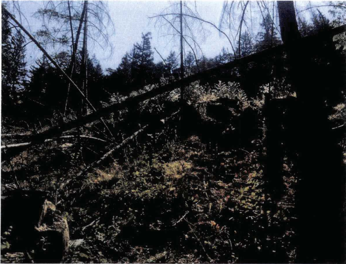
Picture 5: Untreated slash, logs, and woody debris located along the western perimeter of Cultivation Site 2 south of Map Point B. Portions of the fill slope in this area are intermixed with stumps, logs, and woody debris. Treatment of this "unstable fill" requires removal of all buried woody material (stumps, logs, limbs, chunks, etc.). Photo date 8-14-2018.
