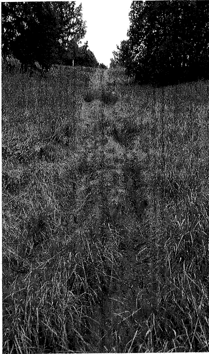
Pictures 1: This is a picture of the rutting segment of atv trail (Segment 06) that is located down the shallow swale that eventually connects with a Class II Watercourse. Use of this atv trail should be discontinued. Photo date 2/26/2016
