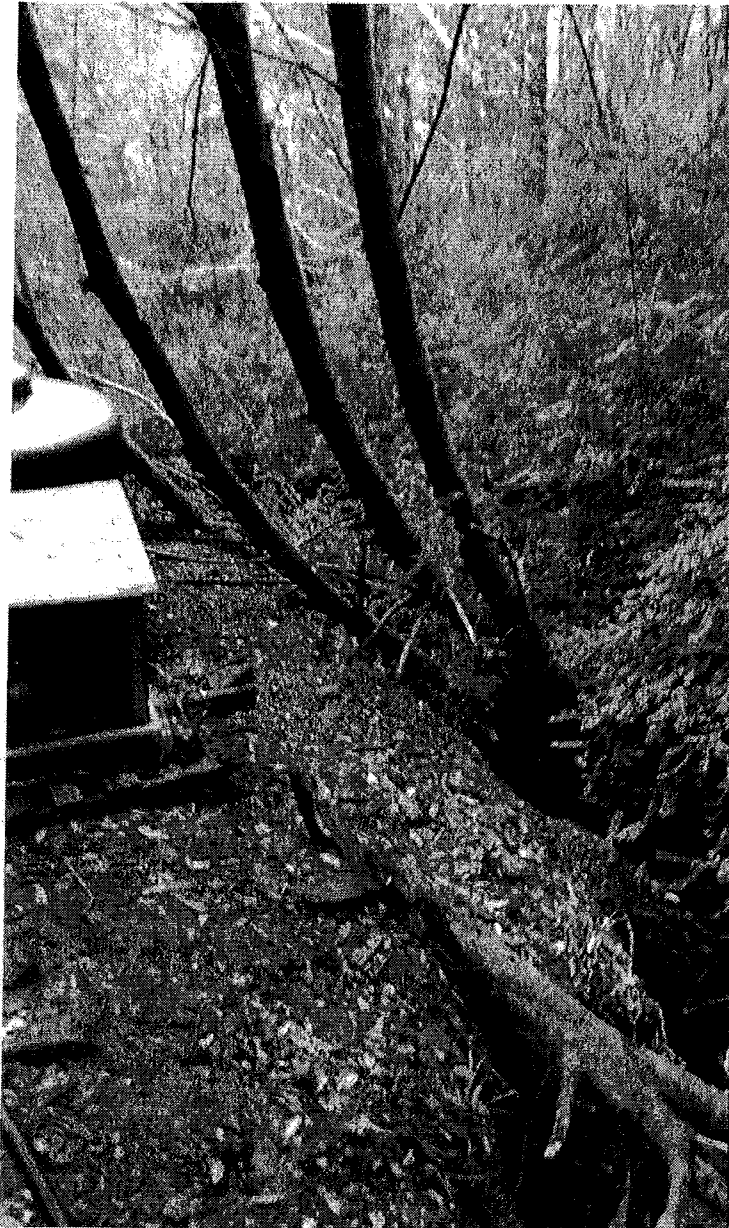
Picture 16: This is a picture that shows the location of the holding tanks and water pump in relation to the undercut bank that it is situated on and the watercourse below. The watercourse is located approximately 6 to 8 vertical feet below the three forked hardwood tree in the picture. Photo date 2/26/16.
