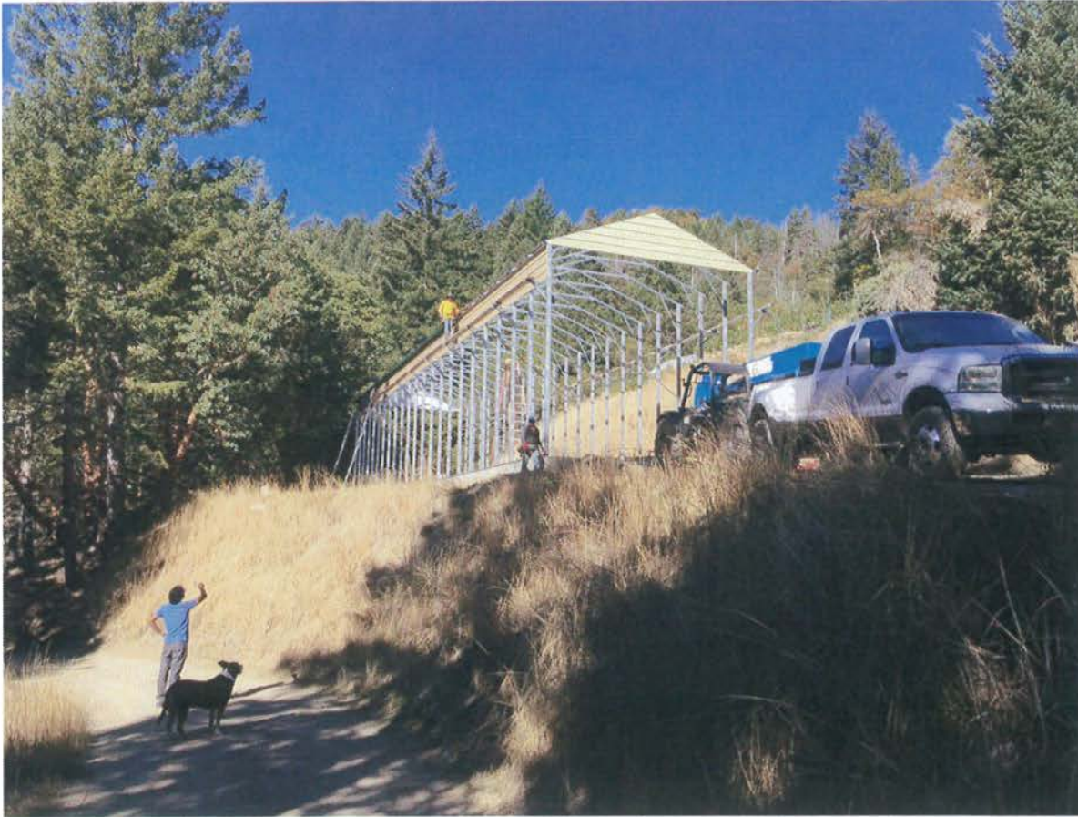
Photo 8: View of Drying and Storage Building facing northwest.
