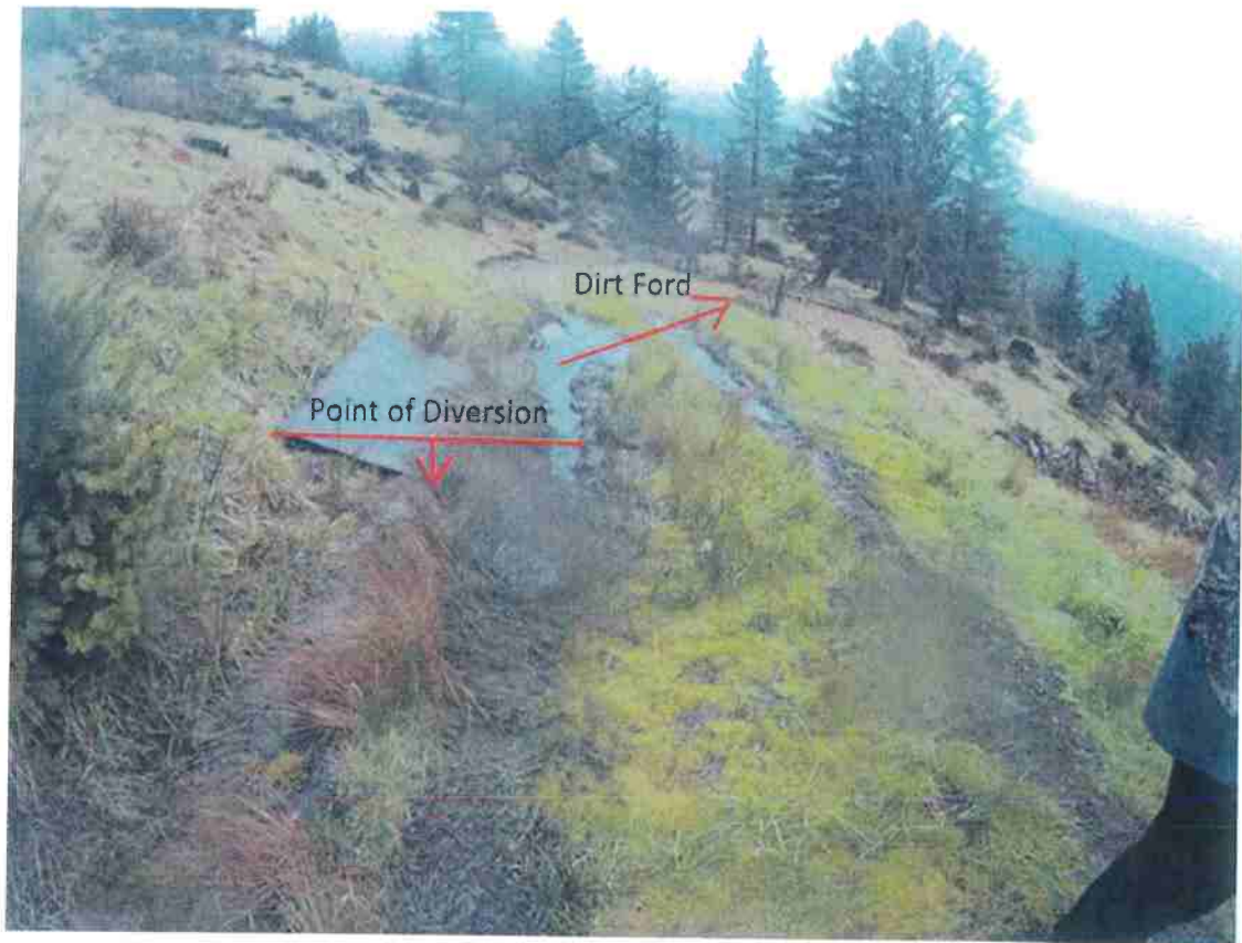
Site 12 the point of diversion and Site 11 a dirt ford. Bank seep drains across legacy hunting road. It is being recommended to install a water bar at Site 11 to ensure the bank seep does not drain down the road surface.
