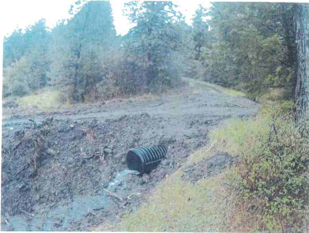
Site 09 – 24" ditch relief culvert. Functioning adequately.
