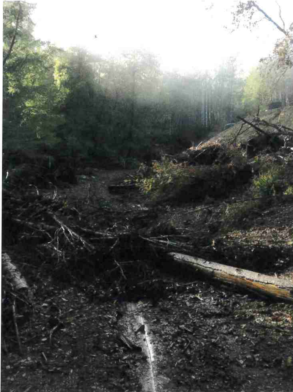
Photo 2: Degraded road requiring road work (Map Point "Degraded Road").
