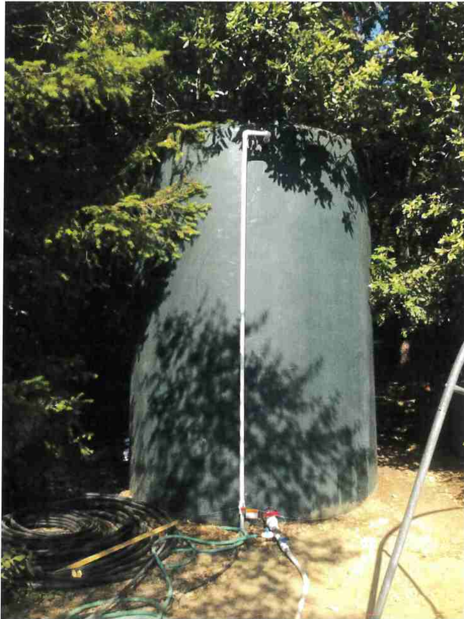
Photo 10: One 5,000 gallon poly storage tank. Photo date 9-8-16
