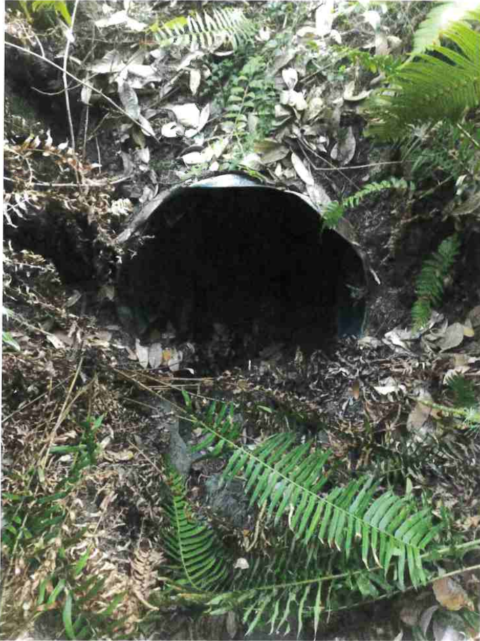
Photo 6: Crossing #1 inlet. Photo date 9-8-16
