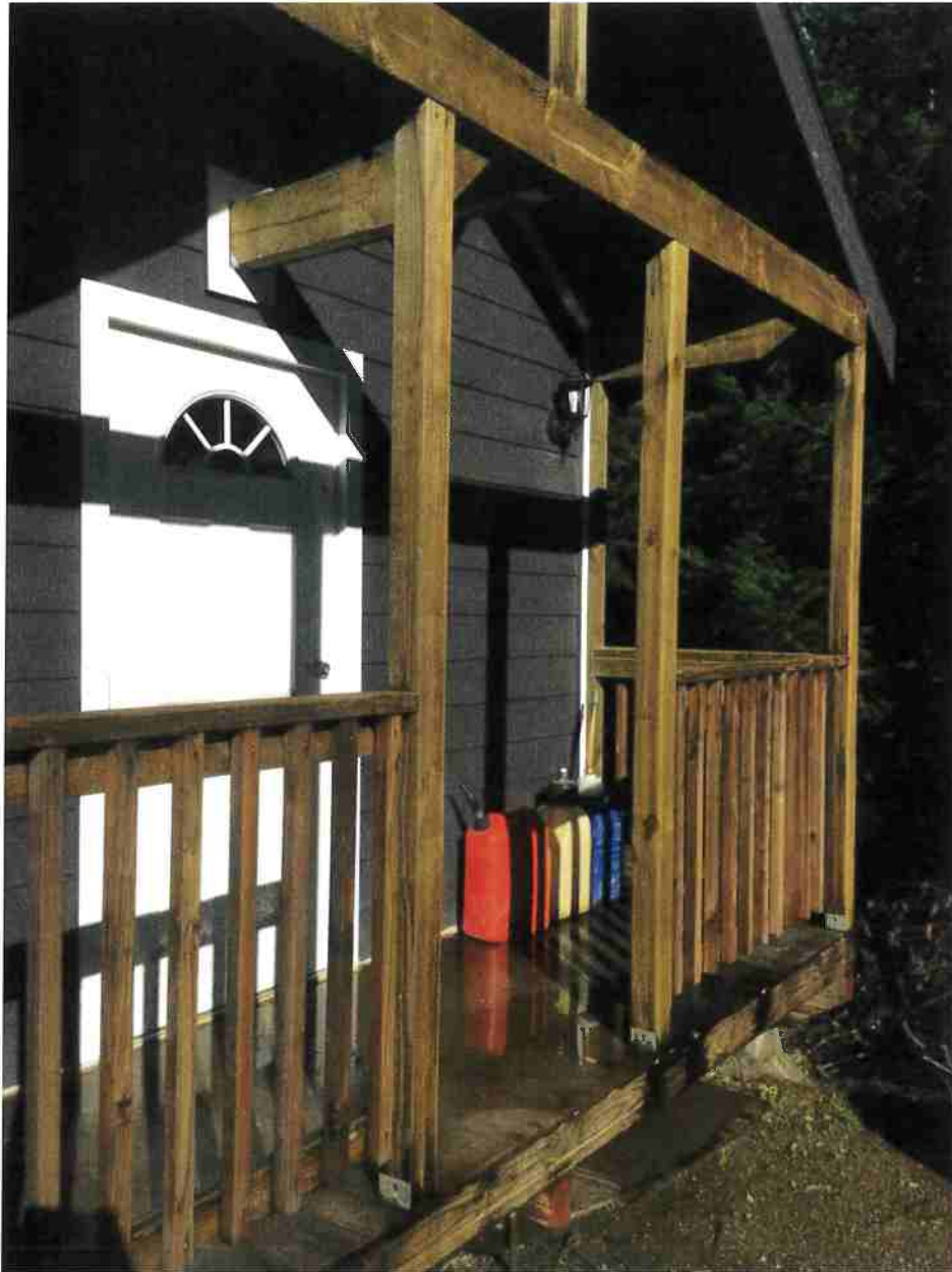
Photo 15: Petroleum storage. Photo date 1-24-17
