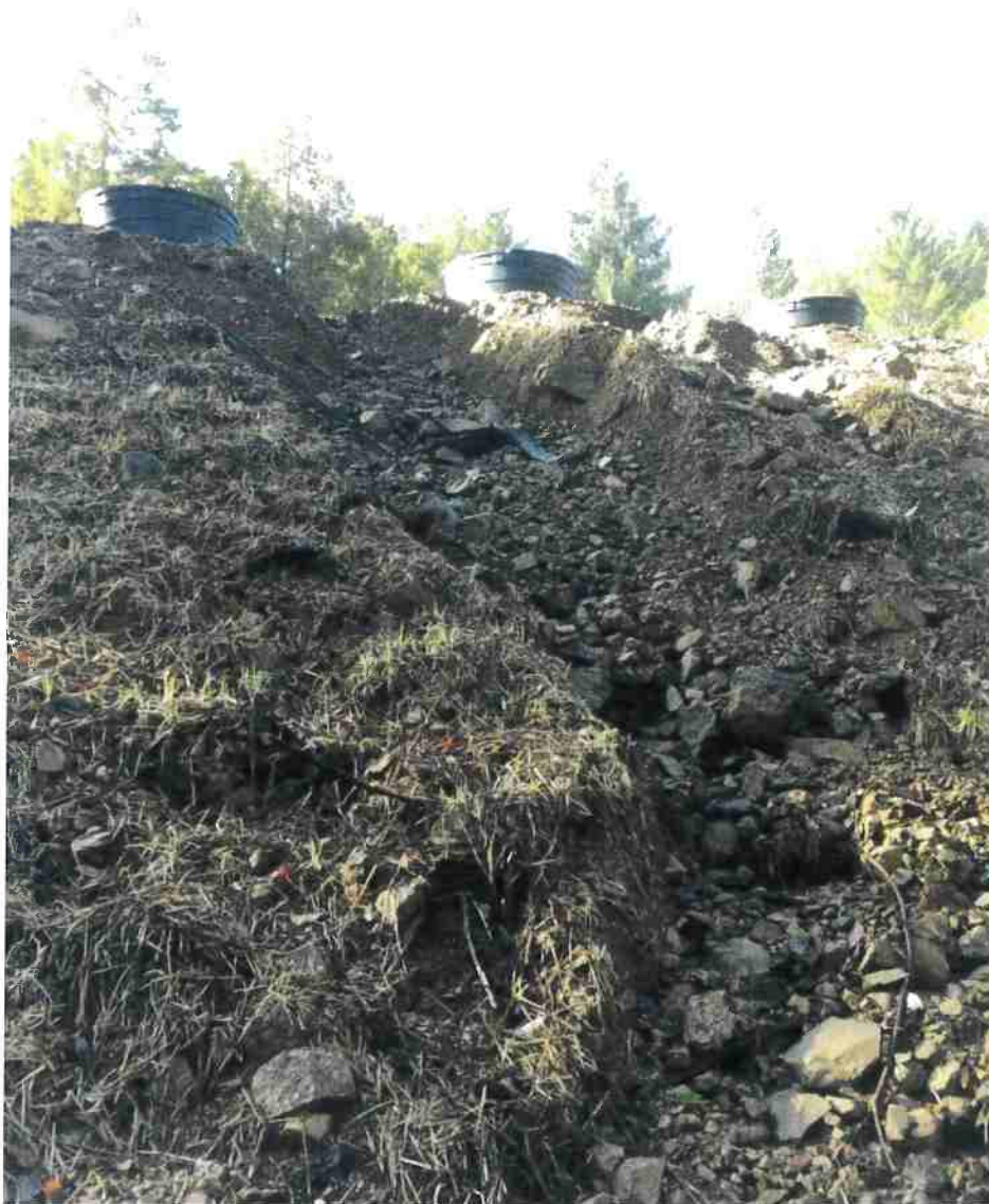
Photo 4: Erosion of fill slope of outdoor cultivation pad (Map Point B). Photo date 1-24-17
