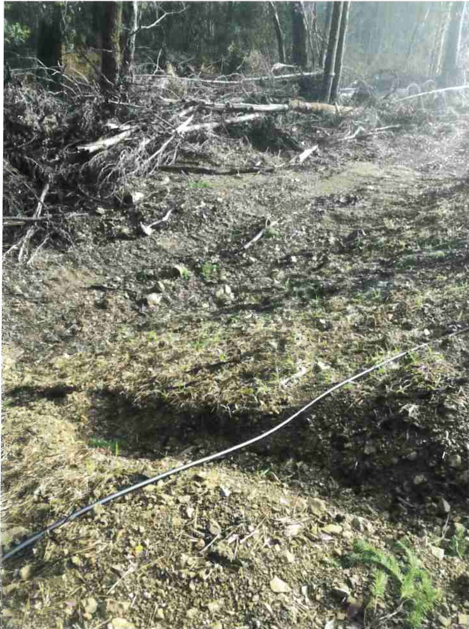
Photo 8: Spoils. Photo date 1-24-17
