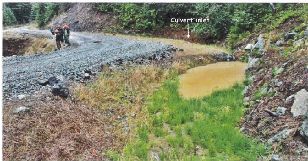
FIGURE 238. Traffic and surface runoff from graveled roads often produces surface erosion, turbid runoff and fine sediment transport that can be delivered to streams. Where ditches can't be eliminated, sediment traps and roadside settling basins can be installed to capture and remove most of the eroded sediment. This settling basin has been constructed along the inside ditch just before a stream crossing culvert inlet (see arrow). Eroded sediment from the road and ditch are deposited in the basin before flow is released to the stream. Fine sediments have filled about 1/3 of this basin and vegetation is now growing. Sediment basins require periodic maintenance to maintain their storage capacity.
