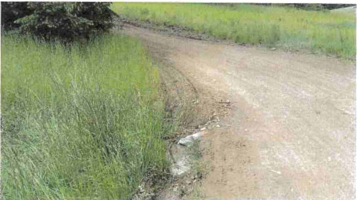
Stream Crossing 1: Class III watercourse consisting of an 18-inch diameter steel culvert, twenty feet in length. This culvert is slightly undersized for the 100-year storm, too short, and filled with sediment because it was installed with a lower gradient than the natural stream channel. Install a 24-inch diameter culvert with a minimum 30-foot length set slightly steeper in grade per the attached specifications.
