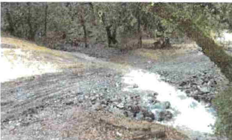
FIGURE 121E. Two weeks after this armored fill was constructed, a spring flow event occurred and the structure maintained its function and integrity. The road approaches had not yet been compacted or surfaced with road rock.
