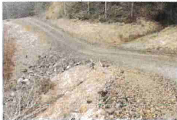
FIGURE 129. This armored fill crossing of a steep, ephemeral stream was constructed to provide a low maintenance crossing. The crossing has been deeply dipped to reduce the volume of road fill and to eliminate the potential for stream diversion. The fill slope has been heavily armored through the area of the crossing to contain sand flows and prevent downcutting. Armored fill cannot be used as load-bearing surfaces. LANDSCAPE FOR FORD, RANCH AND SLURRY, ROAD
