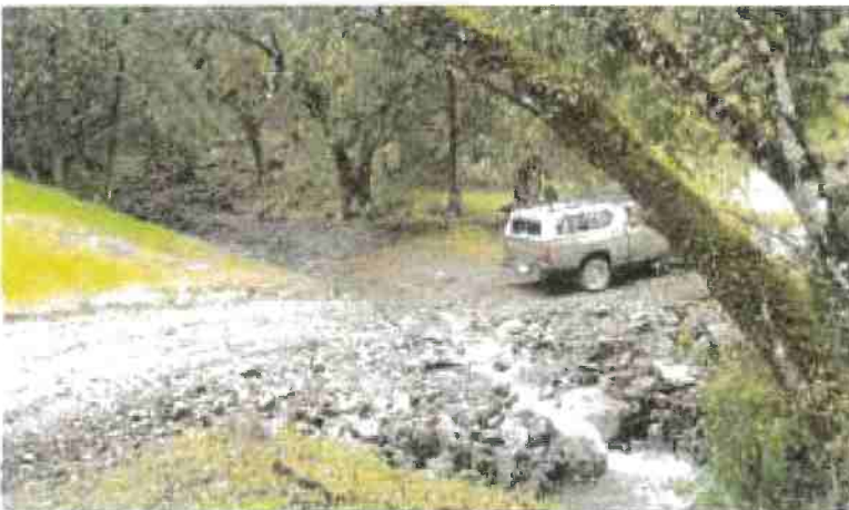
FIGURE 121F. The same armored fill as it appeared after the first winter flood flow. No maintenance was required to reopen the road. It is also clear that no stream diversion is possible at this stream crossing site and the volume of fill within the crossing has been reduced to the minimum amount needed to maintain a relatively smooth driving surface on this low volume road.
