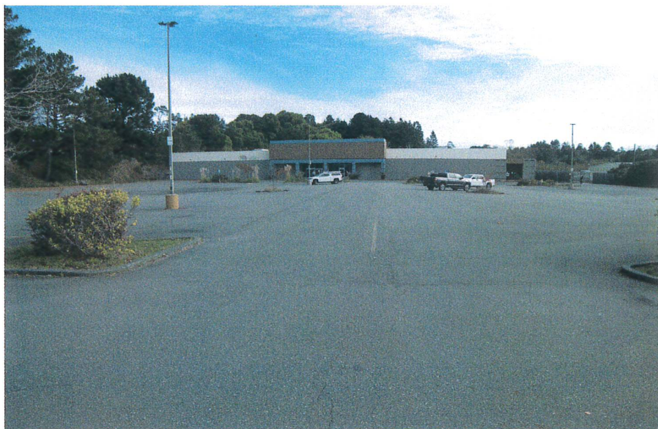
Looking easterly from previous picture over access driveway with paved off-street parking to the right and to the left. Building is in background.
