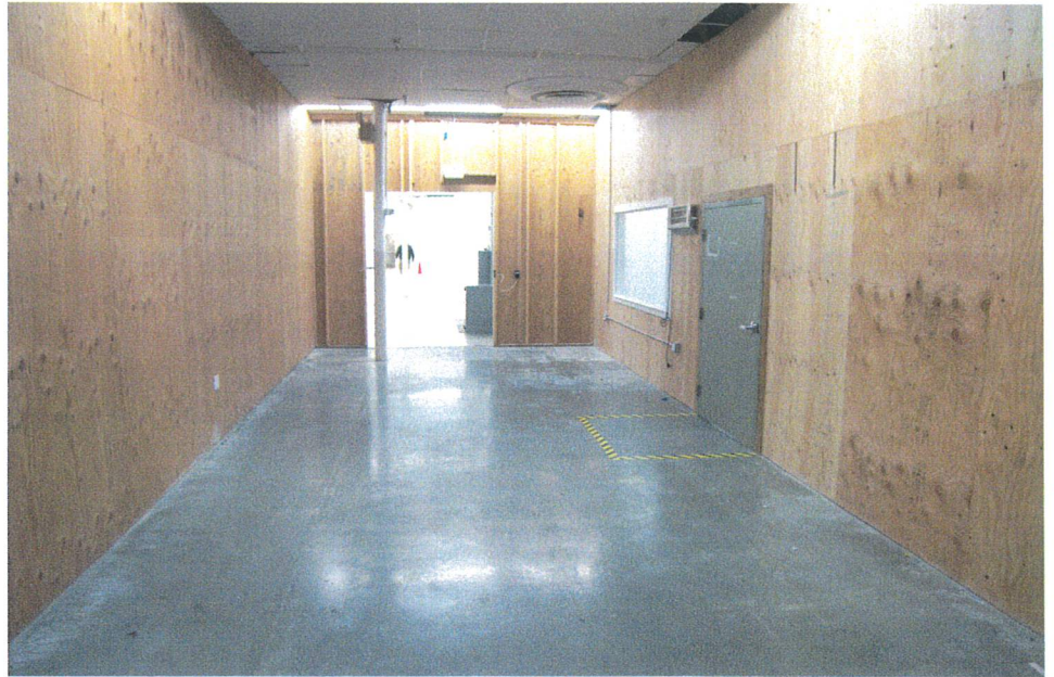
Looking easterly over interior hallway with two adjoining specialty rooms straight ahead and to the right.
