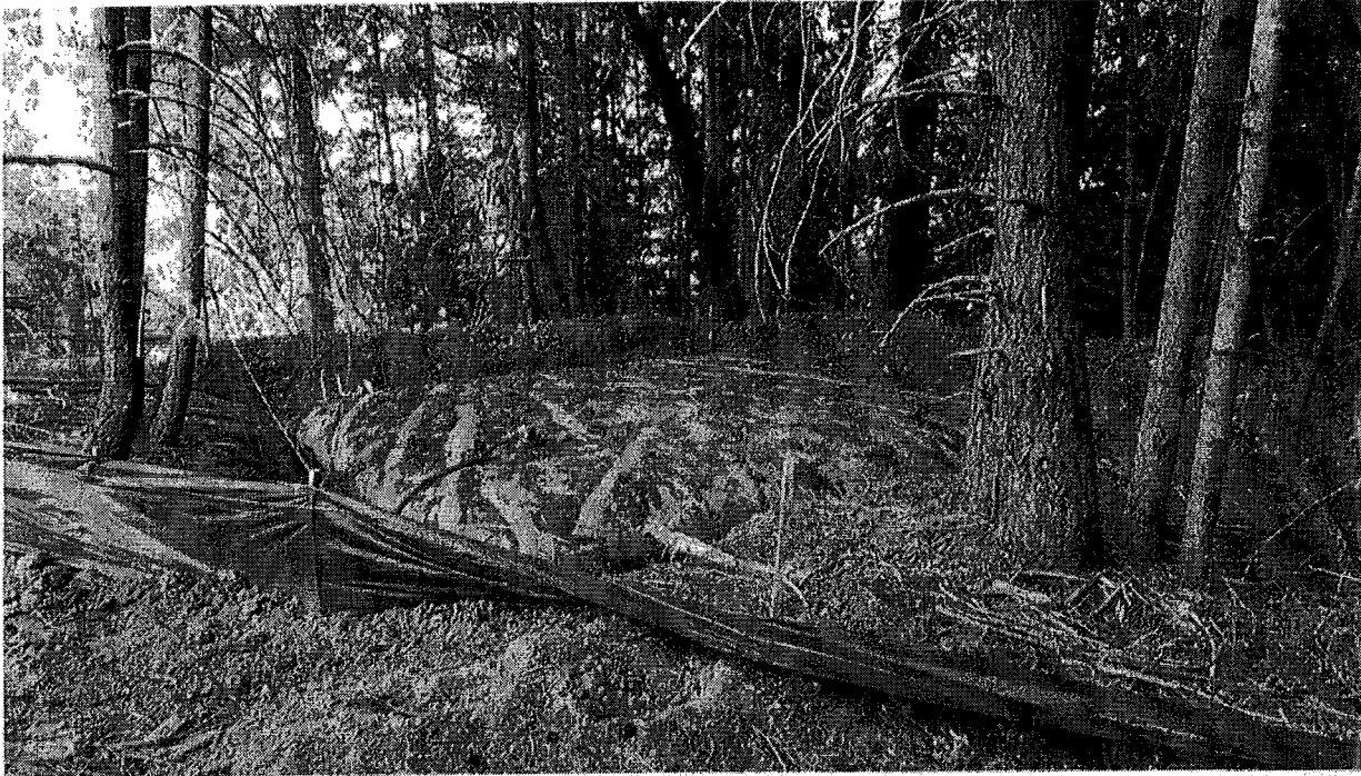
This is an example of a containment pit which will assist in mitigating the impacts if this storage bladder failed.
