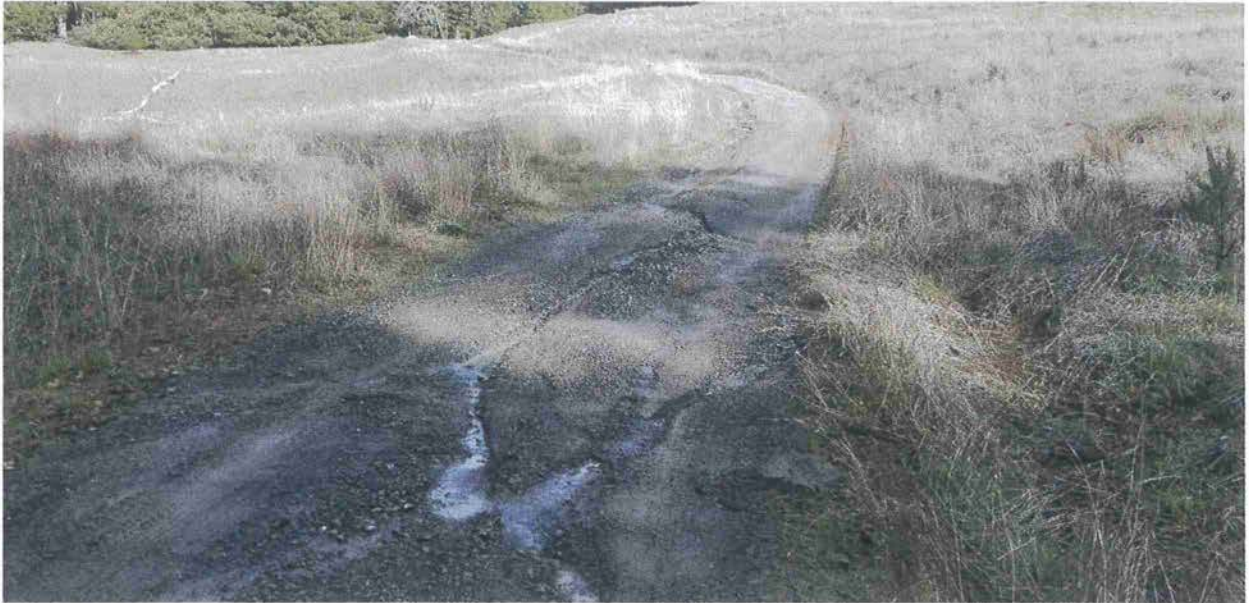
Picture 16: Crossing #2 from the southern approach. Photo date 1-21-2019.
