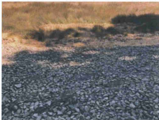
Picture 11 & 12: Existing Rock Ford at Crossing #1 at the head of a Class III watercourse. Photos date 8-13-2018.
