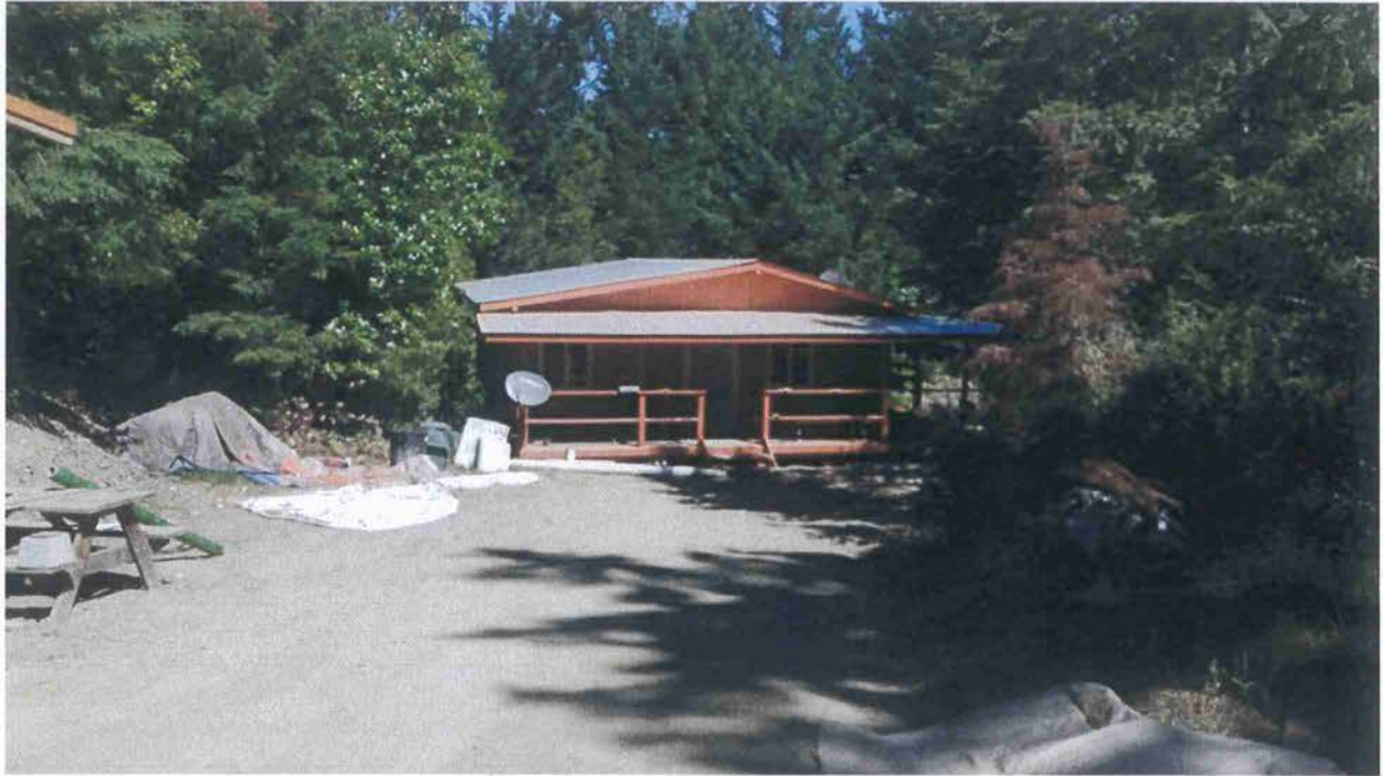
Picture 1: The residence is a place of domestic water use. Photo date 7-06-2017.
