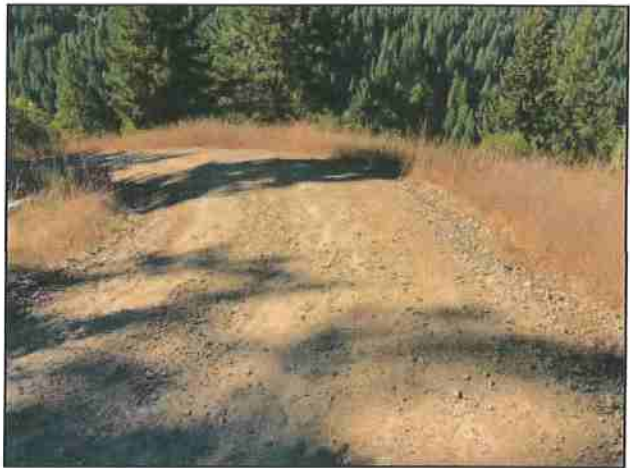
Photo # 769 Private Access Rd @ Curve w/ Turn-out Looking SE
