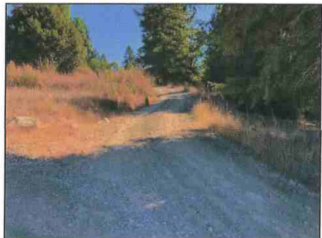
Photo #771 Private Access Rd @ Curve w/ Turn-out Looking SE
