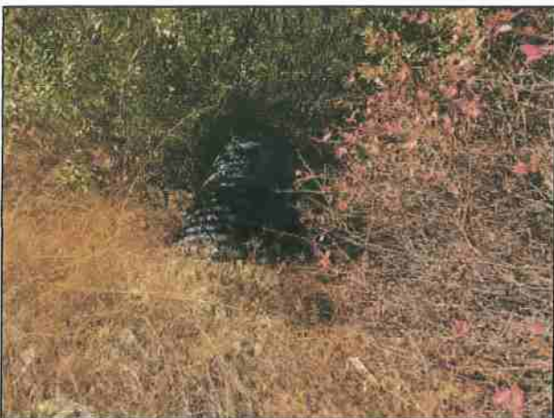
Photo #153 Mad River Medicinals Private Access Rd Looking @ 24" Culvert Out
