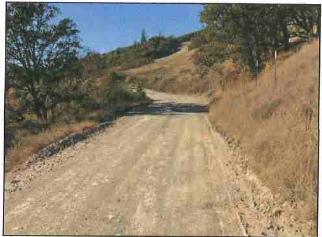
Photo #34 River Rd Looking NW @ Curve w/ Pullout
