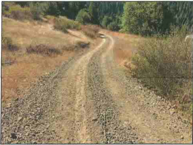
Photo #149 Mad River Medicinals Private Access Rd Looking SW @ Curve w/ Turnout
