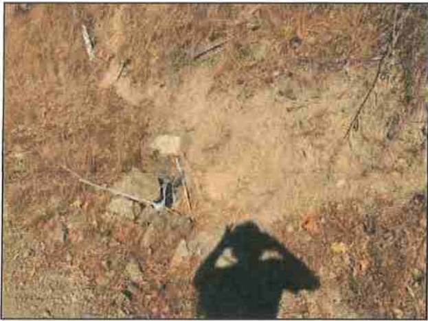
Photo #198 Mad River Medicinals Private Access Rd Looking @ 18" Culvert In
