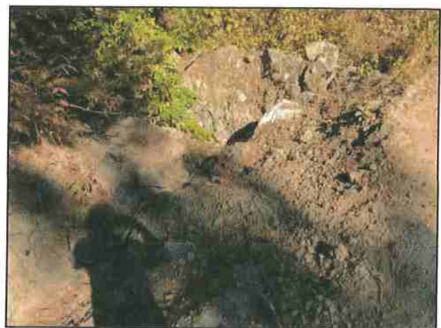
Photo #126 River Rd Looking @ 36" Culvert In
