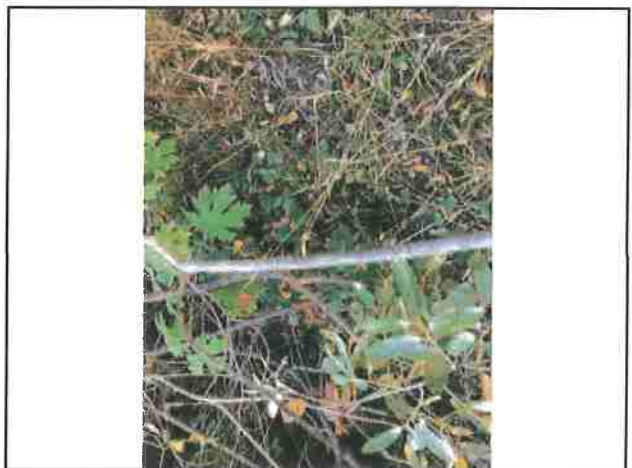
Photo #204 River Rd Looking @ 12" Culvert Out
