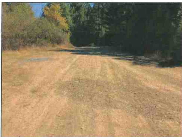
Photo #197 River Rd Looking East @ Curve w/ Turnout
