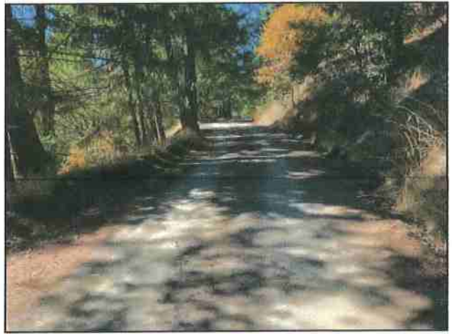
Photo #134 River Rd Looking West @ Curve w/ Turnout
