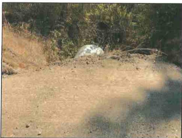
Photo #125 River Rd Looking @ 36" Culvert Out
