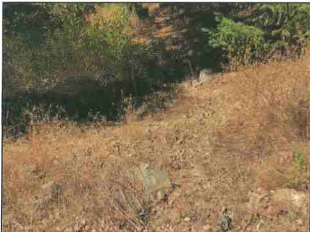
Photo #740 Private Access Rd Looking @ 12" Culvert Out
