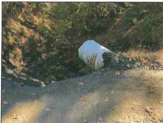
Photo #89 River Rd Looking @ 24" Culvert Out
