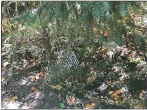
Photo #153 River Rd Looking @ 36" Culvert Out
