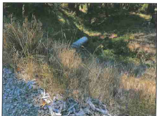
Photo #753 Private Access Rd Looking @ 18" Culvert Out
