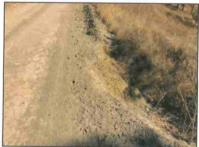
Photo #30 River Rd Looking SE @ Erosion
