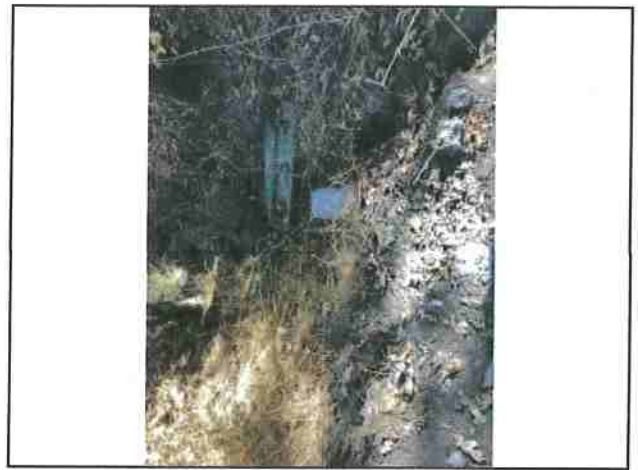
Photo #68 River Rd Looking @ 6" Culvert In
