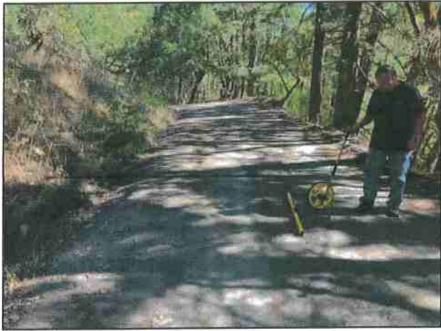
Photo #133 River Rd Looking East @ Curve w/ Turnout
