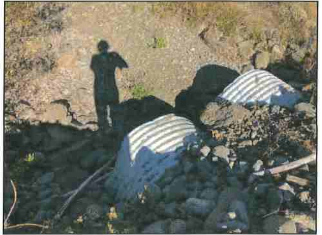
Photo #16 River Rd Looking @ Dual 36" Culverts Out
