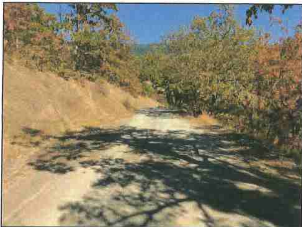
Photo #47 River Rd Looking East @ Turnout
