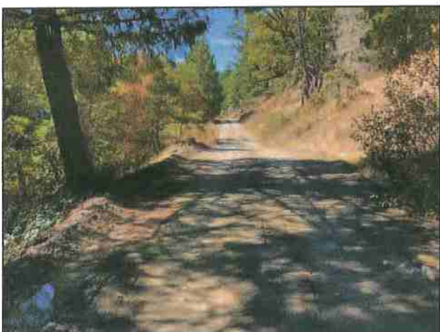
Photo #137 River Rd @ Curve w/ Turnout Looking West
