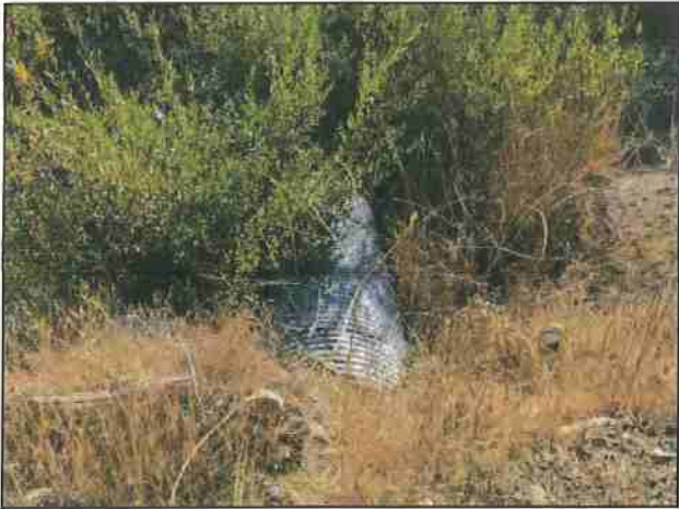
Photo #15 River Rd Looking @ 36" Culvert In
