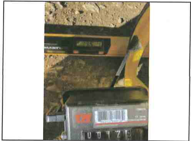
Photo #52 River Rd Slope 17.5% Width 12.8'
