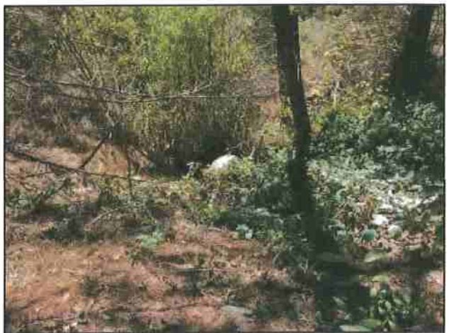
Photo #138 River Rd Looking @ 36" Culvert Out
