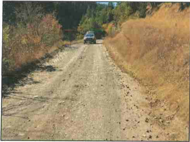
Photo #79 River Rd Looking West@ Curve w/ Turnout
