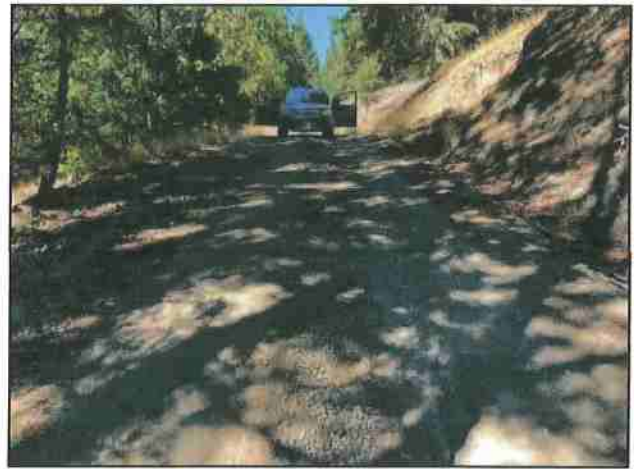
Photo #743 Private Access Rd @ Turnout Looking NW
