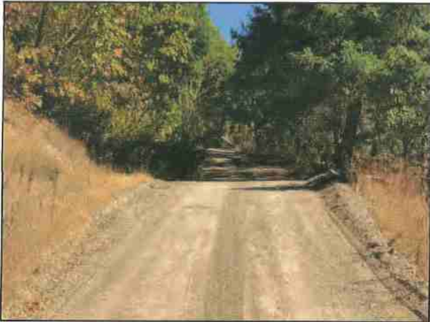
Photo #141 River Rd Looking East @ Curve w/ Turnout
