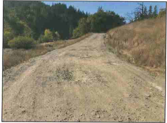
Photo #8 River Rd Looking SW @ Curve w/ Turn-out
