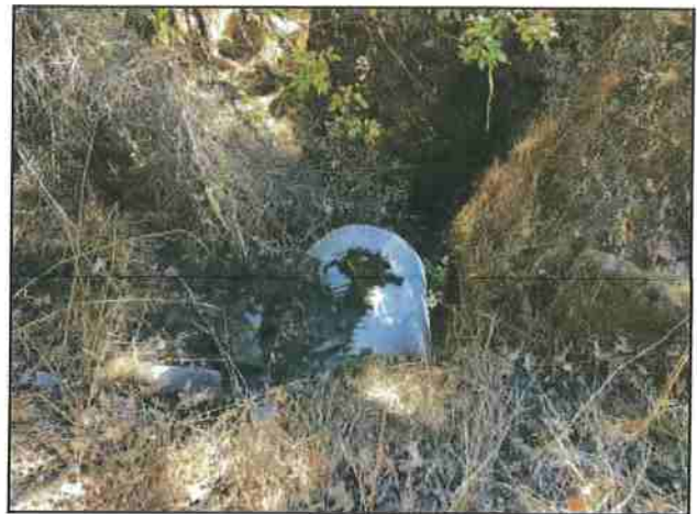
Photo #62 River Rd Looking @ 36" Culvert Out (Dual?)
