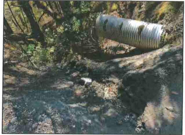
Photo #110 River Rd Looking @ 36" Culvert Out
