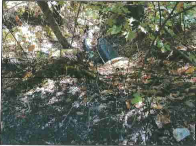
Photo #103 River Rd Looking @ 36" Culvert Out
