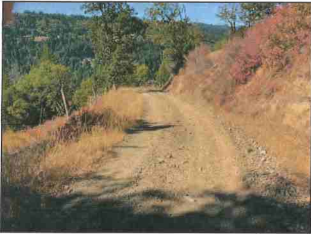
Photo #206 Mad River Medicinals Private Access Rd @ Turnout Looking SW @ Curve
