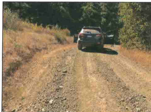
Photo #209 Mad River Medicinals Private Access Rd @ Turnout Looking SW @ Curve
