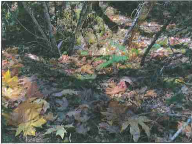
Photo #165 River Rd Looking @ 24" Culvert Out
