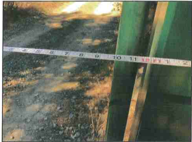
Photo #731A Looking @ Gate in Photo 731 Width 12'
