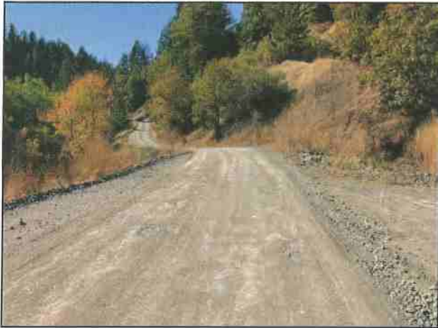
Photo #87 River Rd @ Turnout Looking West Towards Curve
