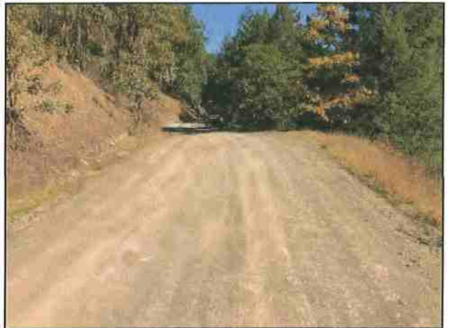
Photo #120 River Rd Looking East @ Curve w/ Turnout
