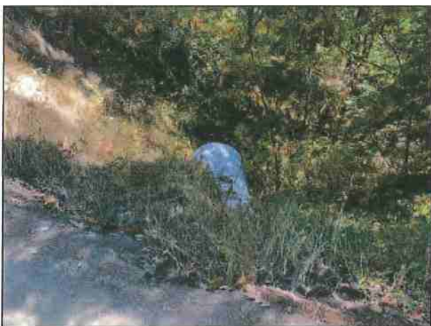
Photo #173 River Rd Looking @ 36" Culvert Out, Inlet Not Found
