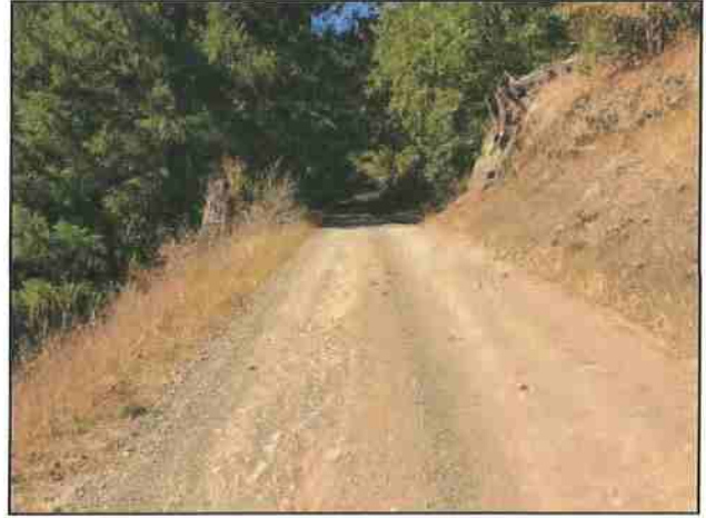
Photo #160 River Rd Looking West
