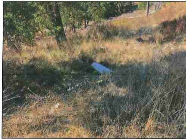
Photo #205 Mad River Medicinals Private Access Rd Looking @ 18" Culvert Out
