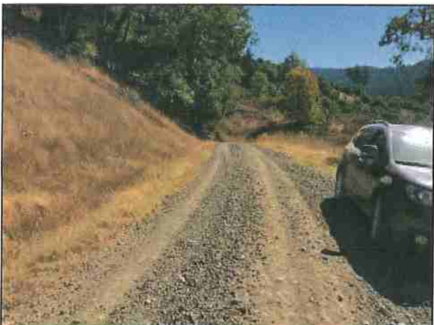
Photo #159 Mad River Medicinals Private Access Rd @ Turnout Location Looking SW
