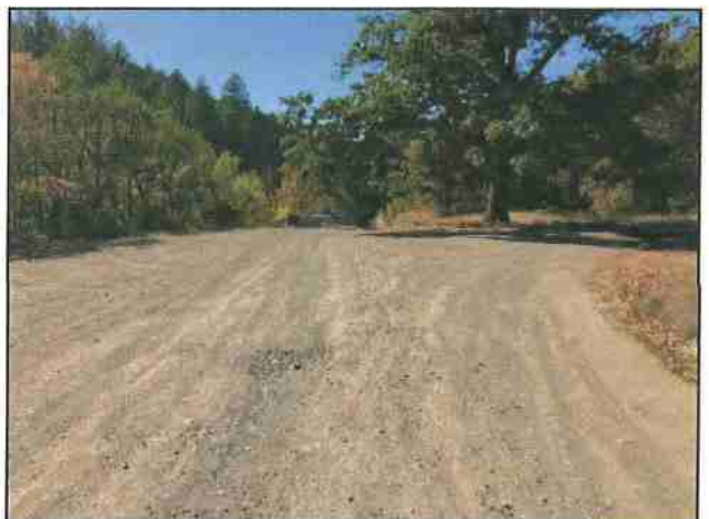
Photo #78 River Rd Looking West @ Turnaround Area
