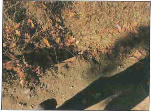
Photo #50 River Rd 12" Culvert In
