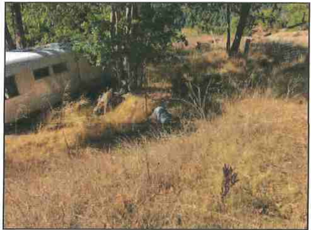
Photo # 199 Mad River Medicinals Private Access Rd Looking @ 18" Culvert Out
