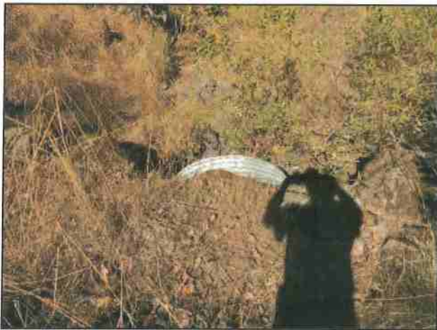
Photo #63 River Rd Looking @ 36" Culvert Out (Dual?)
