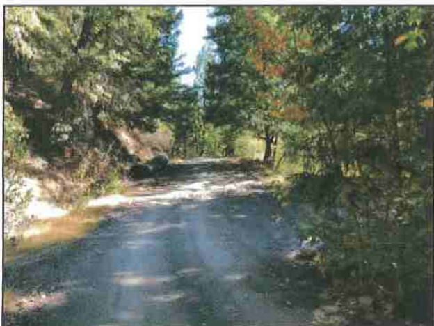
Photo #155 River Rd Looking SE @ Curve w/ Turnout & Old Culvert
