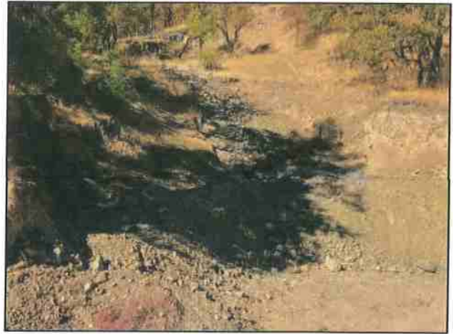
Photo #56 River Rd Looking @ Slide
