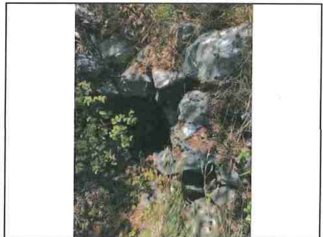
Photo #741 Private Access Rd Looking @ 12" Culvert In
