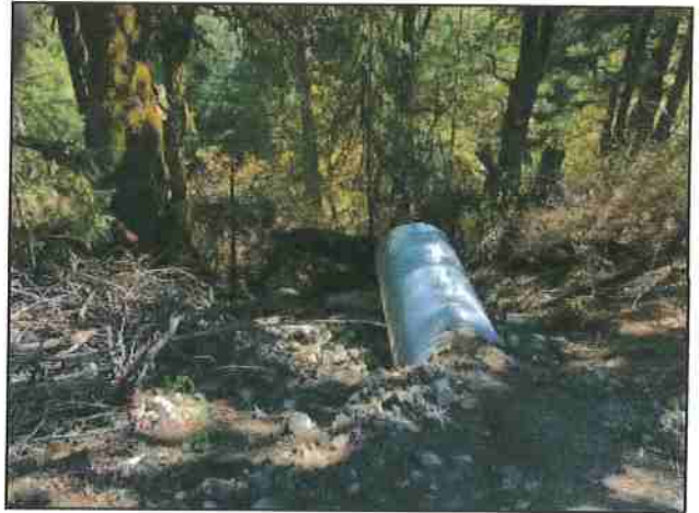
Photo #178 River Rd Looking @ 36" Culvert Out
