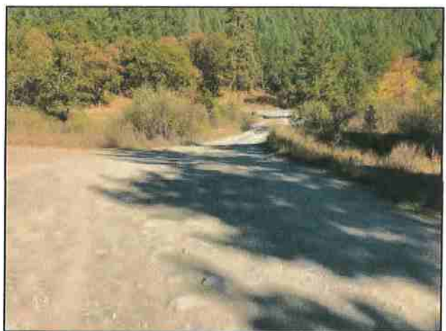
Photo #6 River Rd Looking NE @ Curve w/ Turn-out
