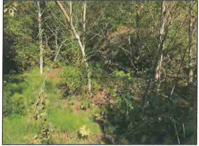
Photo #152 River Rd Looking @ 24" Culvert In
