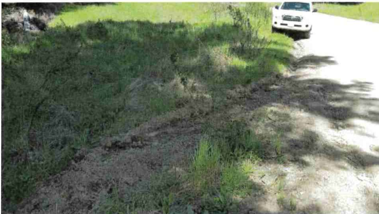
Road Point 9: The lead out ditch is too shallow to effectively capture road surface runoff and contain it along the edge of the road. Re-establish the leadout ditch so that is dug deeper into the road's surface and install three wattle check dams in the ditch and at the leadout ditches outflow above the watercourse to capture road surface runoff sediment.
