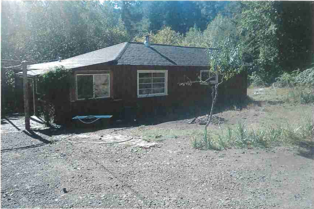
Photo 1: Project area looking south at the existing caretaker unit to be demolished. The new unit will be constructed partially within the footprint of the existing unit and partially within the area shown in this photo in front of the existing unit. Photo taken September 29, 2021.
