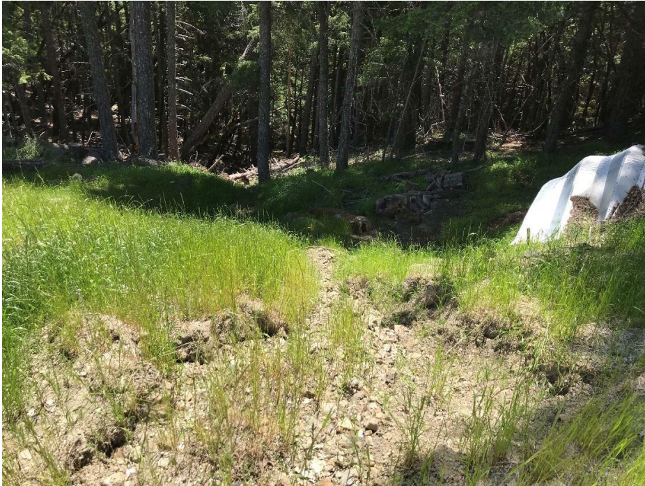
Photo 3. Observation Point 2(a), incised channel going down unstable fillslope toward Class III watercourse (in tree line) from concentration point on graded flat.
