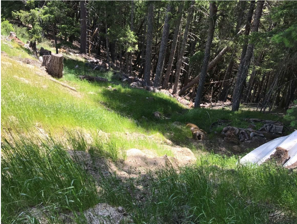
Photo 7. Another view looking down gullied fillslope at Observation Point 2(a), also note cut trees and hazard reduction debris.
