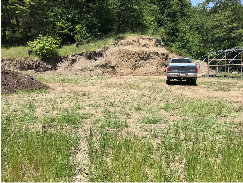
Photo 6. Observation Point 2(b), concaved area on graded flat where water concentrates before heading toward Observation Point 2(a) – fillslope and incises down to Class III watercourse.
