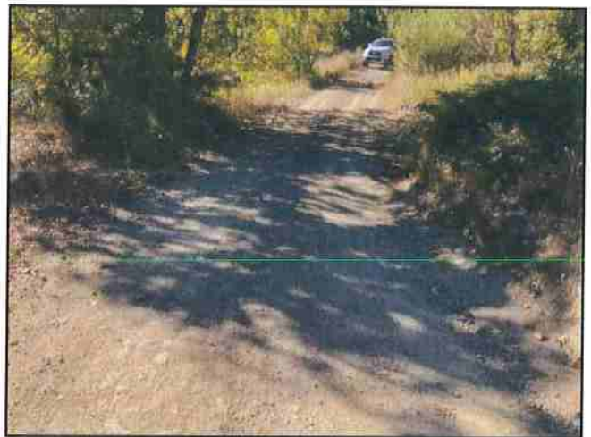
Photo #428 River Rd @ Curve w/ Turnout Looking NW
