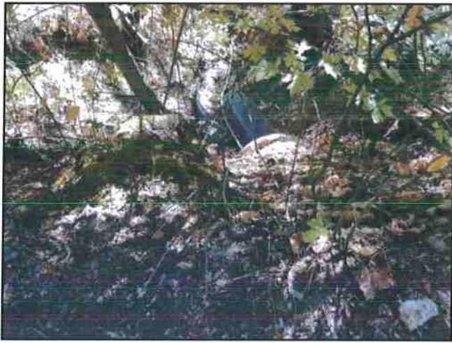
Photo #103 River Rd Looking @ 36" Culvert Out
