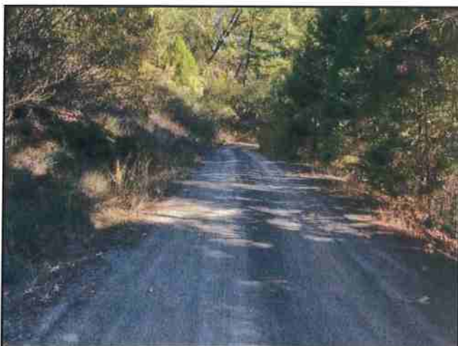
Photo #215 River Rd Looking SE @ Curve w/ Turnout
