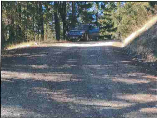
Photo #339 River Rd Looking NW @ Curve w/ Turnout
