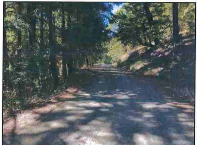
Photo #166 River Rd Looking SE @ Curve w/ Turnout
