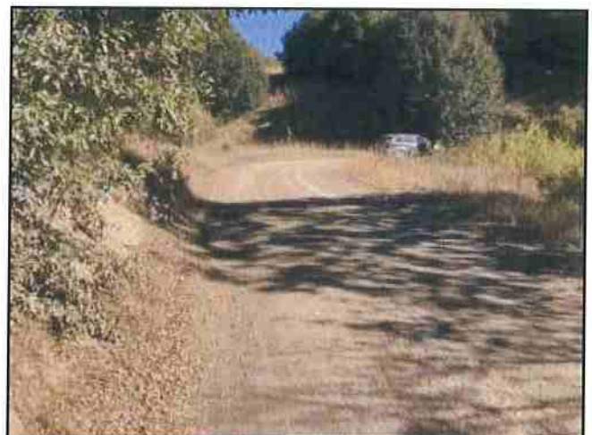
Photo #412 River Rd @ Curve Turnout Looking NE
