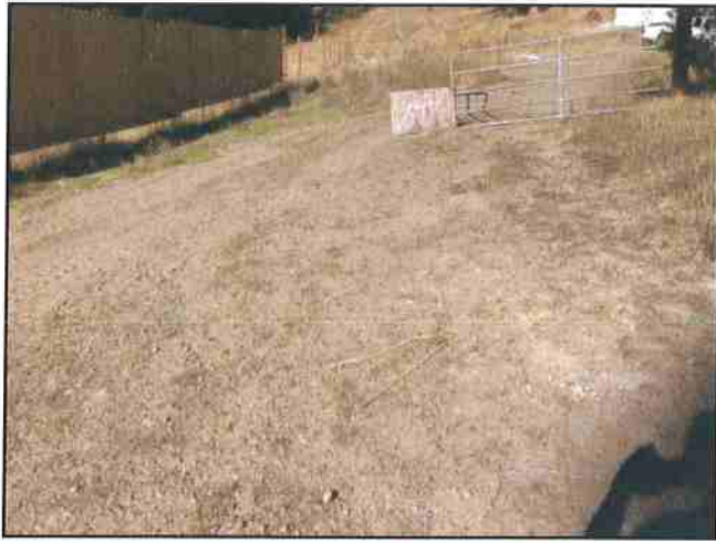
Photo #433 River Rd Looking NE @ Approach
