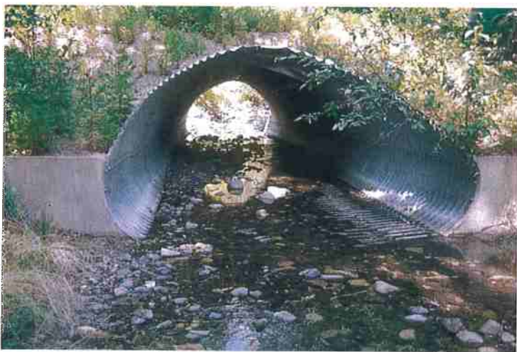
Figure 28. An arched pipe installed on a fish-bearing stream to minimize impacts on fish habitat and migration. Source: Keller and Sherar 2003.
