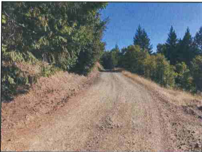
Photo #405 River Rd @ Turnout Location on Curve Looking South
