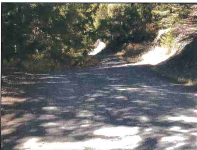
Photo #281 River Rd @ Turnout Location Looking @ Curve
