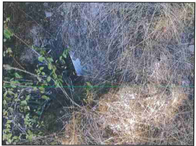
Photo #302 River Rd Looking @ 24" Culvert Out
