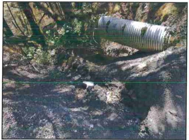
Photo #110 River Rd Looking @ 36" Culvert Out
