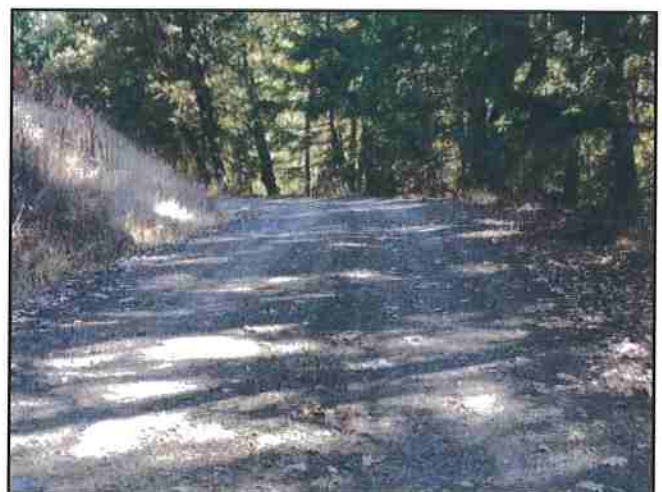
Photo #336 River Rd Looking South @ Curve w/ Turnout
