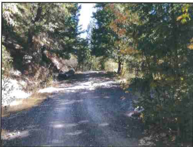
Photo #155 River Rd Looking SE @ Curve w/ Turnout & Old Culvert
