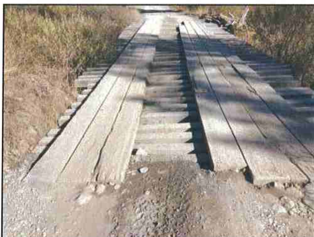
Photo #3 River Rd Looking East @ RR Car Bridge
