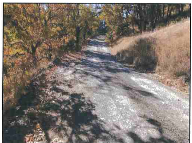
Photo #48 River Rd Looking West @ Turnout
