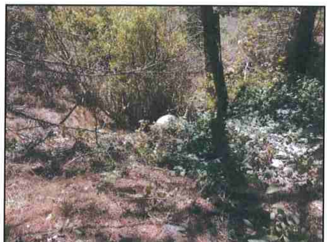
Photo #138 River Rd Looking @ 36" Culvert Out
