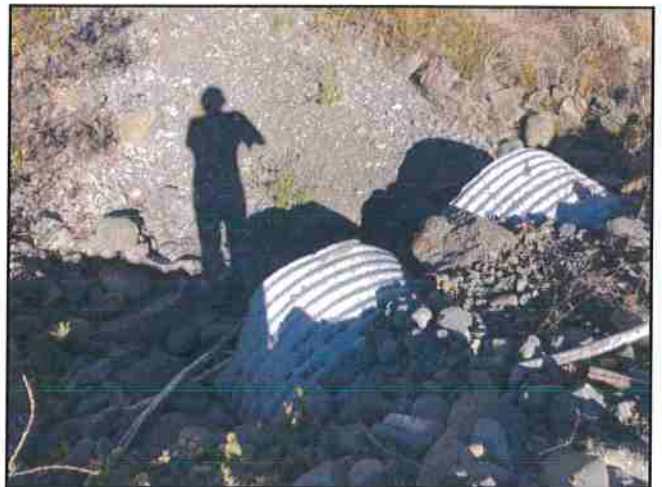
Photo #16 River Rd Looking @ Dual 36" Culverts Out
