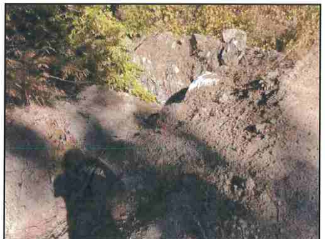
Photo #126 River Rd Looking @ 36" Culvert In
