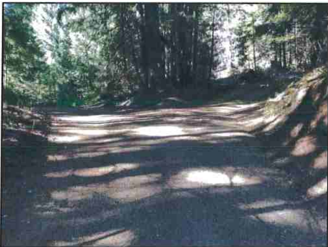
Photo #459 River Rd Looking SW @ Approach
