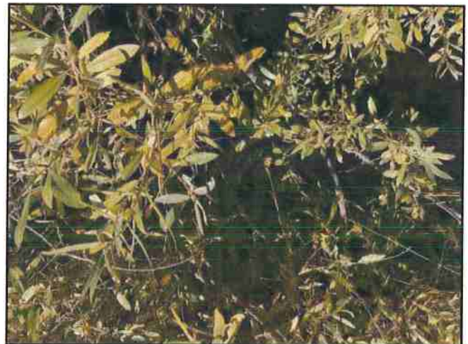
Photo #220 River Rd Looking @ Partially Clogged 24" Culvert In
