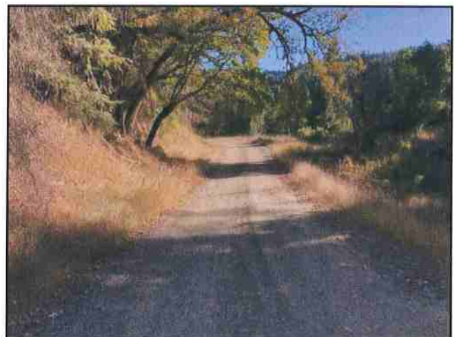
Photo #300 River Rd Looking South @ Curve w/ Turnout
