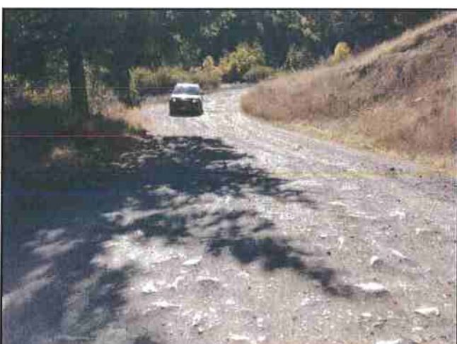
Photo #5 River Rd Looking SW @ Curve w/ Turn-out
