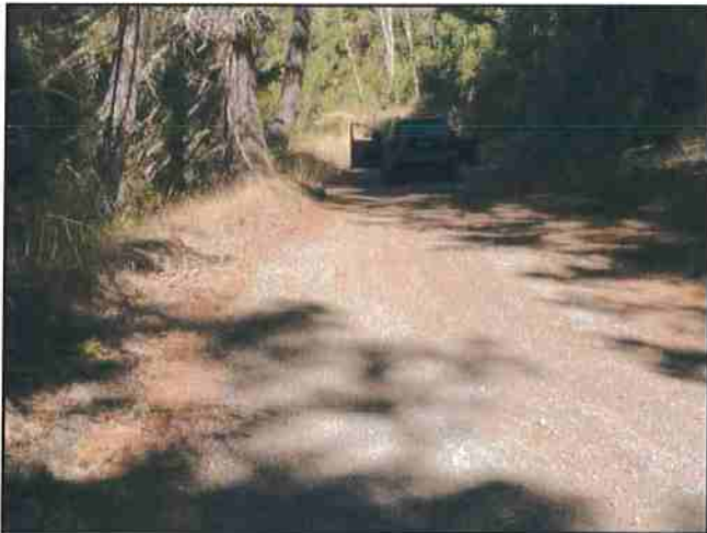
Photo #291 River Road Looking North @ Curve w/ Turnout
