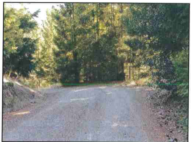
Photo #308 River Rd Looking South @ Curve w/ Turnout
