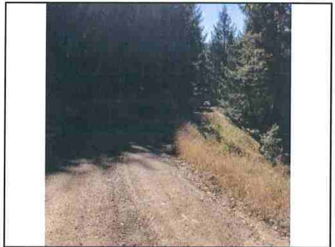
Photo #298 River Rd @ Turnout Location Looking South @ Curve
