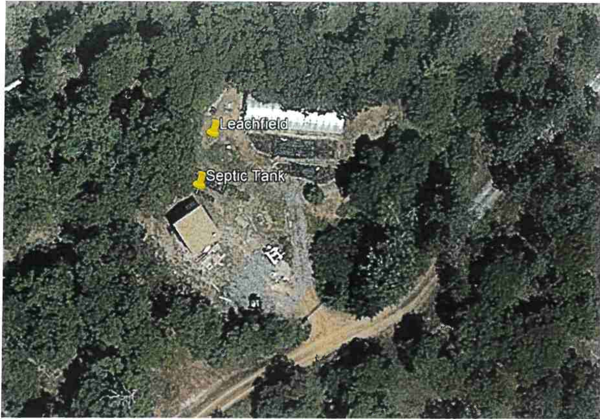
APN: 221-061-036 – approximate location of septic tank and leachfield serving cabin
