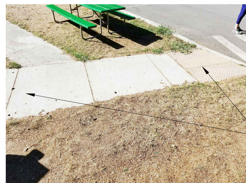
14 WALKWAY AT PICNIC TABLES
