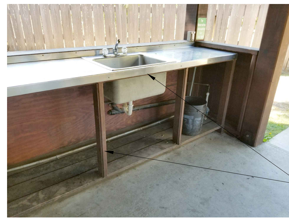
8 SINK/COUNTER AT UPPER PAVILION
