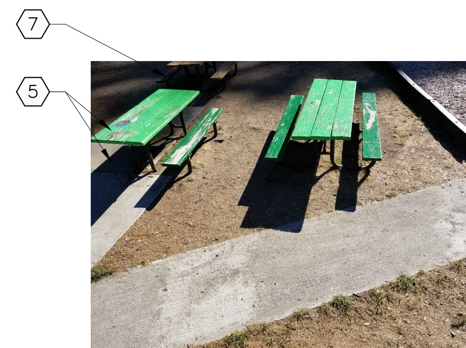
7 PICNIC TABLES AND CONCRETE SLAB AT PLAYGROUND
