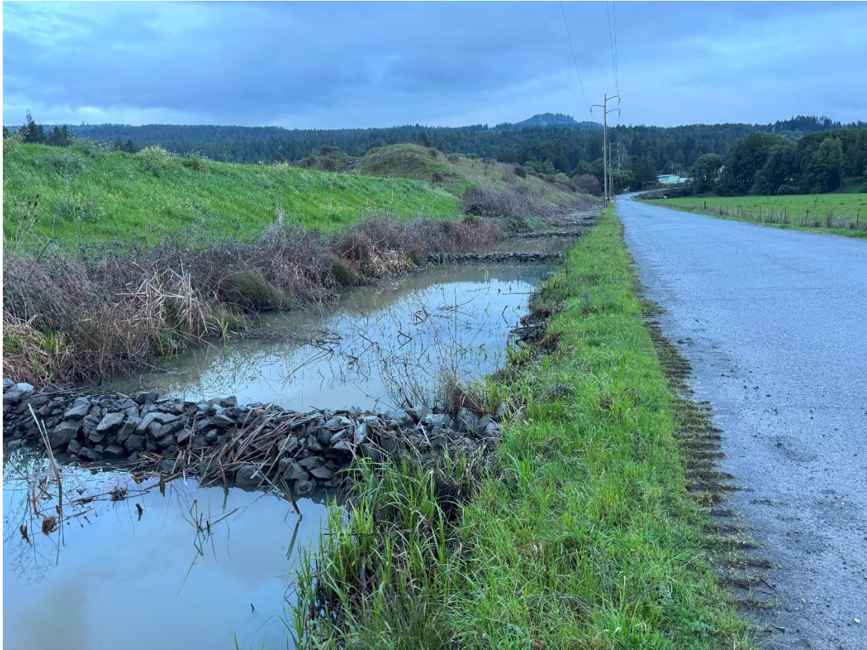
Picture 12 – Looking east at the roadside swale adjacent to the lower yard. These Waters of the State receive runoff from the adjacent stockpile and from the haul roads in the lower yard area. The non-standard rock check dams were installed by the Discharger without obtaining an appropriate permit from the Regional Water Board. Picture taken by Walt Dragaloski.
