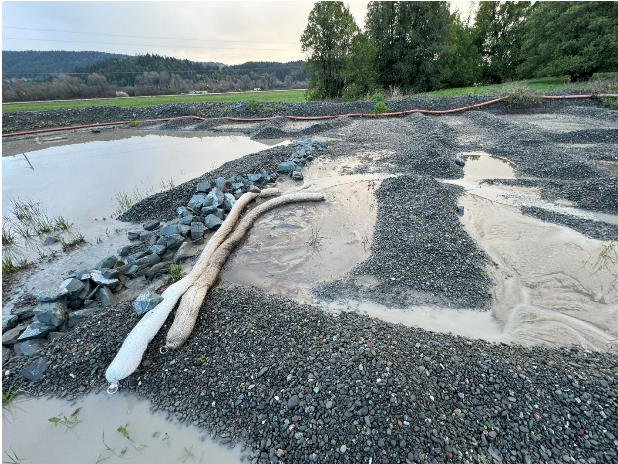
Picture 5 – Looking west at the sediment trap located on the southwest corner of the upper yard. A significant amount of sediment is captured with this non-standard sediment and erosion control BMP. Picture taken by Walt Dragaloski.
