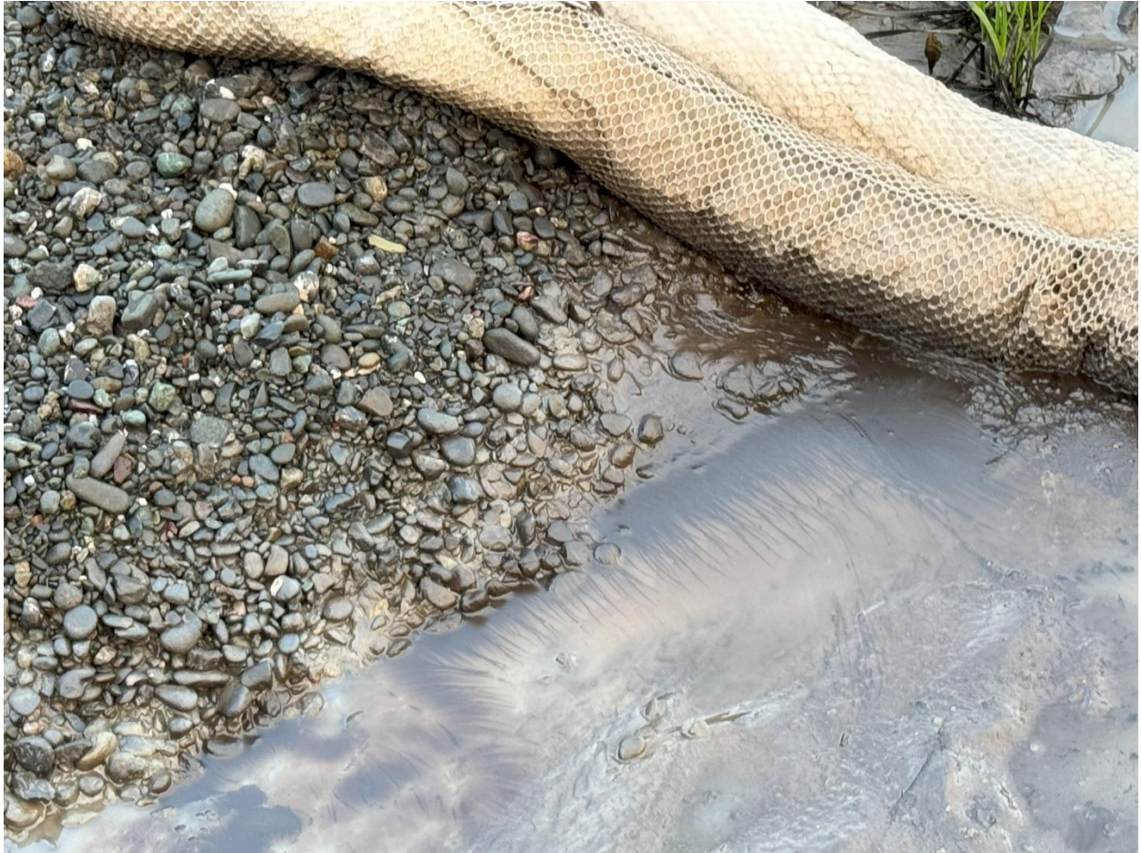
Picture 7 - View of an absorbent sock in the sediment trap. A sheen was observed on the water surface and a black oily residue was observed on the gravel and the absorbent sock within the sediment trap. Picture taken by Walt Dragaloski.
