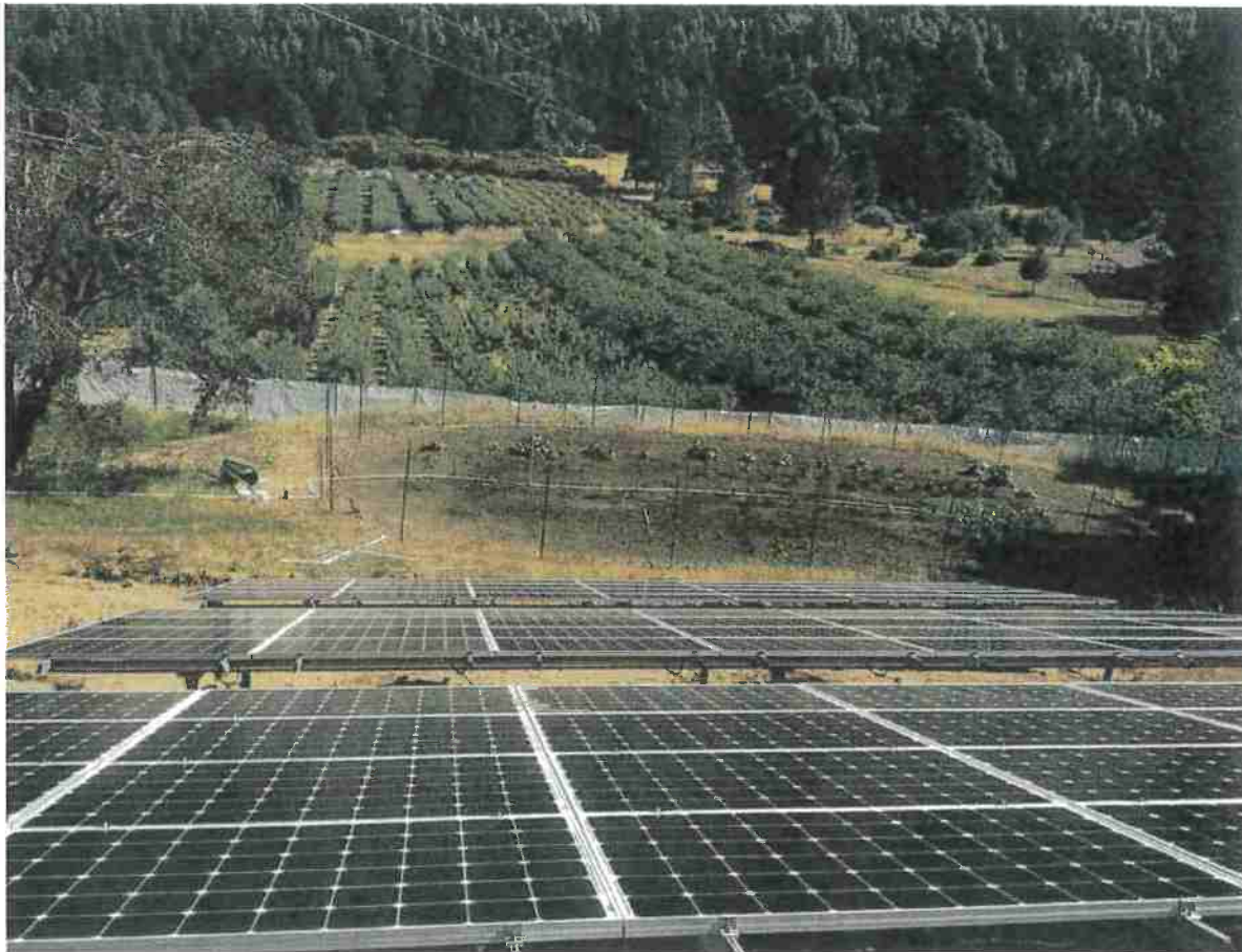
Whitethorn, CA: A 20 kW ground mount grid-tied system powering the home and operations of a local Quince farm.
