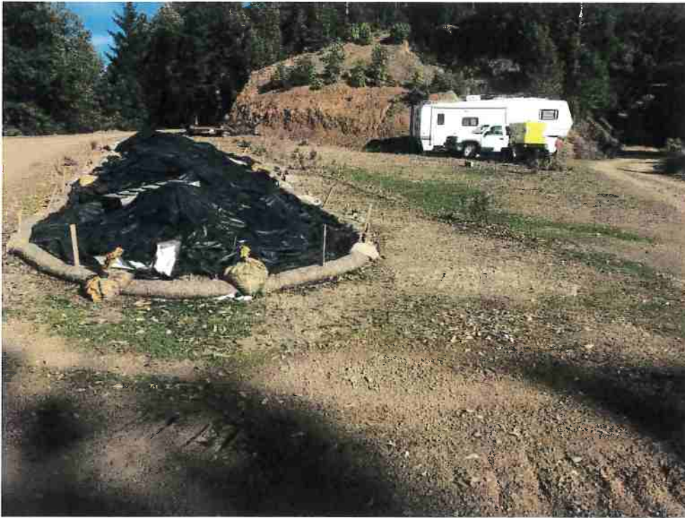
Photo 2. Erosion control measures at Conversion Site 5.
